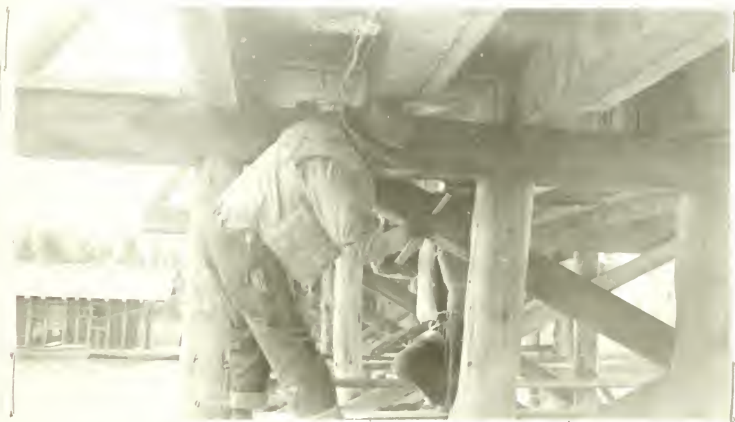
(1935) 202.1 General Maintenance. View of stringer repairs on Fishing Bridge.
