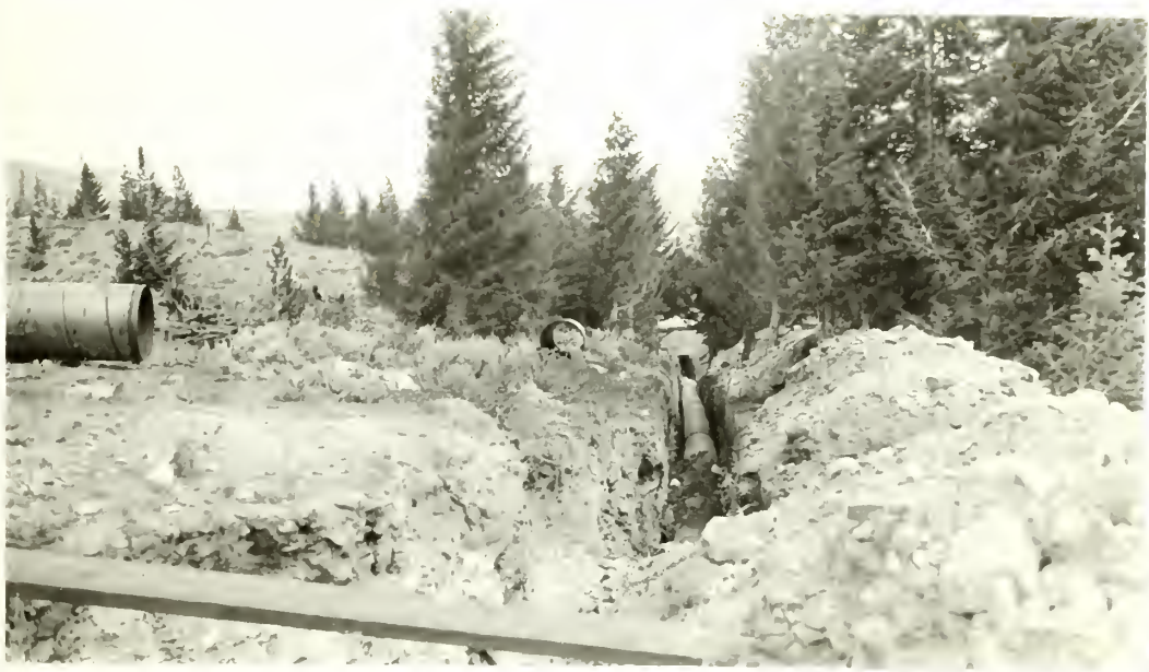
(1935) FP 598 Hydro-electric Plant, Mammoth. View of 30" O.D. pen-stock pipe in place on run around. View from about sta. 30 + 00.
