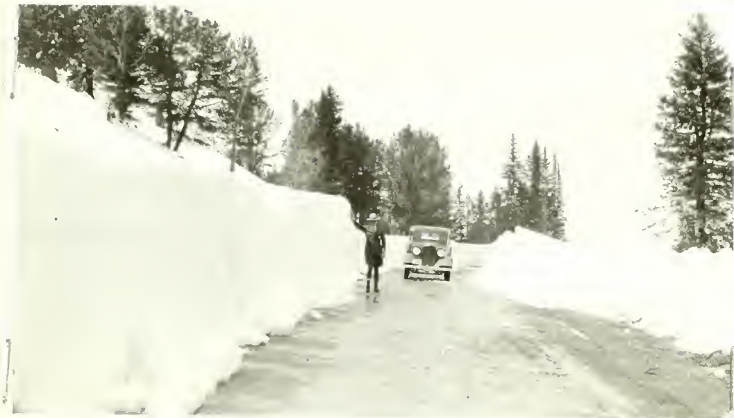
Sylvan Pass a few days after highway had been cleared of snow by Park Service Sno-Go. Note height of drift on upper side of road. This road was opened to travel on May 26, and numerous park visitors enjoyed the unusual experience of driving over snow walled highways.
