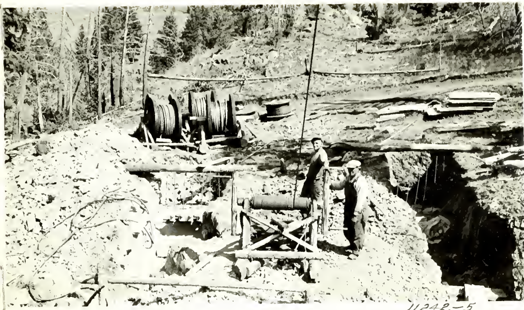
(1935) 509 Elk Creek Suspension Bridge. View of cable reels in position for hanging of cables, highline winch in center, and westerly main cable anchors.
