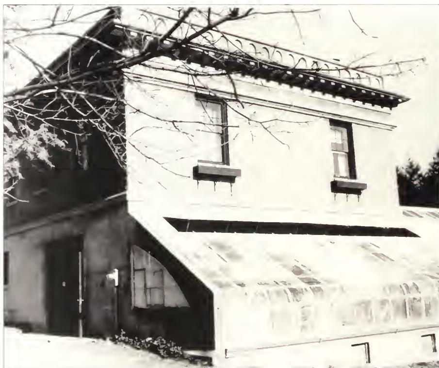
Figure 1.32. A 1970s image looking northeast towards the 1908 concrete gardener's cottage and potting shed, constructed during Thomas Edison's experimentation with concrete (EDIS Archives).
