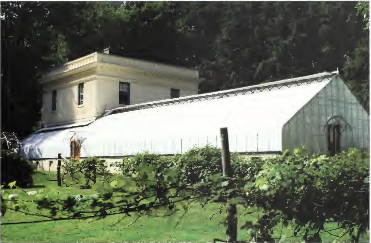
**Figure 2.34: Buildings and Structures.** View looking north towards the gardener's cottage, potting shed, and greenhouse. The gardener's cottage and potting shed, built in c.1908, is one of the earliest examples of monolithic concrete construction developed by Thomas Edison (OCLP, 2009).
