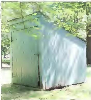
**Figure 2.37: Buildings and Structures.** The hose house, constructed in 1904, is a small-wood-frame structure used to house a fire-hose cart. It is situated within the laundry yard (OCLP, 2009).
