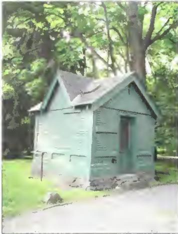
Figure 2.38: Buildings and Structures. Similar in Victorian architectural design and construction as the house, the pump house built between 1882 and 1884, is a small wooden structure with a cross gable roof set on a fieldstone and mortar foundation (OCLP, 2009).
