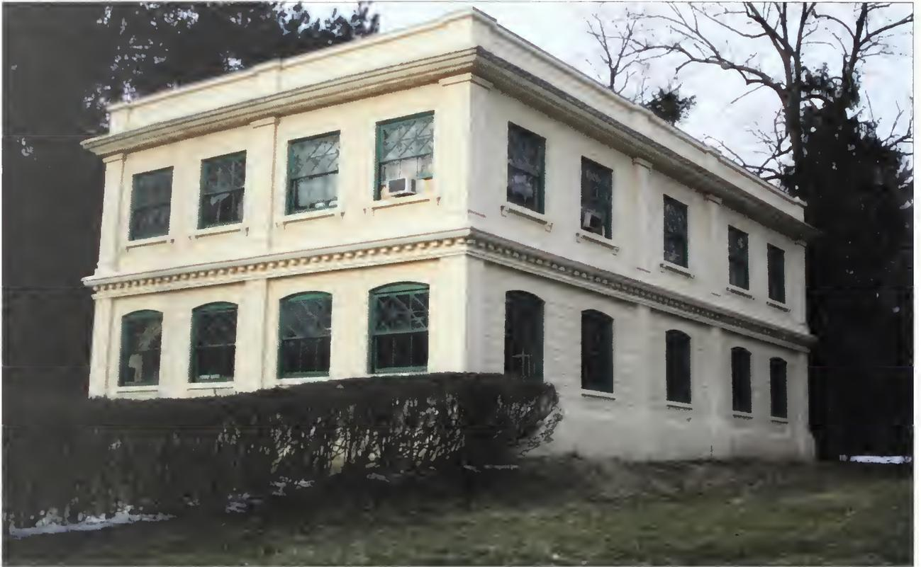
**Figure 2.35: Buildings and Structures.** View looking north towards the garage. It is one of the earliest examples of monolithic concrete construction developed by Thomas Edison. The two-story structure was erected in 1908, east of the house along Honeysuckle Avenue, and in the former location of Pedder's L-shaped chicken house and cow barn (OCLP, 2009).
