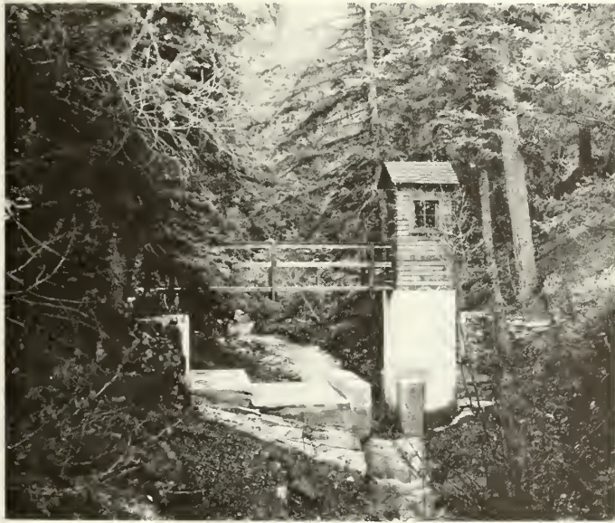
Figure 23.—Combination San Dimas flume and broadcrested weir gaging station near the mouth of Missouri Gulch.
