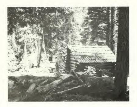
The Squatter's Cabin in Giant Forest was typical of the late nineteenth-century structures built for more comfortable and more frequent occupancy. Considerably more time and thought went into the construction of this generation of shelter. Notching and fitting the logs, splitting the shakes, and laying the chimney masonry took time and considerable effort.
