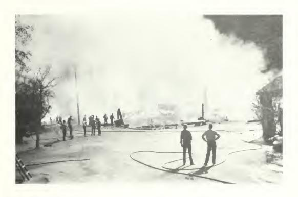
The Ash Mountain fire of November 11, 1939 destroyed several maintenance buildings and could have taken most of the woodframe headquarters development with it. Luckily conditions for spread of fire were minimal on that day. Even so, the hot drafts from the fire blew roof shingles a mile away. As a result of this fire, all new construction in Ash Mountain had to be fireproof.
