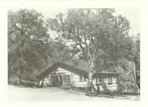
Simple pole-and-shingle buildings such as these housed functions at park headquarters in Ash Mountain. Colonel White's preference for "temporary" (lacking masonry or cement) structures prevailed through the mid-1930s.
