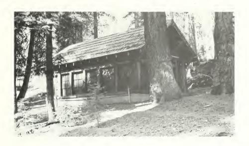
A simple style developed for utilitarian Park Service structures such as this comfort station in Giant Forest. Following the rustic pattern established by the earlier Park Service buildings in Giant Forest, the exposed framing defined the building's edges and structure. The shake infill added the rough texture equivalent to the roughness of the surrounding trees.
