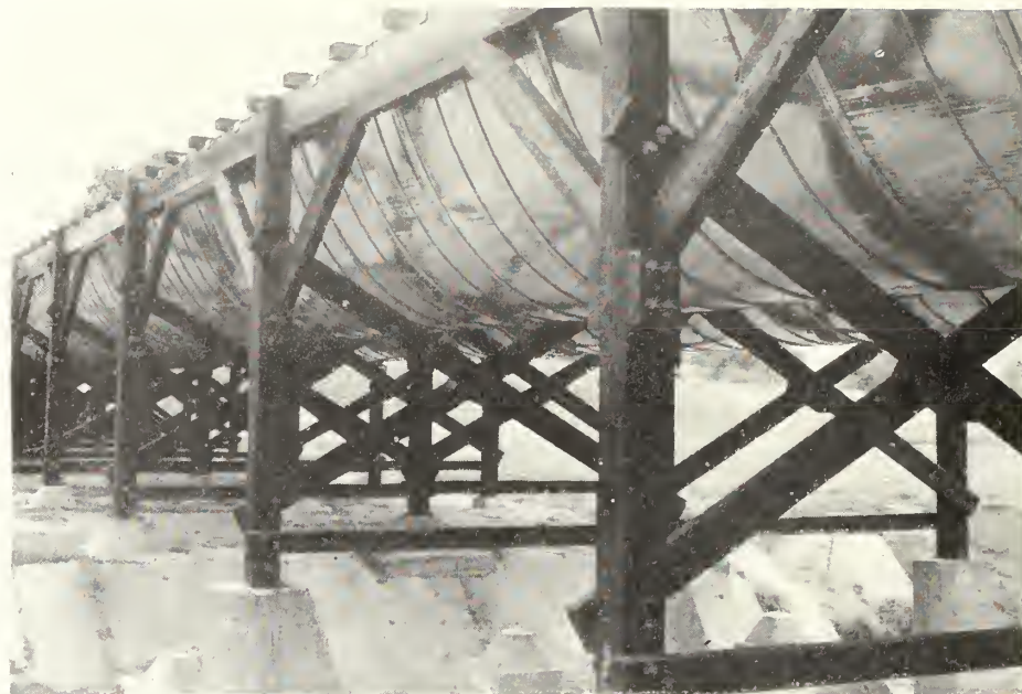
ACCENT ON BETTERMENT typified the rehabilitation and betterment work at the Orland project in California. Above, the rebuilt Highline Flume, complete with new timber supports and concrete footings, plus an expanded capacity. Major features of the rehabilitation program are located on the simplified map at right and above. Drawing by the Bureau's Graphics Section in Washington, D. C.
