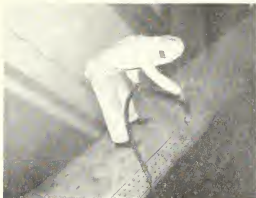
SAND-BLASTING the outlet tube at East Park Dam, above, preparatory to painting on July 19, 1949. DANGEROUS GATE STEM of Stony Gorge Dam, center photo, shows the broken screw threads which made it hazardous to operate the gate even partly, and absolutely impossible to operate if fully. FROZEN ROLLERS at left, from the Stony Gorge spillway coaster gate, show the rigidity of the roller train caused by corrosion and lack of clearance on pins.
