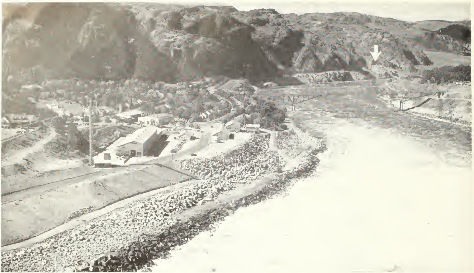
COLUMBIA, YOUR LINING'S SHOWING! —When this photo was taken in July 1950 from the top of Grand Coulee Dam, 320 feet above the river, the first two layers of Columbia River's armor plate riverbank protection had been placed—5 feet of small riprap covering a 2½-foot blanket of gravel. Heavy armor rock, blasted from the quarry on the west bank (see arrow), will cover the top bank. All photos for this article taken by F. B. Pomeroy, Region 1 photographer.
