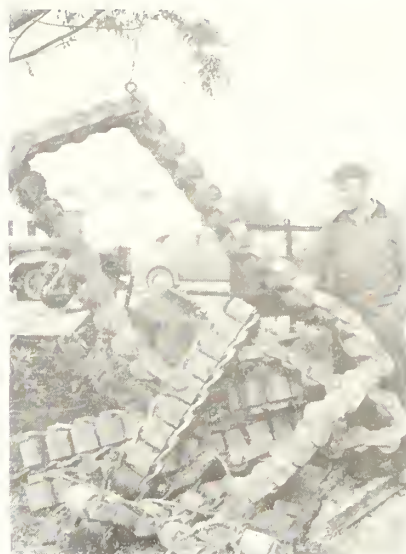
SAND-BLASTING the outlet tube at East Park Dam, above, preparatory to painting on July 19, 1949. DANGEROUS GATE STEM of Stony Gorge Dam, center photo, shows the broken screw threads which made it hazardous to operate the gate even partly, and absolutely impossible to operate if fully. FROZEN ROLLERS at left, from the Stony Gorge spillway coaster gate, show the rigidity of the roller train caused by corrosion and lack of clearance on pins.
