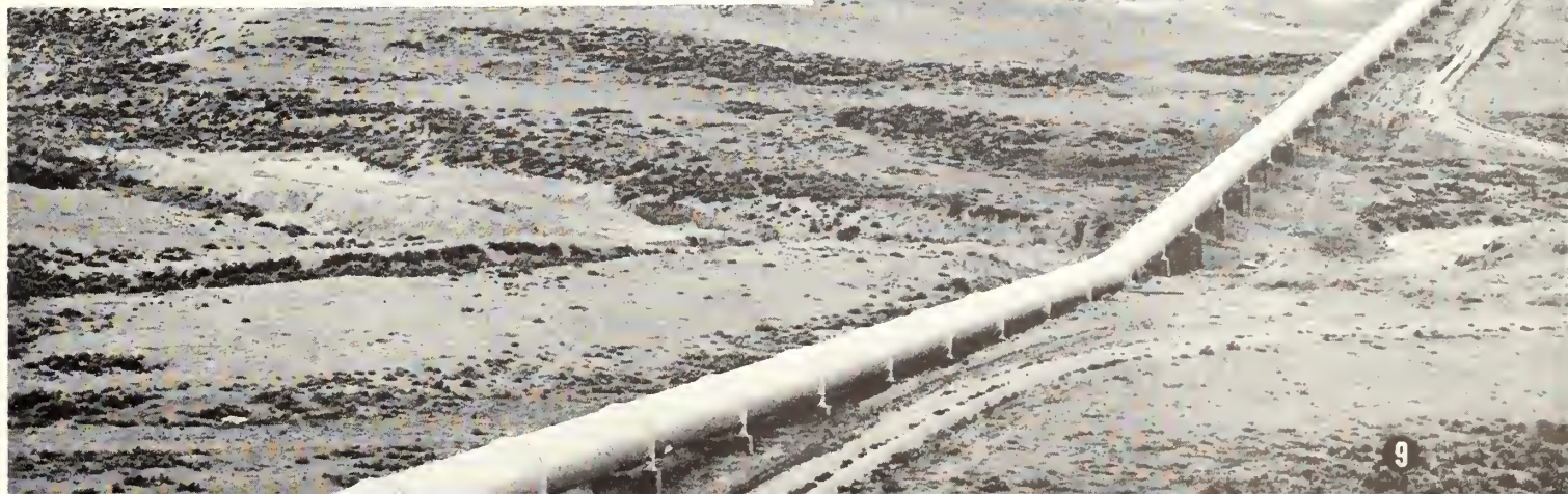
This scene approximately 17 miles north and east from Shoshone River siphon shows the Heart Mountain canal crossing Buck Spring Creek through an inverted siphon. Photo by Harold I. Sylten, of Region 6.
