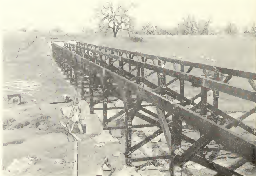
ROTTING TIMBERS (at left) typical of the condition of 30-year-old wooden structures on the Orland project in February 1949 before the reconstruction program started. Below, reconstructing the Highline Flume, a job which resulted in better water service and averted the threat of collapse.
