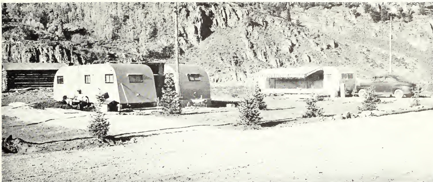
These Reclamation-designed trailer cottages are proving more popular than the usual construction camp home. At left: Typical dual unit cottage. One unit contains living, dining room, and kitchen; the companion unit contains two bedrooms and a bath. Photo by F. S. Finch, Region 5 photographer.
