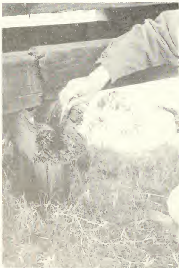
ROTTING TIMBERS (at left) typical of the condition of 30-year-old wooden structures on the Orland project in February 1949 before the reconstruction program started. Below, reconstructing the Highline Flume, a job which resulted in better water service and averted the threat of collapse.
