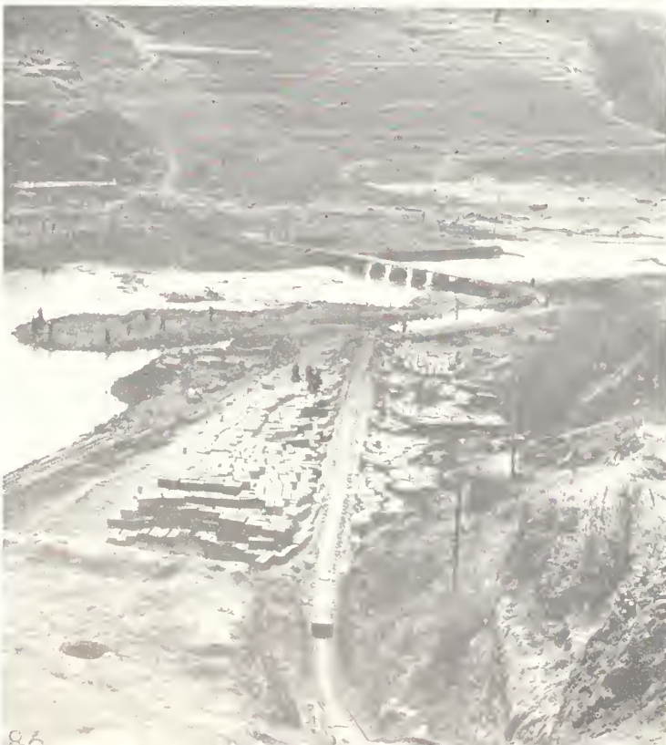
THE STONE BLOCK SLIDE —Looks like a railroad, but it goes "swish" instead of "chug." Stone blocks are loaded onto sleds at the top of the incline, and shoved off. The sled invariably stops near the center of the stock pile where it is unloaded, carried up the hill, and loaded for another slide. Note the terraces.
