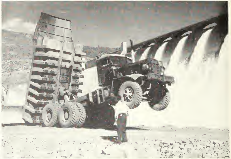
ROCK DWARFS MAN —Although Columbia River's granite armor rock must weigh a minimum of 3 to 6 tons, some rocks weigh up to 34 tons. The one at left is in the 20-ton class. The truck above weighs almost 60,000 pounds, and can carry 20 to 30 tons, but it is not uncommon for one or two huge boulders to lift the front wheels clear off the ground. A dozer, blade visible at left of photo, solved the truck driver's dilemma in this problem.
