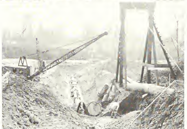
Above left: Removing old pipe line to avoid Rogue River highwaters. At top right: Precarious supports for old pipe line. Note new cylinder pipe being laid nearby. Immediately above: New concrete cylinder is seen edging toward river crossing. All photos by A. E. Baker, Region 1.
