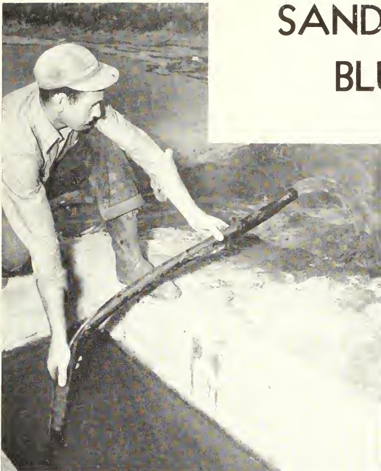
Jack Eickmeyer operating sand pump to remove silt from concrete chamber used to clean water before it enters pump and sprinkling system. Water and pressure required to operate jet-pump is obtained through garden hose from discharge side of sprinkler pump. Both photos by H. E. Foss, Region 1.
