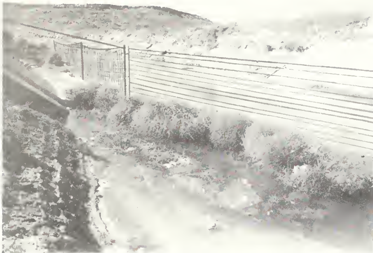
TRAPPED! Tumbleweeds are sliding down the wires, forced to make a detour into the weed trap "basket" on the main Conchas Canal.
