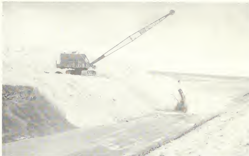
UNDER A BLANKET OF SOIL —A Bureau-operated dragline places a cover of earth 1 foot deep over newly sprayed asphalt membrane lining in the Wyoming Canal of the Riverton project, Wyoming. The cover soil is the same material excavated from the canal to smooth and grade it in preparation for the new lining. All photos for this article taken by Jewell R. Benson.
