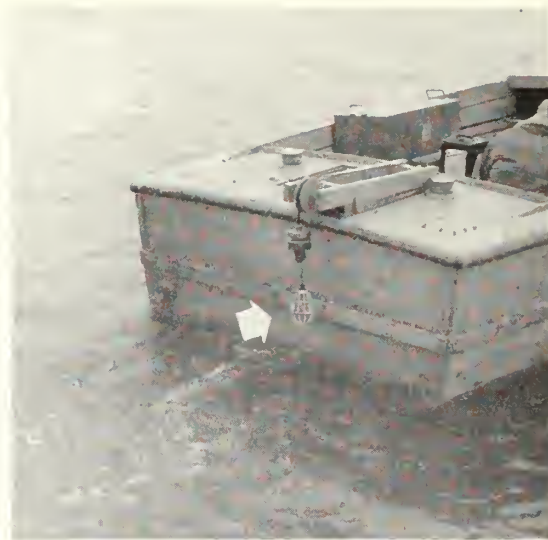
IT WRITES UNDER WATER —Or more properly, the thermistor bead shown in the center panel above sends messages which are recorded on the device in the boat (upper left). Once a week thermistor visits 16 specific locations, takes a dive to the bottom of Lake Hefner, and on the way down sends a continuous report on the temperature of the water to the recording machine.
