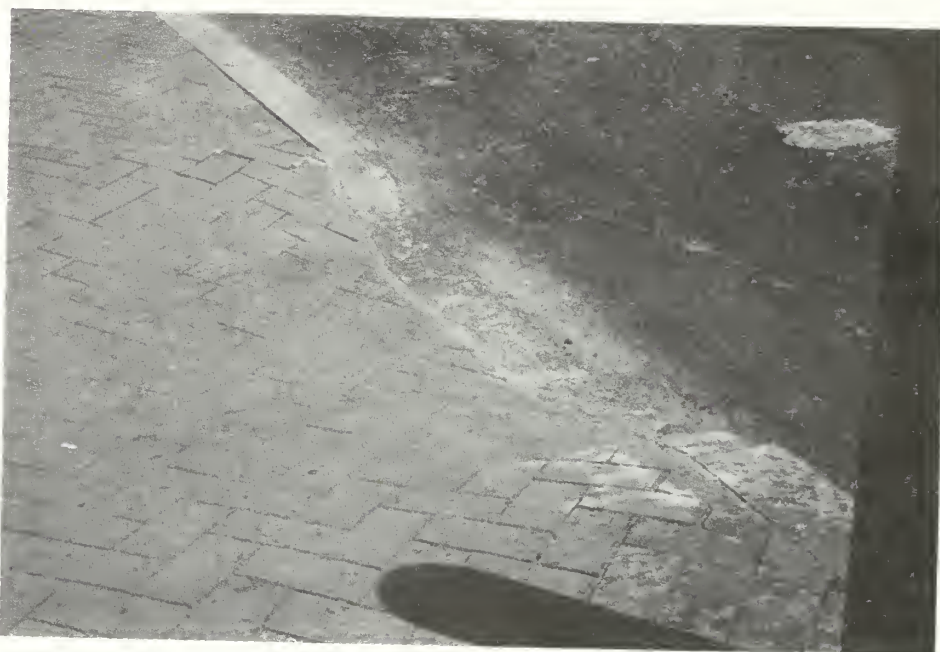
Photo 34: Granite curb was ground down creating a flush joint with the street paving.
