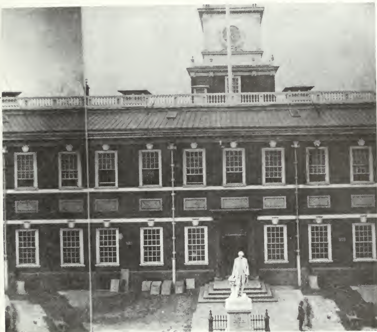
Photo 4: Laying flagstone on the Chestnut Street walkway, 1870. This stereo opticon view captured the work in progress to repave the Chestnut Street frontage with flagstone, replacing the earlier brick surface. Also visible in this view is the recently installed statue of George Washington and surrounding fence. From Independence NHP files, #33.
