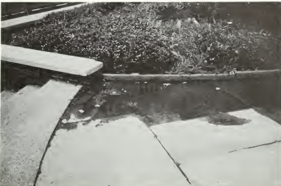
Photo 72: Many drop inlets are completely filled with silt and debris creating ponding.
