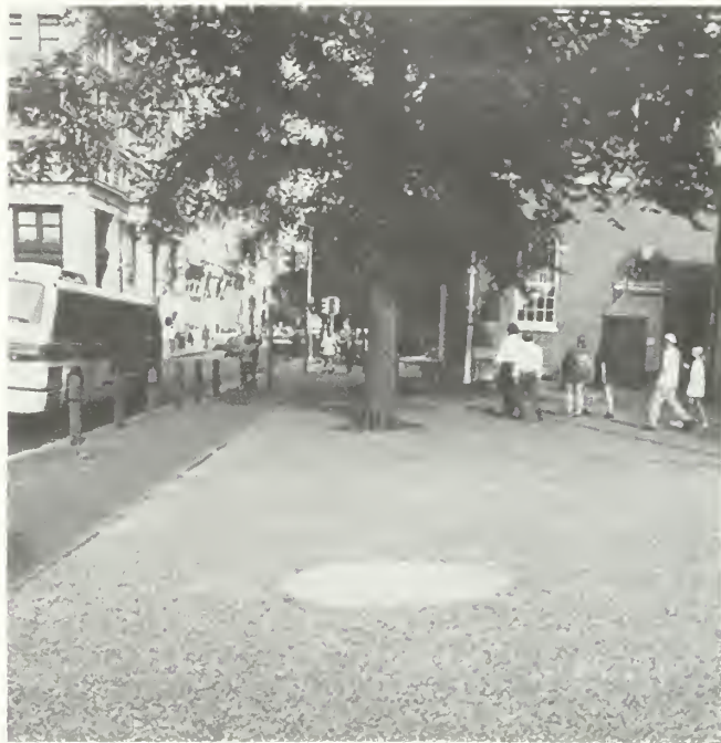
Photo 62: Patching of exposed aggregate paving indicates location of former double row of trees lining Chestnut Street in front of Independence Hall.
