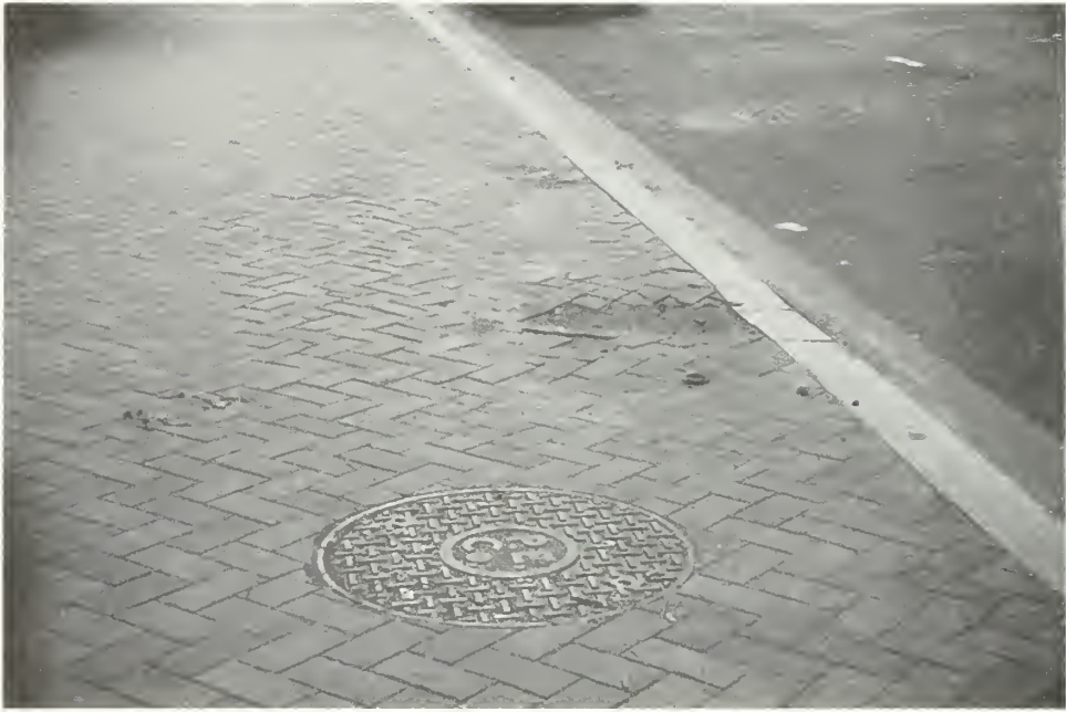
Photo 49: Damaged sidewalk brick paving along curb line.
