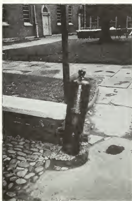
Photo 61: Paving at the base of the cannon is severely damaged.
