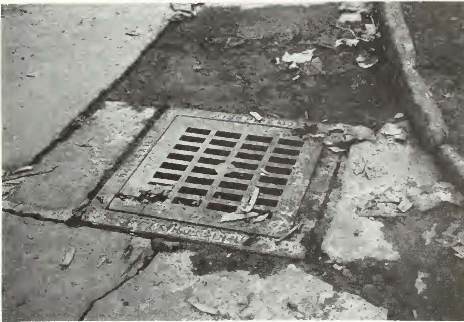
Photo 71: Pavement irregularities have caused many drain inlets to sit higher than the adjacent ground, resulting in little runoff collection.
