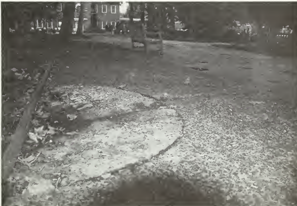
Photo 58: Central walkway apron tree well infilled with exposed aggregate paving.
