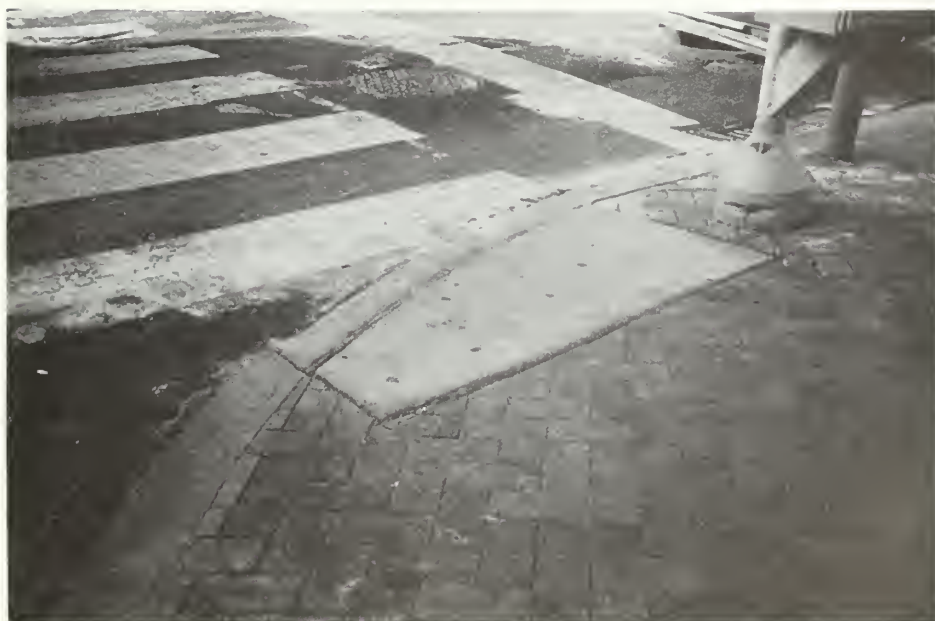
Photo 33: Concrete curb ramp is incompatible with adjacent stone curbing and brick paving.
