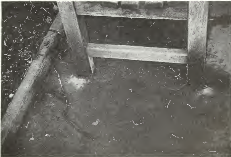
Photo 78: Bench anchoring brackets are embedded in the paving.
