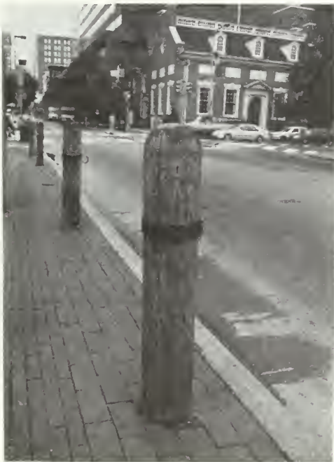
Photo 82: Wooden bollards found along Chestnut Street. Note the iron band with metal ring attached.
