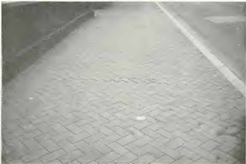
Photo 50: Subtle indications of settlement as indicated by depression in sidewalk brick paving.
