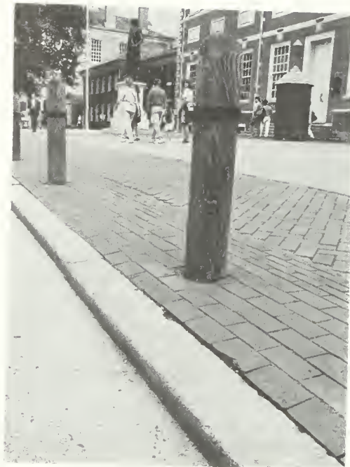
Photo 39: Running bond and herringbone patterns of brick paving and the adjoining exposed aggregate paving.
