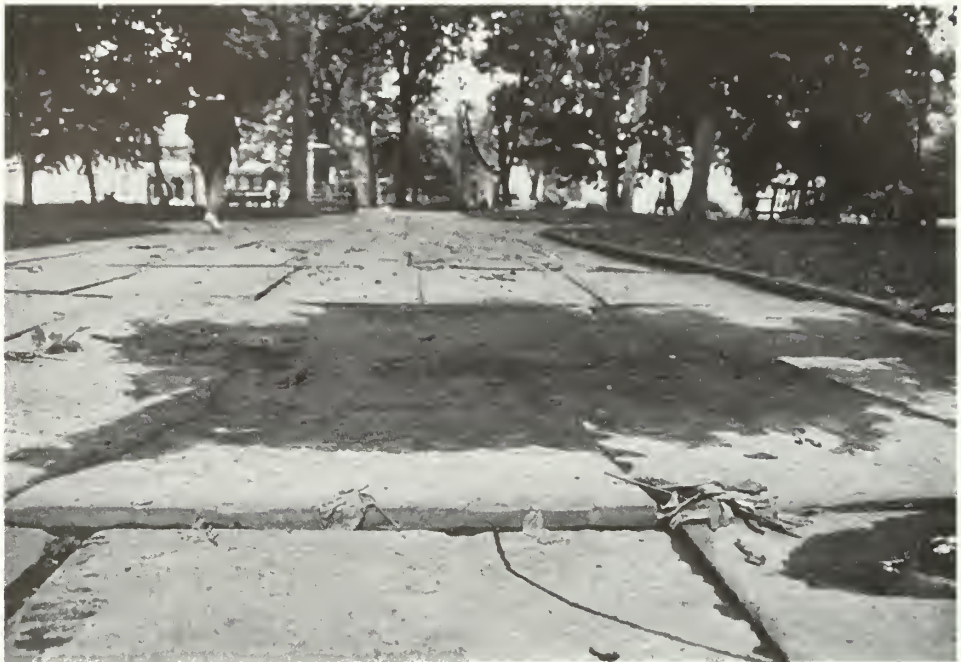
Photo 54: Bluestone paving damage resulting from subgrade settlement causes extensive ponding.
