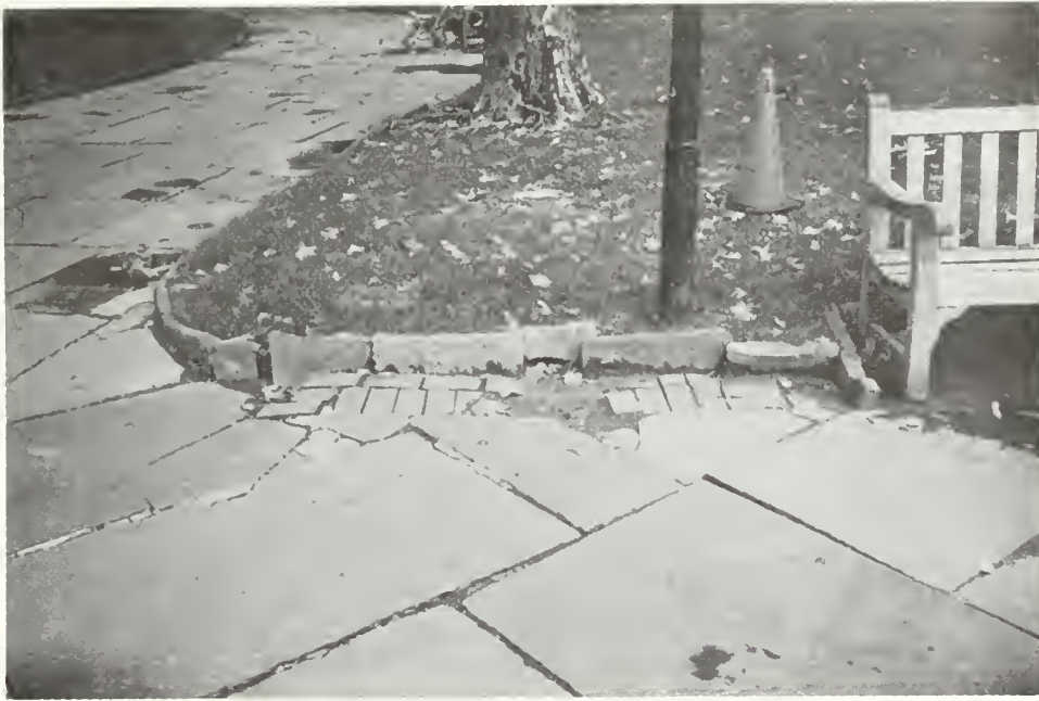
Photo 56: Damaged bluestone paving and stone curbing along lawn area. Note the infill brick pavement next to the bench.
