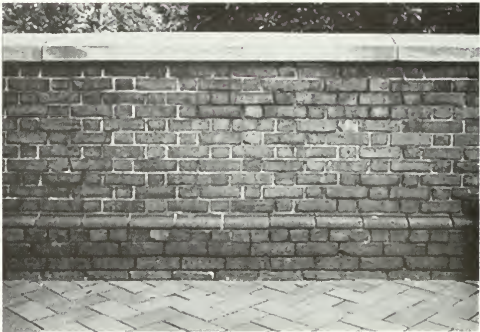
Photo 21: Brick retaining wall enclosing much of Independence Square. Note the white marble coping, Flemish bond, and molded brick water table at the base of the wall.
