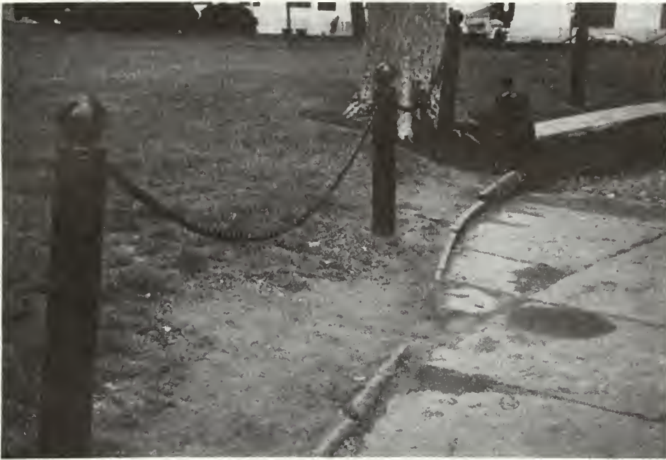
Photo 70: Soil compaction along heavily used paved areas results in loss of turf grass groundcover.
