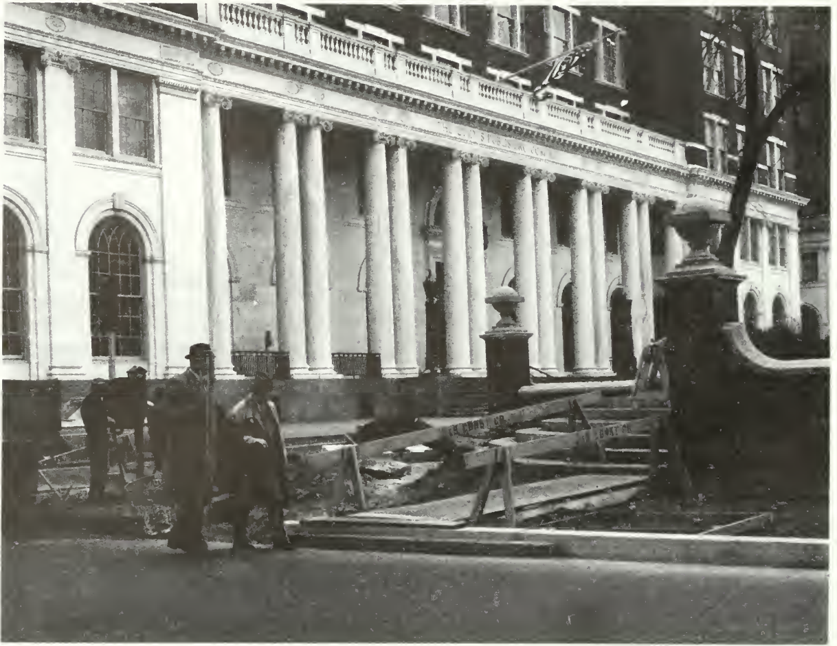
Photo 18: Repaving the sidewalks, 1962. In 1962 the National Park Service removed the flagstone sidewalks along the periphery of the square and repaved with brick in order to reflect the 18th century appearance.
