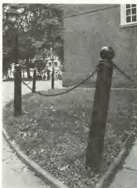
Photo 81: Cast iron bollards and chain barriers line the lawn areas south of Independence Hall.
