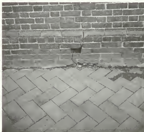
Photo 29: Typical "missing brick" style weep hole occurs every 30 feet along the base of the brick perimeter retaining wall.
