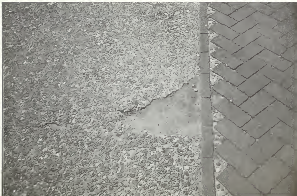
Photo 44: Example of cracked and spalled exposed aggregate paving along Chestnut Street in front of Independence Hall.
