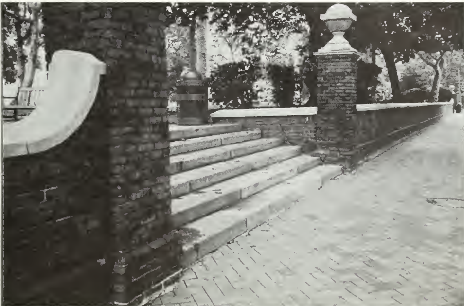
Photo 23: Central stairway along Walnut Street with brick piers flanking the marble steps. Note how brick wing wall meets grade at the top of the stairs.
