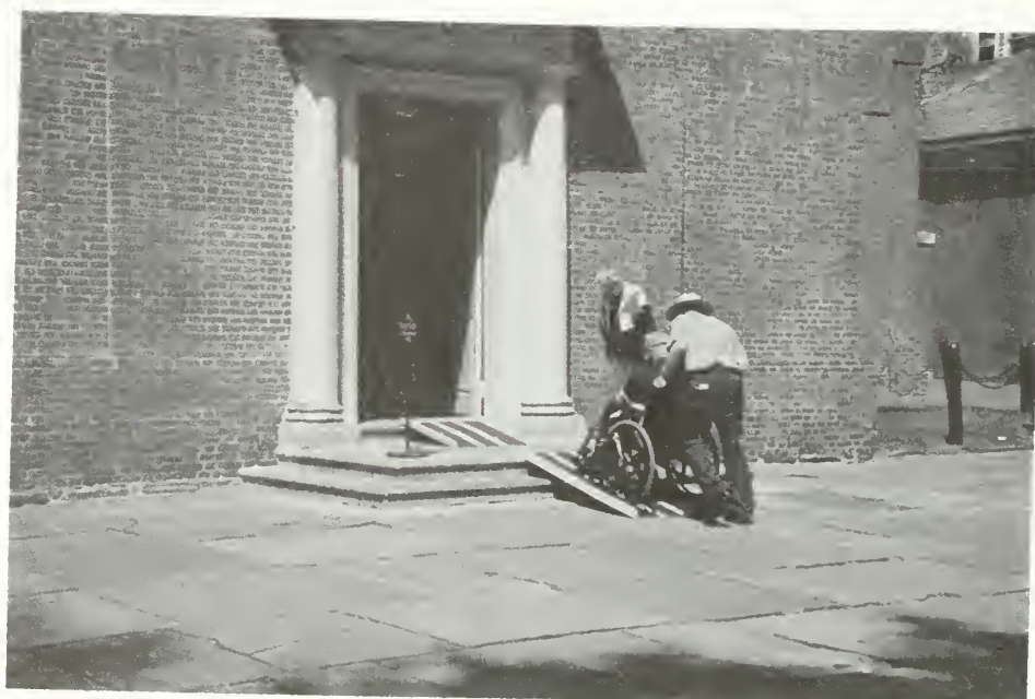
Photo 35: Moveable ramps providing disabled access to Independence Hall first floor.
