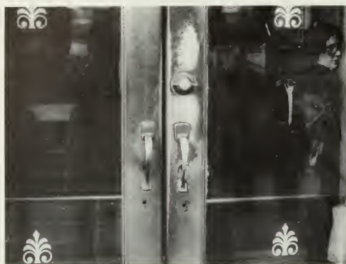
Figure 117. Human Abrasion At the Old Post Office in Baltimore, Maryland, the bronze and glass doors show the abrasive effect of human hands on the natural patina combined with a residue of dirt and oil (from skin, which contains a minute amount of acid). This wear with accompanying superficial discoloration is only a minor problem. Over the years, these doors have received inadequate maintenance and inappropriate changes (to the hardware) and repairs. Such doors should be thoroughly cleaned to the bare metal; the holes plugged, ground down, and polished; and new chemical artificial bronze patina applied and protected by a lacquer with a corrosion inhibitor and/or with periodic applications of wax or oil (see section on bronze Chapter 15). (David W. Look)
