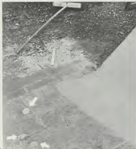
Figure 131. Salvaging a Flat Seam Terneplate Roof. (a) The roof of the Henry E. Bradford House Carriage Barn (c. 1860s) in Bennington, Vermont, had been covered with an asphalt coating (background) which obscured the true cause of the leaking roof. Once the asphalt coating was scraped from the surface (foreground left), it was noticed that the nails in the sheathing had "popped up" (light spots) and had cut through the terneplate. (b) After the asphalt coating had been scraped away and the nail holes repaired with solder (left foreground), the roof was then painted with red-lead primer (right foreground). The primed roofing was given two finish coats of iron oxide paint. (John G. Waite)
