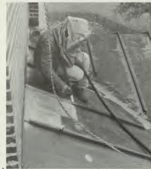
Figure 133. Abrasive Cleaning of Terneplate Roof and Replating. (a) Sections of the original terneplate roof at Lindenwald (Martin Van Buren National Historic Site) in Columbia County, New York, designed by architect Richard Upjohn in 1848, were cleaned with a low-pressure blasting of crushed walnut shells to remove accumulated paint and rust before replating with a lead/tin alloy. (b) The new terneplating was applied in localized areas (only where the original terne had been damaged by falling slates or removed because the sheet iron underneath had corroded). The new terneplating was applied where the bare iron was exposed using a soldering "copper" (a large soldering tool) fabricated for the project. After cleaning and replating, the restored roof was painted. (John G. Waite)
