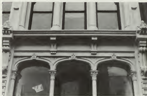
Figure 178. Aluminum Replacement of Minor Structural Elements of a Facade. For minor structural members without great loads, aluminum can be used as a substitute material; however, the capacity of a cast-aluminum column must be designed or checked by a structural engineer and not just assumed to be adequate. When the Grand Opera House in Wilmington, Delaware, was restored, missing cast-iron columns on the first-floor storefronts (flanking center bay entrance, lower center of photograph) were cast in aluminum to match the missing pieces of the original cast iron. (John G. Waite)
