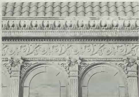
Figure 23. Pressed Copper Sheet Metal Cornice, Frieze, and Pilasters; Conservatory of the Christian Heurich Mansion, 1307 New Hampshire Avenue, NW, Washington, D.C., 1902; Appleton Clark, architect. The copper work was assembled from many pieces of sheet copper pressed with low relief designs. (Jack E. Boucher, NAER)
