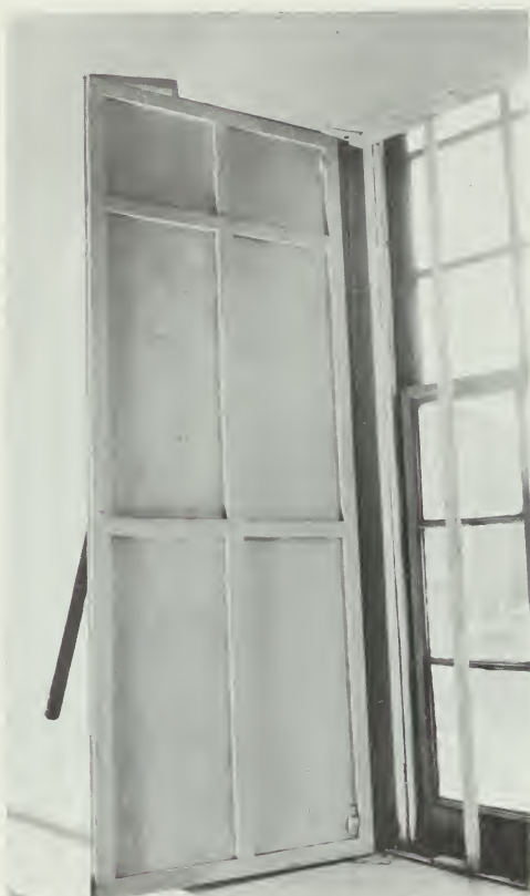
Figure 54. Wrought-iron Shutters, Arch Street Meeting House, 302-338 Arch Street, Philadelphia, Pennsylvania, 1803-1804; Owen Biddle, architect and master builder. The shutter is on the window of the "fireproof" vault used to store records. The iron shutter has a frame of hand-forged rectangular bars to which a series of rolled sheets was riveted. (George Eisenman)
