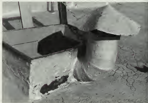
Figure 128. Deterioration of Tinplate by Asphalt Coating. The tinplate flashing of the roof hatch has been corroded away (between the corner and the vent) by the action of the asphalt coating and water. (John G. Waite)
