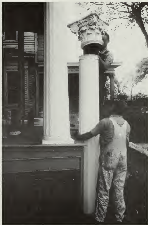
Figure 141. Repair of Galvanized Sheet Metal Capitals. (a) Fabricated for the 1890 Bullard-Hart House, Columbus, Georgia, these Corinthian capitals were originally assembled from many pieces of pressed sheet metal, which were soldered together to form the acanthus leaves. (b) The capitals were in salvageable condition and were taken to a sheet-metal shop where they were cleaned. Loose pieces were resoldered and caulked; missing pieces were replaced with new stamped pieces; and the completed capitals were repainted. The deteriorated wooden column shafts were repaired and repainted. The restored capitals were refitted onto the shafts and the entire columns were then returned to their original positions. (Thomas Taylor)
