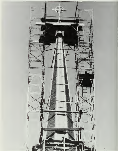
Figure 177. Reinforced Polyester Replica. The original cross of St. Agnes Church, Cohoes, New York, was removed from the steeple in the 1890s to serve as a grave marker. The original wrought-iron steeple cross, still intact, was used as a model to cast a new cross of reinforced (fiberglass) polyester. Fiberglass was chosen as a substitute material because of the inaccessible location (top of the steeple) where maintaining wrought iron (painting) would be difficult and expensive and because from the street level no one would be able to detect the substitute materials. (John G. Waite)
