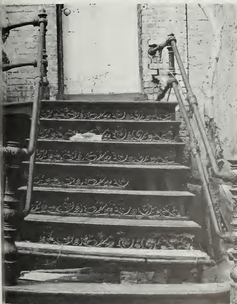
Figure 166. Damaged Cast Iron. This cast-iron perforated stoop in the 700 block of I Street, NW, in Washington, D.C., was fractured in several places because of differential settlement. As the right side of the stairs sank into the ground, the weight of the stoop was redistributed and induced shear, tensile, and torsion forces that were too great for the cast iron to resist. Differential settlement can also be caused by the upward and outward growth of a tree adjacent to a stoop and the downward settlement of a dead tree stump as it decays. Patching or repair work will be effective until the problem is corrected. The stoop should be disassembled and a new concrete foundation poured; the stoop can then be reassembled using welded fractured pieces and recast missing pieces. (David W. Look)
