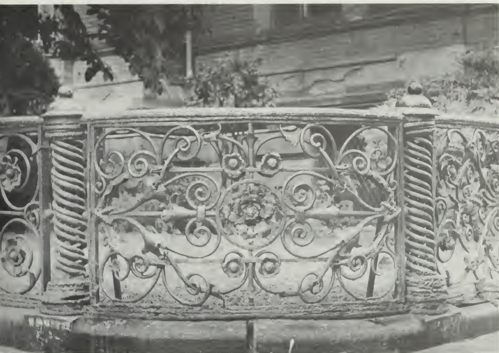
Figure 53. Wrought-iron Fence, Frederick Ames Mansion, 306 Dartmouth, Boston, Massachusetts, 1872; John Sturgis, architect. This fence was fabricated by hand from iron bars; square and round sections were hot-worked into spirals, circles, and scrolls. Even the fence posts are compact spirals of strong rods shaped about a central support to make them rigid. (Esther Mipaas)
