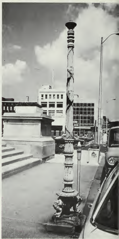
Figure 154. Damage to Bronze. In the Court Square Historic District in Springfield, Massachusetts, five of six bronze street lamps were vandalized or accidentally damaged by automobiles backing into parking spaces. (a) The one lamp that survived intact was used to make new molds. (b) The missing leg and lamp were recast (not shown) and/or repaired with funds from a matching grant from the National Park Service in 1976. The recast pieces were chemically treated to obtain a green patina that matched the weathered appearance of the original sections of the lamps. A plan was drafted to relocate the lamps 12 inches from their previous position at the curb to prevent any further damage from parking automobiles. (Thomas Taylor)
