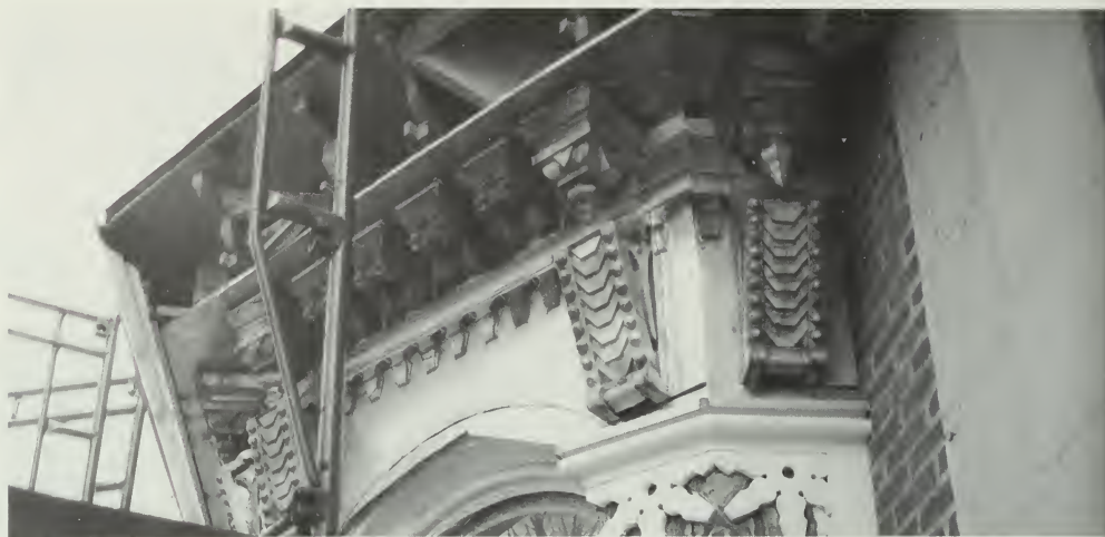
Figure 142. Restoration of Galvanized Sheet Iron and Cast-Zinc Cornice. This is the upper third of a wooden bay window on a Second Empire brick rowhouse in the Logan Circle Historic District of Washington, D.C. (a) From the window down, the bay is wood and glass. The roof of the bay had leaked for years and the wooden roof rafter and projecting supports for the cornice had rotted. The bay window was carefully disassembled and rebuilt replacing all deteriorated lumber. The surviving pieces of galvanized sheet-iron and cast-zinc cornice were taken to a sheet-metal shop. The pieces that were repairable were cleaned; missing portions of brackets on the right were replicated of galvanized sheet iron using the originals as a model. (b) On the opposite side of the bay, all of the brackets and modillions are repaired originals but all of the flat and molded sections are new 26-gauge galvanized steel. The 65-year-old sheet-metal worker on this job said that the only two major advances in metal cornices in his lifetime are the use of pop rivets for fasteners (used also in leatherwork) and the use of autobody putty to patch holes, mold small missing details, and waterproof joints. The putty dries hard and can be sanded. (David W. Look)
