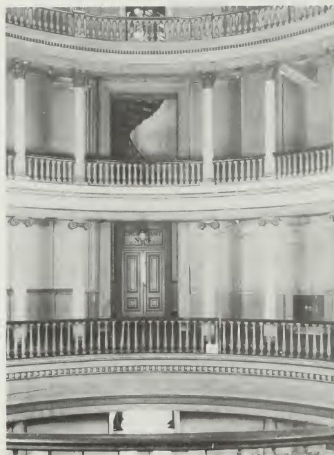
Figure 73. Rotunda Galleries, Old St. Louis Courthouse, Fourth and Market Streets, St. Louis, Missouri, 1859 expansion; William Rumbold, architect. The courthouse has many iron elements, including the intricate elliptical cast-iron staircases in the wings and half of the Ionic and Corinthian columns which support the rotunda galleries. Every other column is wood. The cast-iron columns were added to take the increased load of the dome, a major feat of engineering and architectural design. William Rumbold accomplished the detailed engineering of the dome between 1859 and 1862, one and one-half years before the dome of the U.S. Capitol was completed. (Piaget, NAER)
