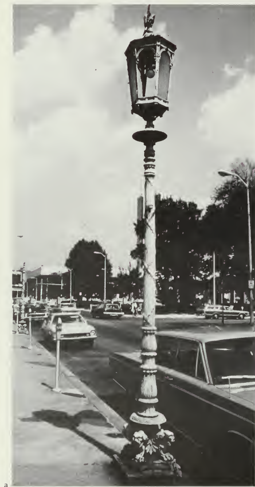
Figure 154. Damage to Bronze. In the Court Square Historic District in Springfield, Massachusetts, five of six bronze street lamps were vandalized or accidentally damaged by automobiles backing into parking spaces. (a) The one lamp that survived intact was used to make new molds. (b) The missing leg and lamp were recast (not shown) and/or repaired with funds from a matching grant from the National Park Service in 1976. The recast pieces were chemically treated to obtain a green patina that matched the weathered appearance of the original sections of the lamps. A plan was drafted to relocate the lamps 12 inches from their previous position at the curb to prevent any further damage from parking automobiles. (Thomas Taylor)
