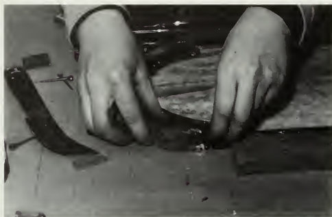
Figure 126. Lead Came Replacement. (a) On the table is a tracing of the original pattern of the lead comes of a late 19th-century stained glass window from the Pilgrim Congregation Church, Cambridge, Massachusetts. Because of the severe deterioration of the original lead comes, it was necessary to replace them with new comes that matched the original configuration. (b) This is a detail of the fitting of the new comes around the original glass. (Cummings Studios)
