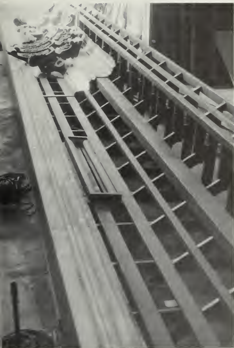
Figure 143. Preassembling Cornice. As illustrated in figure 122, most sheet-metal cornices were supported by wooden support members projecting out from the facade of the building, either as an extension of the roof framing or as a cantilever from a parapet wall. In either case, these wooden support members are often found to be rotten and have to be replaced. For large cornices high above the street level, it may be economically unfeasible to use scaffolding for in situ repairs and reconstruction unless the scaffolding is also needed for other work. The entire galvanized sheet-iron cornice of the ZCMI Store in Salt Lake City, Utah, was preassembled on the ground with repaired original parts and new pieces onto a new support system fabricated on mild steel angles. Fifty-foot sections of the preassembled cornice were then hoisted to the top of the facade and bolted to the building without the need for scaffolding. (Steven T. Ward)
