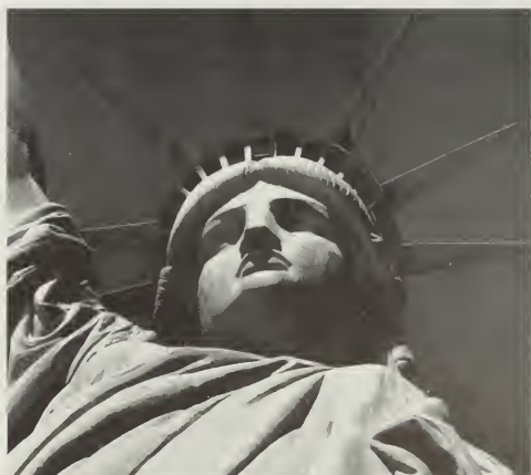
Figure 149. Resistance to Corrosion. Little damage had occurred to the copper at The Statue of Liberty. Galvanic corrosion, however, occurred where saline rainwater provided the electrolyte between the copper and the iron armature, resulting in considerable loss in the cross-section of the armature. (Robert Baboian)
