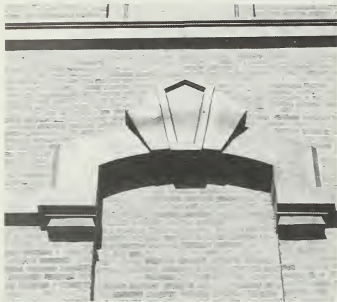
Figure 137. Deterioration of Zinc. At the 1874 Cohoes Music Hall, Cohoes, New York, the original zinc window lintels and belt course were cleaned by sandblasting, resulting in pitting and corrosion of the metallic surface. Note the whitish corrosion products caused by the abrasive cleaning and subsequent exposure to the weather. The lintels had been painted originally but were left bare after the cleaning. Zinc and galvanized sheet iron should always be primed and painted with paints especially formulated for zinc. (John G. Waite)
