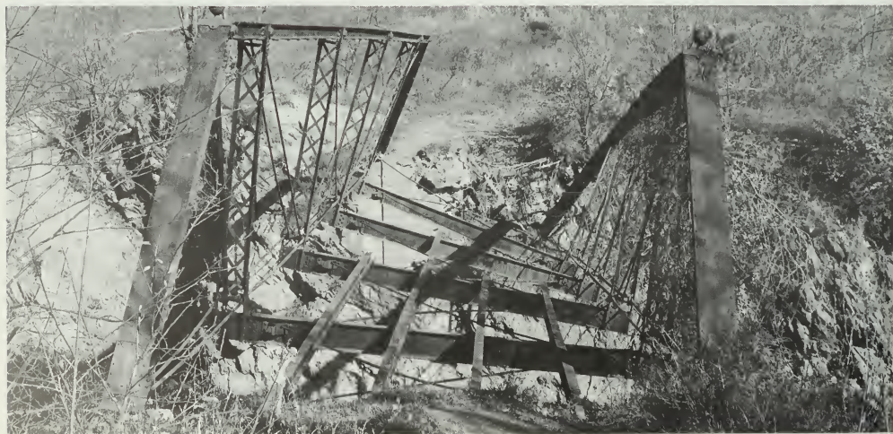
Figure 122. Structural Failure. This 19th-century wrought-iron truss bridge at Brunswick, New York, partially collapsed because the cut-stone abutment supporting it washed away. Once the support was removed, the bridge twisted. (John G. Waite)
