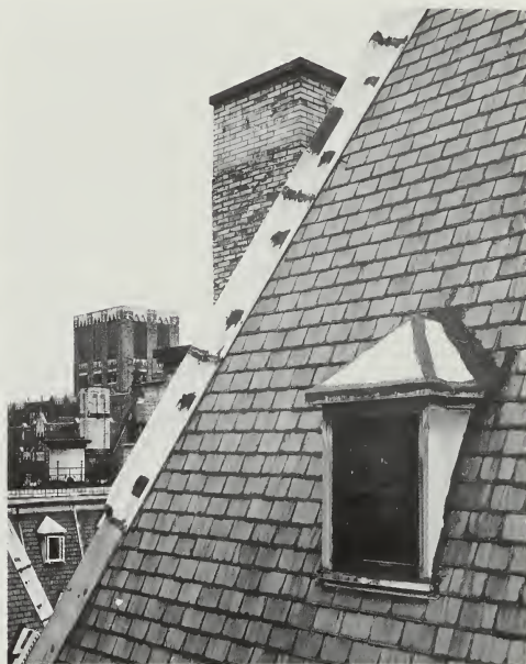
Figure 148. Inappropriate Patching Compounds.
