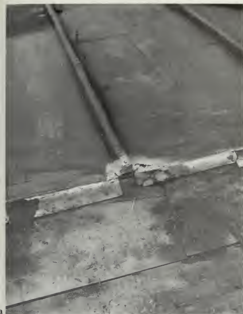
Figure 132. Repair and Replacement of Terneplate Roofing. (a) The ends of the original terneplate batten covers at Lindemould were badly corroded and could not be replated. (b) The unsalvageable sections were cut out and replaced with terne-coated stainless steel soldered in place. (c) The deteriorated terneplate valley was replaced with sheets of terne-coated stainless steel; the terne coating allowed the valley to be soldered to the original roofing plates. Although terne-coated stainless steel was a good choice, in theory, it proved to be a difficult material to work with in the field. (Correctly, the availability of thinner gauges and a more malleable stainless steel have improved the workability of this material.) (d) The original terneplate had rusted through completely in some areas, requiring reroofing. New sheets of terne-coated stainless steel, duplicating the pattern of the original terneplate, are being laid over rosin paper. (John G. Waite)
