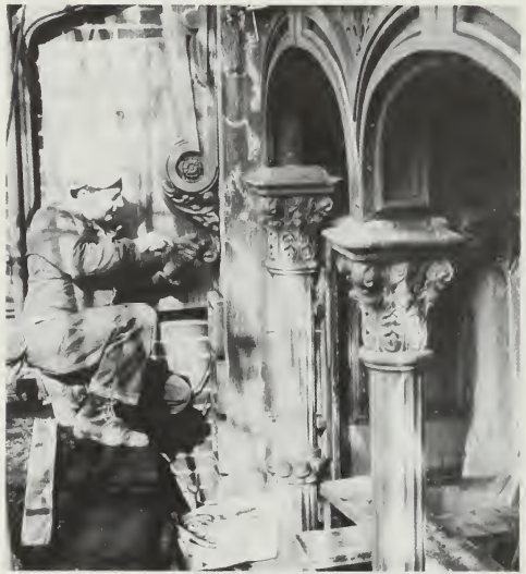
Figure 174. Erection of Cast-Iron Facade. To assemble the Main Street shop facade of the Wilmington Grand Opera House, many assembled sections and individual pieces were shipped to the job site where they were screwed and bolted together in their final positions. (Steven T. Baird)
