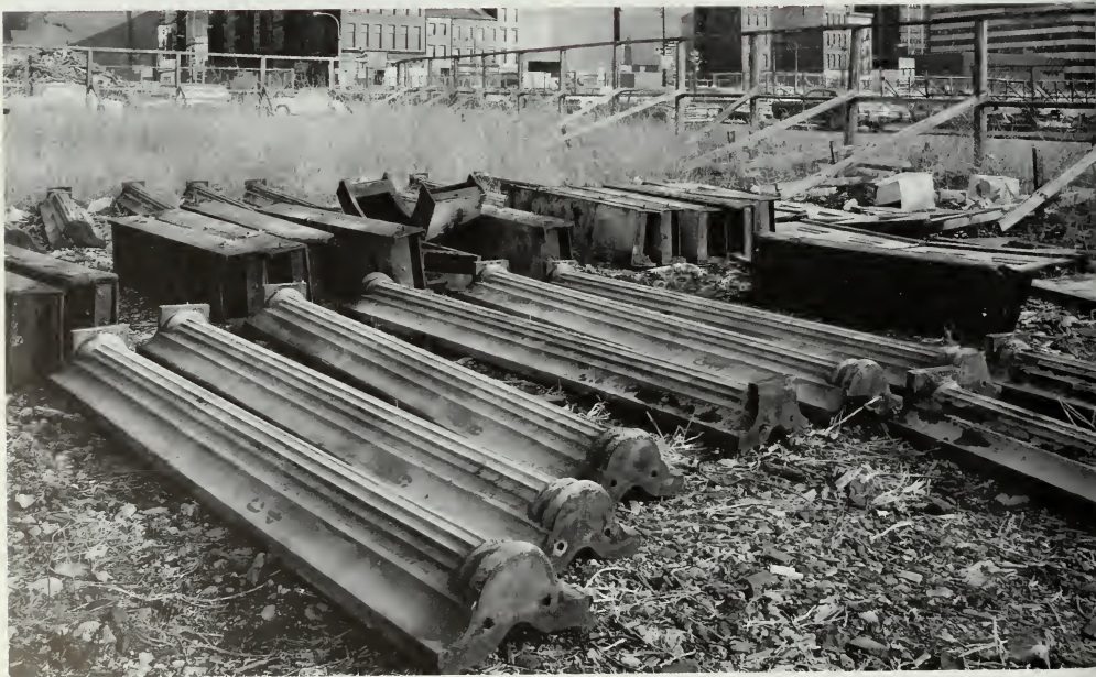
Figure 168. Dismantled Cast-Iron Facade. The Edgar Laing Stores in New York City were erected by James Bogardus in 1849 and had one of the earliest cast-iron facades. The building was demolished in 1971 for an urban renewal project, but its cast-iron facade was carefully dismantled so it could be reerected on another site at a later date. Unfortunately, while the components were in storage, most of them were stolen and apparently sold for scrap. Dismantling of a building should be considered a measure of last resort, to be attempted after all other efforts to save a building in situ have failed. (Jack E. Boucher)
