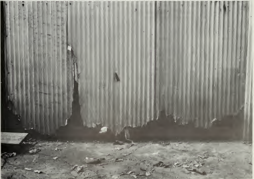
Figure 182. Corrosion and Severe Deterioration of Aluminum. The corrugated aluminum siding on a commercial building in Green Island, New York, has been severely deteriorated by the splashing of water and snow-melting salts. (John G. Waite)
