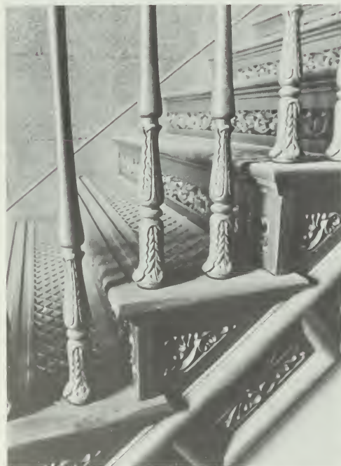
Figure 81. Restored Cast-iron Stairs, Old Customs House (now known as West Virginia Independence Hall), Wheeling, West Virginia, 1859; Ammi B. Young, Architect of the Treasury. In this building the people of western Virginia declared their independence during the Civil War and joined the Union. These cast-iron stairs and balusters have recently been restored with the recasting of missing or damaged pieces. Perforated stairs were originally designed to combine decorative, functional, and economical detailing; to provide elaborate but strong construction; and to reduce the weight and quantity of iron required. (West Virginia Independence Hall Foundation)
