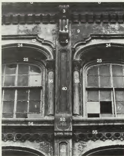
Figure 165. Sequence of Dismantling. Once the bolts and screws have been located, the parts can be numbered. The numbers on the photograph indicate to the contractor the order of disassembling the cast-iron facade, which is the reverse order of its original erection. (Steven T. Baird, AIA)
