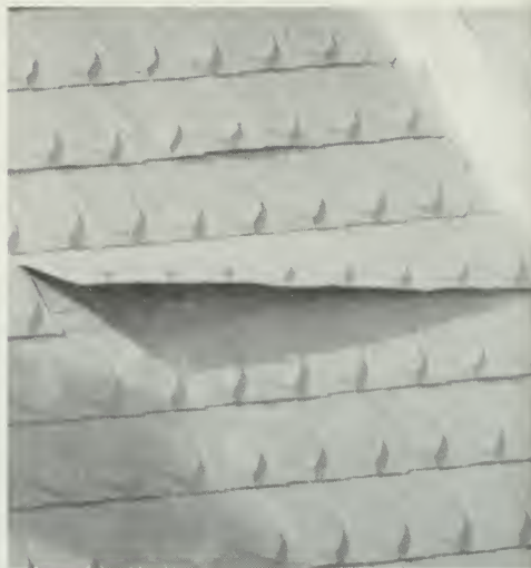
Figure 123. Anchorage Failure. The nails holding down this section of embossed galvanized sheet-iron roofing have deteriorated and the wind has lifted up the corner of the sheet, allowing water to leak through the roof sheathing. Other sections (not shown in the photo) had flapped in the wind until the sheet metal cracked with fatigue failure and tore loose. In 1977 this roof at St. Edward's University in Austin, Texas, was cleaned and supplemented with reproduction "shingles" where needed. (St. Edward's University)
