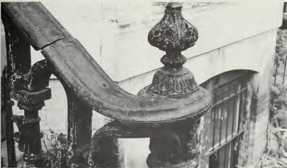
Figure 160. Cast-iron Corrosion, Fracture, and Missing Pieces. (a) The massive newel posts of the stair railings on the entrance of 637 I Street, NW in Washington, D.C., are hollow and are made up of several pieces screwed and bolted together. The newel post to the right side of the stairs is substantially intact. (b) The finial of the left newel post is missing. Note the threaded rod in the center of the newel post used for assembly. Inside the railing, loose rust has collected to a depth of about a half inch. Water seeped into the hollow rail and froze, resulting in the crack. (David W. Look)
