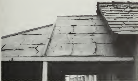
Figure 119. Creep. Deterioration of milled sheet lead roof on a 19th century canal warehouse and office at Nantwich Basin of the Shropshire Union Canal at Nantwich, Cheshire, England. The failure has been caused by creep and the expansion and contraction of the lead. (John G. Waite)
