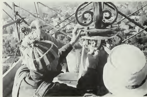
Figure 177. Reinforced Polyester Replica. The original cross of St. Agnes Church, Cohoes, New York, was removed from the steeple in the 1890s to serve as a grave marker. The original wrought-iron steeple cross, still intact, was used as a model to cast a new cross of reinforced (fiberglass) polyester. Fiberglass was chosen as a substitute material because of the inaccessible location (top of the steeple) where maintaining wrought iron (painting) would be difficult and expensive and because from the street level no one would be able to detect the substitute materials. (John G. Waite)
