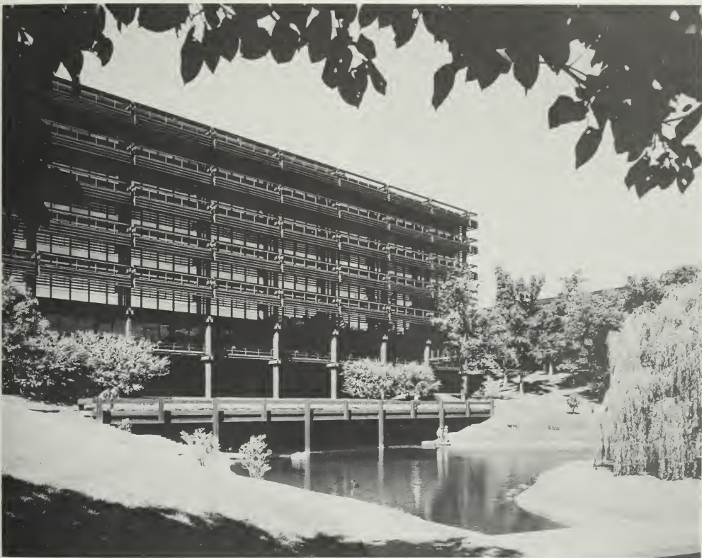
Figure 110. "Corten" Steel, Deere and Company Administrative Center, Moline, Illinois, 1964; Eero Saarinen, architect. The Deere and Company building, which received many architectural awards, was among the first to make extensive architectural use of this unpainted, corrosion-resistant material for exterior steel members. (Deere and Company)
