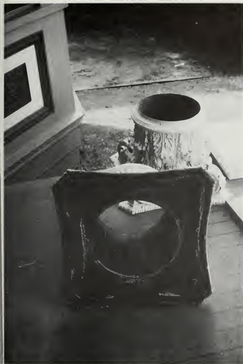
Figure 141. Repair of Galvanized Sheet Metal Capitals. (a) Fabricated for the 1890 Bullard-Hart House, Columbus, Georgia, these Corinthian capitals were originally assembled from many pieces of pressed sheet metal, which were soldered together to form the acanthus leaves. (b) The capitals were in salvageable condition and were taken to a sheet-metal shop where they were cleaned. Loose pieces were resoldered and caulked; missing pieces were replaced with new stamped pieces; and the completed capitals were repainted. The deteriorated wooden column shafts were repaired and repainted. The restored capitals were refitted onto the shafts and the entire columns were then returned to their original positions. (Thomas Taylor)
