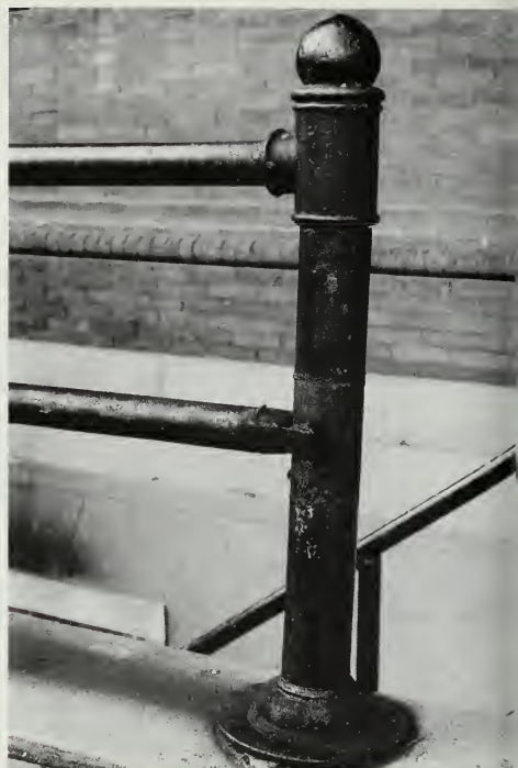
Figure 161. Inappropriate Repairs of Cast Iron. A simple cast-iron pipe railing guards the areaway of the Old Pension Building in Washington, D.C. The collar on the newel post to receive the bottom rail is missing (it probably cracked off from the pressure of expanding rust and/or ice). Unfortunately, a strap was welded to each side instead of repairing or reproducing the collar. (David W. Look)
