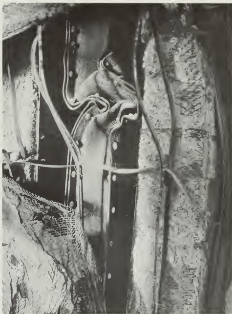
Figure 120. Column Buckling from Fire. In 1906 San Francisco was shaken by a severe earthquake, followed by fires that raged out of control for hours. In the Fairmont Hotel, the metal lath and plaster that covered the columns was probably damaged by the earthquake and was not sufficient to protect the steel from the intense heat. Portions of this building settled down approximately 7 feet from their original position because 37 columns buckled from the heat in this manner. (From Trial by the Fire at San Francisco: The Evidence of the Camera, 1906, Library of Congress.)
