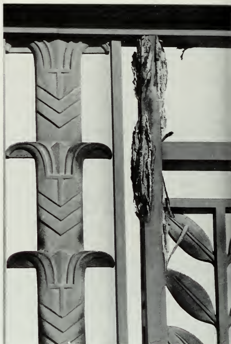
Figure 183. Exfoliation Deterioration. In Washington, D.C., at the Folger Shakespeare Library designed in 1932 by Paul Phillippe Cret, the aluminum alloy balcony railing began to exfoliate in layers, similar to rusting wrought iron. The corrosion product was grayish white and lifted up from the surface as if the metal had exploded. All of the cast ornamental sections were in relatively good condition; only the straight, bar stock was affected. The original specifications stated that the railing was to be an aluminum and chromium alloy. However, a recent laboratory report analyzed a four inch section cut from a sound piece of metal next to a corroded area and indicated that it was high-copper alloy (structural aluminum) fitting into the category of alloy 2017, which is not recommended for exposed outdoor use since it is not corrosion resistant. It is amazing that it lasted 47 years outdoors. All of the straight bar stock of the railing should be replaced with alloy 6063. The cast ornament could be cleaned and reused since they are obviously of more corrosion-resistant alloy and show no signs of deterioration. (David W. Look)
