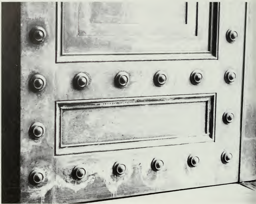
Figure 153. Improper Cleaning of Bronze. The bronze doors on the Pennsylvania Avenue side of the National Archives in Washington, D.C., were cleaned improperly. They now vary in color from a golden bronze to green to copper orange and brassy yellow. Some of the original artificial patina applied at the foundry has been removed, leaving a blotchy appearance. Part of the corrosion from the deicing salt remains, and the doors have a streaked, unattractive appearance. At this point, the only feasible treatment would be to clean the doors thoroughly (down to the bright metal), by mild chemicals or soft abrasive cleaning. A new artificial patina could be applied to return the doors to their original appearance. To protect against future damage, the doors should be given a barrier coating of wax which will need to be renewed periodically. The maintenance staff should be notified not to use salt near the doors and not to clean or polish the doors other than washing them down once a year with a nonionic detergent. When washed, the doors should be thoroughly rinsed with distilled water and wiped dry with a clean cloth to prevent water spots and streaks. (David W. Look)
