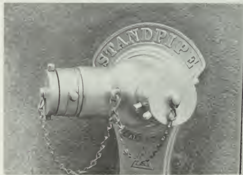
Figure 37. Brass Siamese Standpipe Connection, Rookery Building, 209 South LaSalle Street, Chicago, Illinois, 1886; Burrham and Root, architects; W. D. Allen, manufacturers. Brass fittings can be functional and very attractive when kept well polished. Even though the natural weathered dark patina on brass is protective, it is generally considered to be unsightly and great effort is expended to recapture the metallic gleam. (Margot Gayle)
