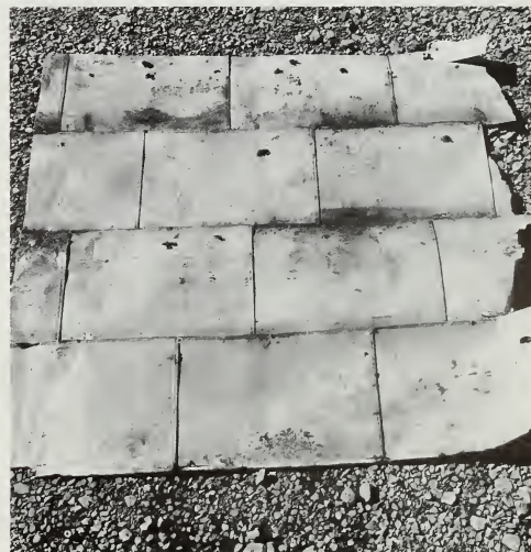
Figure 129. Corrosion Failure of Terneplate Roofing. Hyde Hall, built between 1817 and 1833, near Cooperstown, New York, was roofed with flat-seam terneplate. (a) The plates have deteriorated because of a lack of proper maintenance. Unfortunately, the exposed (top) surface of the terneplate was painted with asphalt coating, which accelerated the corrosion of the roofing. (b) The terneplate also corroded from the underside. When installed, the terneplate was not painted on the underside as it should have been. Condensation formed on the unprotected bottom side of the metal roof and could not evaporate, an ideal situation for corrosion. (John G. Waite)
