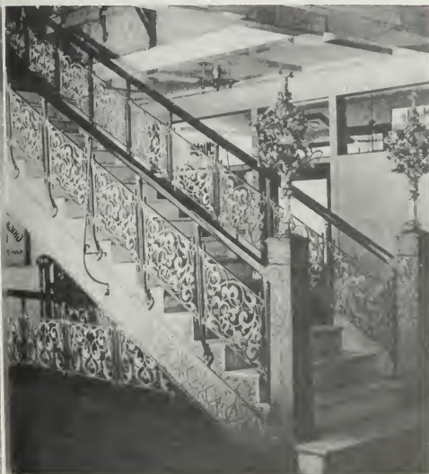
Figure 112. Cast Aluminum Staircase, Monadnock Building, 13 West Jackson Boulevard, Chicago, Illinois; Burham and Root, architects; Winslow, Brothers, Co., foundry. Although the Monadnock Building is widely known as the last skyscraper with load bearing walls, few people know that it contains the second known architectural use of cast aluminum in America. The first story staircase, including the newell posts, electroliers, balustrade railing, facias, and stringers, are all cast of aluminum. The lamps have been removed. Aluminum ventilation grilles near the exterior doors are also illustrated, but have also been removed. (plate 4, Collection of Photographs of Ornamental Iron Executed by Winslow Bros., 1893, Library of Congress)
