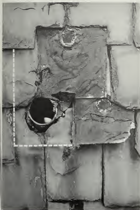
Figure 139. Zinc Corrosion, Erosion, and Inappropriate Repairs. In construction of the Nott Memorial at Union College in Schenectady, New York, during the 1870s, architect Edward Tuckerman Potter used "illuminators" in the ornamental slate roof. These were slate-sized zinc plates with a small colored-glass disc 1 3/4 inches in diameter inserted in the center. Barely discernible from the outside, they transformed the vaulted dome within a "heaven" of red, yellow, purple, orange, and green stars. Shown here is a cluster of three illuminators, each consisting of a zinc plate with a small colored-glass insert and the connecting tube through the metal deck and plaster to the interior. The zinc was inaccessible and not kept painted. Small fragments of slate broke off and tumbled down with gravity. The wind and rain eroded away the layer of corrosion from the zinc surface. The left plate is missing (see dotted line), showing the connecting tube. The corner of the lower right plate is missing because it became brittle and fractured off. Unfortunately, modern roofing cement applied over the zinc plates is accelerating the deterioration. (John I. Mesick, The Nott Memorial: A Historic Structure Report Schenectady, New York: Union College, 1973, p. 65)
