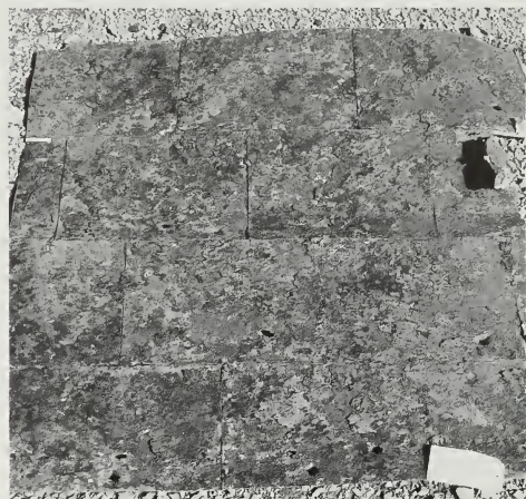
Figure 129. Corrosion Failure of Terneplate Roofing. Hyde Hall, built between 1817 and 1833, near Cooperstown, New York, was roofed with flat-seam terneplate. (a) The plates have deteriorated because of a lack of proper maintenance. Unfortunately, the exposed (top) surface of the terneplate was painted with asphalt coating, which accelerated the corrosion of the roofing. (b) The terneplate also corroded from the underside. When installed, the terneplate was not painted on the underside as it should have been. Condensation formed on the unprotected bottom side of the metal roof and could not evaporate, an ideal situation for corrosion. (John G. Waite)
