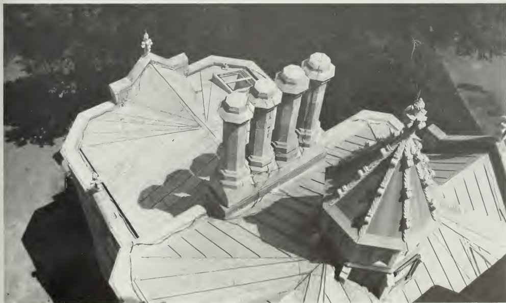
Figure 135. Complete Substitution of Lead-Coated Copper Roofing for Terneplate Roofing. The 1864 wing addition of Lyndhurst, Tarrytown, New York, originally had a terneplate roof. In an attempt to find a more permanent roofing material, a lead-coated copper roof was substituted for the terneplate, duplicating the pattern and sheet sizes of the original roof. In such substitutions, details may have to be redesigned because of differences in expansion and contraction rates and differences in workability of the material. The color of lead-coated copper is not the same as terneplate because terneplate roofing was never left unpainted. Therefore, lead-coated copper roofing substituted for terneplate should also be painted if it seen from normal viewing angles (usually from street level). (John G. Waite)
