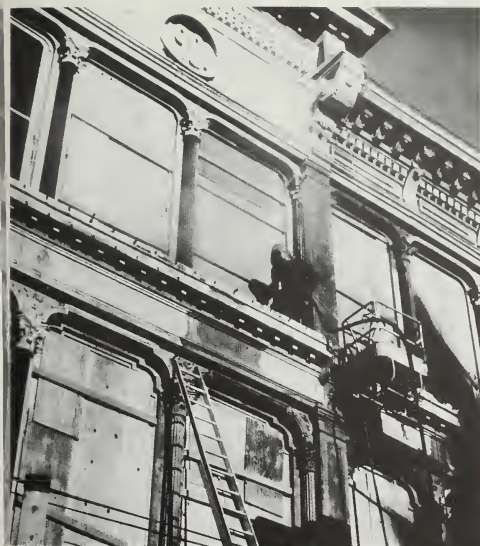
Figure 163. Cleaning Cast Iron. The facade of the Zions Cooperative Mercantile Institute (ZCMI) Store was sandblasted to locate the screws and bolt connections and thereby discover the method of assembly and disassembly. The cast iron should not be heavily sandblasted (down to the bare metal) unless that entire section of the facade is being dismantled. As pieces are being removed, they should be primed immediately to avoid rusting. If the building is not to be dismantled, it is best to remove only the loose paint with a wire brush, being careful not to damage caulked joints and connection holes. Any bare cast iron should be spot primed. Steven T. Baird, AIA)
