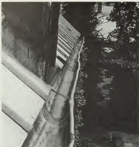
Figure 121. Overloading. The copper gutter on the Senate House, Kingston, New York, installed in the 1920s, has been distorted by ice and snow; the seams between gutter sections have opened. The problems were compounded by the lack of stiffness of the gutter and the absence of adequate provisions for expansion and contraction. The steel restraining straps are deteriorating because of an electrolytic reaction (galvanic corrosion) with the copper (the more noble metal). (John G. Waite)
