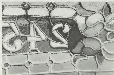
Figure 125. Lead Came Damage. One of the most common uses of lead is the comes in stained glass windows, transoms, and skylights (see figure 8). Although lead comes are sometimes damaged by corrosion, especially where rain or condensation might collect at the bottom border came (a very slow process), they usually are damaged by creep and fatigue. The weight of the lead and glass in the entrance transom pictured above has caused the comes to creep, resulting in a noticeable sag and outward bulge. This transom did not have iron support bars found on many stained glass windows. The bars (sometimes called saddle bars) were usually set into the frame and attached to the lead comes with copper wires. Transoms are adversely affected by the vibrations of slammed doors and the outward force of compressed air in a vestibule. To complicate things further, the difference in the expansion and contraction coefficients of the lead comes and lead-tin solder has resulted in fatigue cracking, usually at joints. (H. Weber Wilson)
