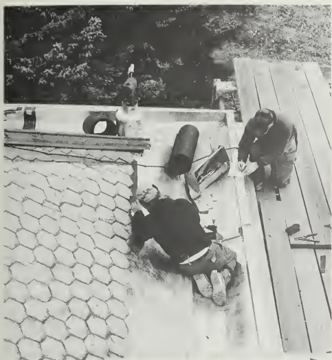
Figure 134. Replacing Flashing and Gutters. Workmen replaced the deteriorated terneplate flashing and gutters at Olana, built between 1870 and 1874 near Hudson, New York, for the noted artist Frederic E. Church. The polychromed slate roof was restored to the original pattern, and lead-coated copper was substituted for the original terneplate flashing and gutters because of ease of maintenance - it does not require painting, unless there is a need to match the terneplate in color. The original terneplate was painted. (John G. Waite)
