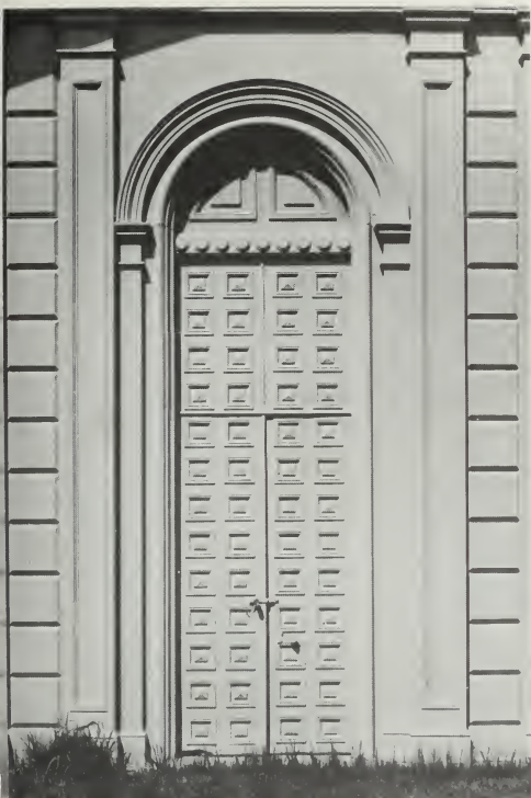
Figure 72. Cast-iron Personnel Door (south elevation) and Girder-Column Detail (interior), Watervliet Arsenal, New York, 1859; Daniel D. Badger's Architectural Iron Works of New York City. (a) This military storehouse is the most nearly all-iron building in the United States: the walls, window frames, doors, and columns are all cast iron, and the roof trusses are wrought iron. Built as a "fireproof" warehouse for ammunition storage, this classical Greek and Roman building was cast in sections at Badger's foundry and shipped by barge up the Hudson River to be assembled on the foundation in less than three months. (b) The detail shows a cast- and wrought-iron girder connected to a cast-iron column. The cast-iron part of the girder, the top three-quarters, is perforated to reduce the weight of the load and slightly arched to take compressive stresses. The wrought-iron part is at the bottom of the girder to take tensile stresses. (Jack E. Boucher, NAER)
