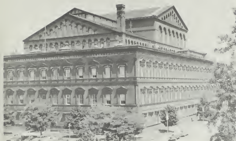
Figure 10. "Tinplate" Roofing, Old Pension Building, Fifth and G Streets, NW, Washington, DC, 1883; Montgomery C. Meigs, engineer. (a) The building consists of offices around the perimeter of a large court. The roof over the offices has a very low pitch and is covered with flat-seam tinplate, while the steep-pitched roofs over the court have batten tinplate roofs. (b) Flat seam tinplate roofing was used on low-pitched roofs because the edges of the plates could be interlocked and soldered together to provide a continuous waterproof covering. Stamped on each plate of the Pension Building roof is "Holkingshee Forge Best Roofing, 40 lbs., Manion Process License." The metal is actually terneplate. Surviving examples of true tinplate iron or steel are rare. (c) The batten tinplate roofs over the central court were typical of steep-pitched roofing of tin and other materials. They can be seen at a distance and provide a strong design element to the building. (David W. Look)
