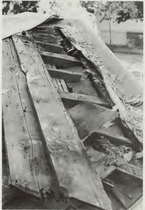
Figure 124. Successive Failure. If a metal architectural element such as a tinplate roof fails, more than just the tinplate may be destroyed. (a) Deterioration is evident in the original framing and roof sheathing of the Schuyler Mansion entrance wing in Albany, New York. The entrance wing was added to the building about 1817 and reroofed with tinplate sheets during the 19th century. The tinplate gutter liners eventually deteriorated and were replaced with copper during the 1930s. However, the tinplate roof remained and electrolysis occurred along the roof perimeter where the copper and tinplate were in contact. (b) Consequently, the tinplate was completely corroded away (as seen here) when the deteriorated roofing was removed. This resulted in major damage to the sheathing, framing, and masonry walls of the entrance. (John G. Waite)
