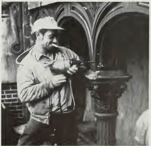
Figure 175. Drilling Holes. Originally, screw and bolt holes were cast into the pieces of iron for new ironwork; however, for the restoration of existing cast-iron facades which may have settled over the years, the holes are sometimes drilled into the replacement parts at the job site to insure correct alignment. (Walter Smalling, Jr.)
