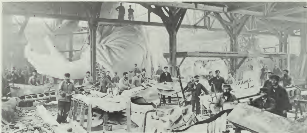
Figure 25. Copper Statue of Liberty, New York City Harbor, 1883-1886; Frederic Auguste Bartholdi, sculptor; Alexandre Gustave Eiffel, engineer. This photograph was taken in the metal shop in France where the sheet copper was fabricated. In the foreground, sheet metal workers are hammering the copper over wooden forms. The temporarily assembled arm and shoulder in the background, were later disassembled and shipped to the United States. Eiffel, who later designed the 984-foot Eiffel Tower of the Paris Exhibition of 1889, engineered the steel armature to support the statue built to the design of Bartholdi. (Rare Book Division, New York Public Library; Astor, Lenox and Tilden foundations)
