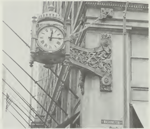
Figure 29. Bronze Clock, Marshall Field and Company Department Store Addition, corner of State and East Washington Streets, Chicago, Illinois, 1907; Graham, Anderson, Probst & White, architects. This huge bronze clock, weighing 7\frac{3}{4} tons and hanging 17 feet above the sidewalk, was designed by Pierce Anderson for the addition to Marshall Field's store. With a 46-inch face and a minute hand measuring 27 inches, the clock and its twin on another corner of the building can be seen for blocks. These magnificent works of art have become part of the city's landscape as a fourth generation of Chicagoans meet "under the clock." (Margot Gayle)
