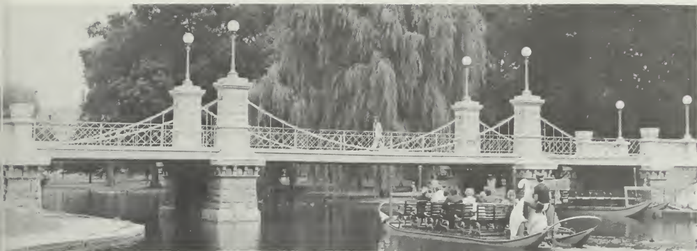
Figure 61. Suspension Bridge, Public Garden, Boston, Massachusetts, 1867; Elemens Herschel and William Preston, engineers. Popular among Bostonians, this small suspension bridge originally consisted of plank flooring hung from chains made of flat wrought-iron links. In 1921 the bridge's deteriorated wood was replaced with steel beams; the bridge was reinforced in 1975 with more steel and concrete. Although the deck has been replaced, the masonry piers and the chains hung between them are still largely original. (Carleton Knight, III)
