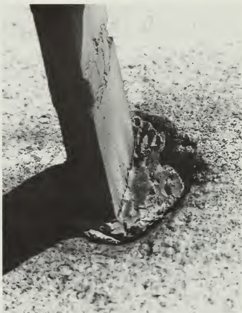
Figure 127. Lead Packing. At the U.S. Treasury Building in Washington, D.C., the iron fence is supported by stone posts. The iron rails are fitted into pockets in the stone. Water seeped into the pockets and the iron rusted, causing it to expand. Rust, plus freezing and thawing action, caused the stone to spall. To remedy the situation, the iron fences were removed; the ends of the rails were cleaned of rust and repainted; and the fence was re-erected with lead packing. This lead is soft enough to accommodate thermal expansion and contraction of the iron. It also waterproofs the ends of the bars. (John Myers)
