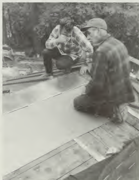
Figure 132. Repair and Replacement of Terneplate Roofing. (a) The ends of the original terneplate batten covers at Lindemould were badly corroded and could not be replated. (b) The unsalvageable sections were cut out and replaced with terne-coated stainless steel soldered in place. (c) The deteriorated terneplate valley was replaced with sheets of terne-coated stainless steel; the terne coating allowed the valley to be soldered to the original roofing plates. Although terne-coated stainless steel was a good choice, in theory, it proved to be a difficult material to work with in the field. (Correctly, the availability of thinner gauges and a more malleable stainless steel have improved the workability of this material.) (d) The original terneplate had rusted through completely in some areas, requiring reroofing. New sheets of terne-coated stainless steel, duplicating the pattern of the original terneplate, are being laid over rosin paper. (John G. Waite)
