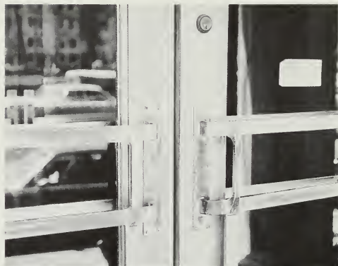
Figure 156. Oxidation of Monel. These exterior doors on the Headquarters of the United Mine Workers of America in Washington, D.C., have a greenish-brown patina of oxidation and an accumulation of dirt and fingerprints. Although the patina is protective, it is not attractive, and detracts from the overall appearance of the building. The push bars are brass with chrome plating which has worn through. To restore the doors to their original appearance, they should be cleaned and polished; and the push bars should be removed, cleaned, polished, replated, and reinstalled. (David W. Look)
