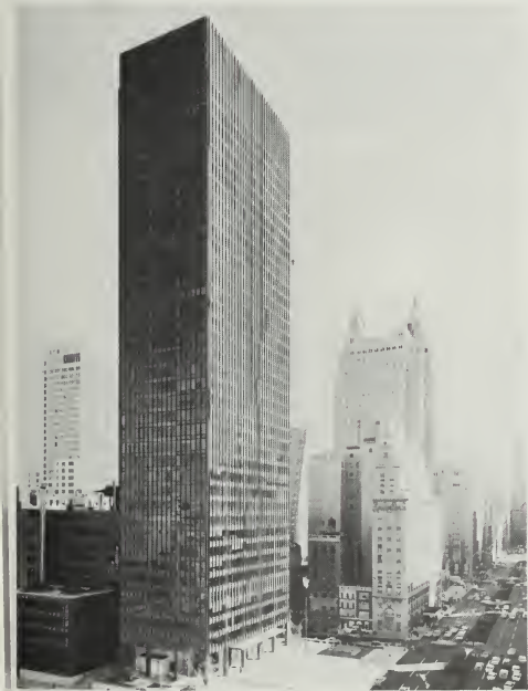
Figure 34. “Bronze” Curtain Wall, Seagram Building, 375 Park Avenue, New York City, 1958; Ludwig Mies Van der Rohe, architect. The curtain wall consists of 4 1/2- by 6-inch extruded architectural “bronze” (really brass: 57% copper, 3% lead, and 40% zinc) I-beam mullions (2 1/2 inches larger than the largest bronze sections extruded to that time), Muntz metal spandrels (brass also: 60% copper and 40% zinc), and pink-gray, heat- and glare-resistant glass in story-high architectural bronze frames. The 26-foot-long architectural bronze I-beams were extruded rather than built up with welded plates to avoid waviness in the sections. The architectural bronze, which only resembles real bronze with a statuary brown patina in color, is regularly rubbed with oil to prevent the bronze from forming a natural green patina. (Ezra Stoller)
