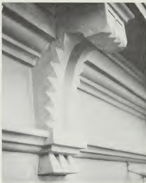
Figure 164. Exposure of Connections and Joints. After the Wilmington Opera House was sandblasted, screw and bolt holes were visible. A cast-iron bracket such as this one may be made of as many as 10 pieces. (Steven T. Baird, AIA)
