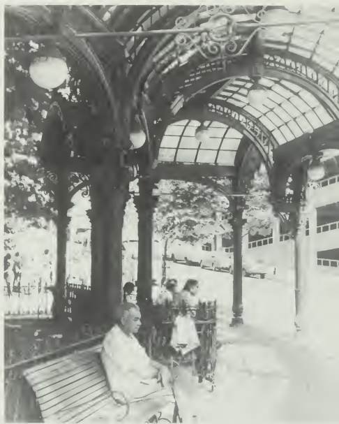
Figure 60. Iron and Glass Pergola, Trolley Station, Pioneer Square, Seattle, Washington, 1909. This station, which has become a symbol of the revival of the city's old commercial area, consists of glass panes held between ribs of wrought iron supported by cast-iron arches and columns, both of which are in compression. The wrought-iron tie rods (top of photo) take the outward thrust of the arches; thus, the rods are in tension. Iron members in tension had to be made of wrought iron because cast iron is suitable only for compressive loads. However, iron members in compression could be of either cast iron or wrought iron, whichever was more economical and convenient for the iron shop to fabricate. By the late 1960s, most of the glass in the pergola was broken and the iron was rusting. Preservationists, planners, and city officials worked together to rehabilitate Pioneer Square with the pergola as its centerpiece. Wooden patterns were carved from which sand molds were made to recast the lost and broken iron parts. With new lamps and fresh paint, the pergola was rededicated in 1973. (John Iochman, Seattle Office of Historic Preservation)
