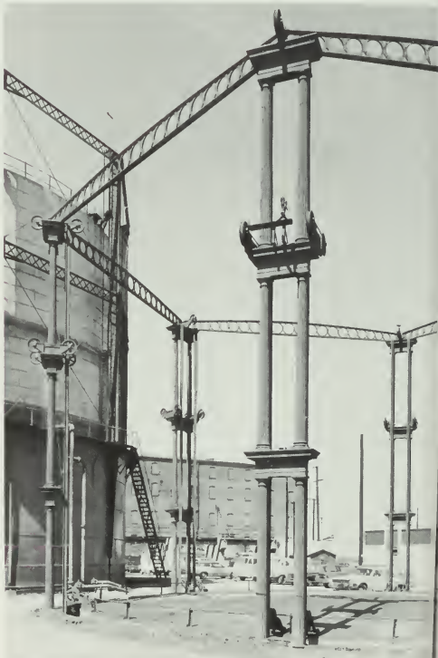
Figure 63. Cast-iron Gasholder, Petersburg Gaslight Company, Petersburg, Virginia, 1851–1852. The Greek Revival style gasholder has six pairs of slender Doric columns three tiers high which served as "guides" for the expandable tanks. Cast-iron horizontal members, which provided stability and carried only their own weight, are widest at the centers to resist bending. In this case the top of the beam is in compression and the bottom is in tension. To reduce weight, the beams were perforated with circles graduated in size toward the ends. (Jack E. Boucher, NAER)
