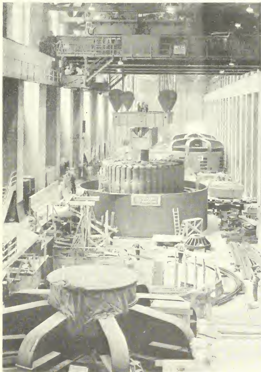
A 500-ton rotating field of one of the largest generators in the world is lowered into place by means of two traveling cranes, each with a capacity of 300 tons.
