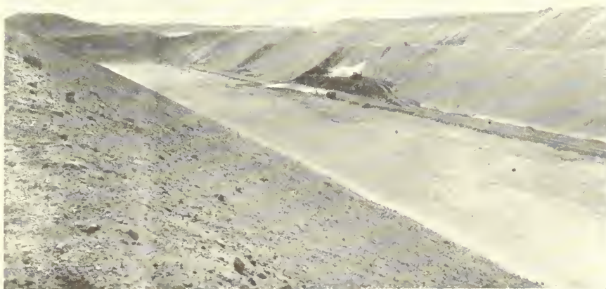
All-American Canal. Placing compacted lining.
