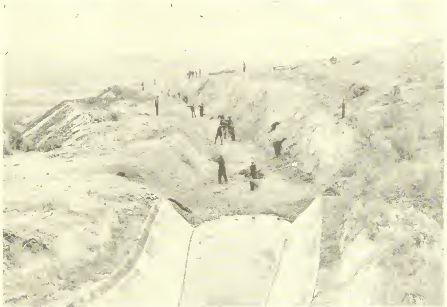
TOP: ENROLLEES LAYING RIPRAP—LOWER EMBANKMENT DEER FLAT RESERVOIR, BOISE PROJECT, IDAHO. BOTTOM: C. C. C. CREW AT CHANNEL OUTLET, CLEANING AND SLOPING STANFIELD CANAL, STANFIELD PROJECT, OREGON.
