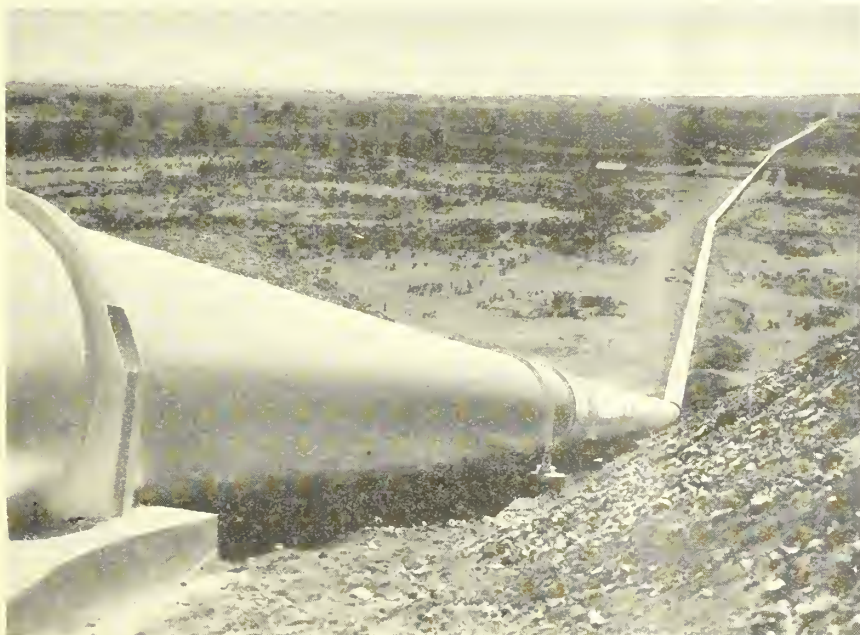
The Malheur River siphon of the Owyhee project, Oregon, the largest of its type on the continent, carries the main canal through the Malheur River Valley and over a low range of hills 4½ miles away. The siphon is being constructed of 80-inch pipe. It is approaching completion.
