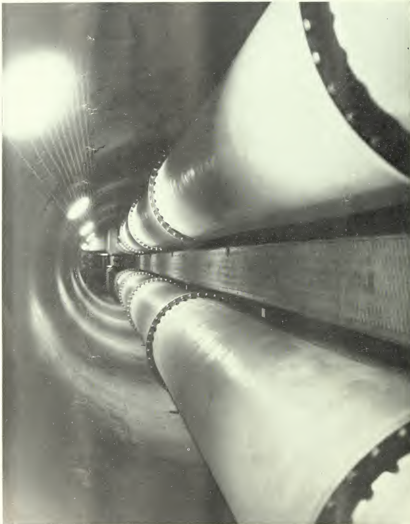
OUTLET WORKS OF THE NEWLY COMPLETED RYE PATCH DAM, NEVADA, THROUGH WHICH THE CONTROLLED WATERS OF THE HUMBOLDT RIVER ARE RELEASED FOR USE BY IRRIGATORS BELOW.
