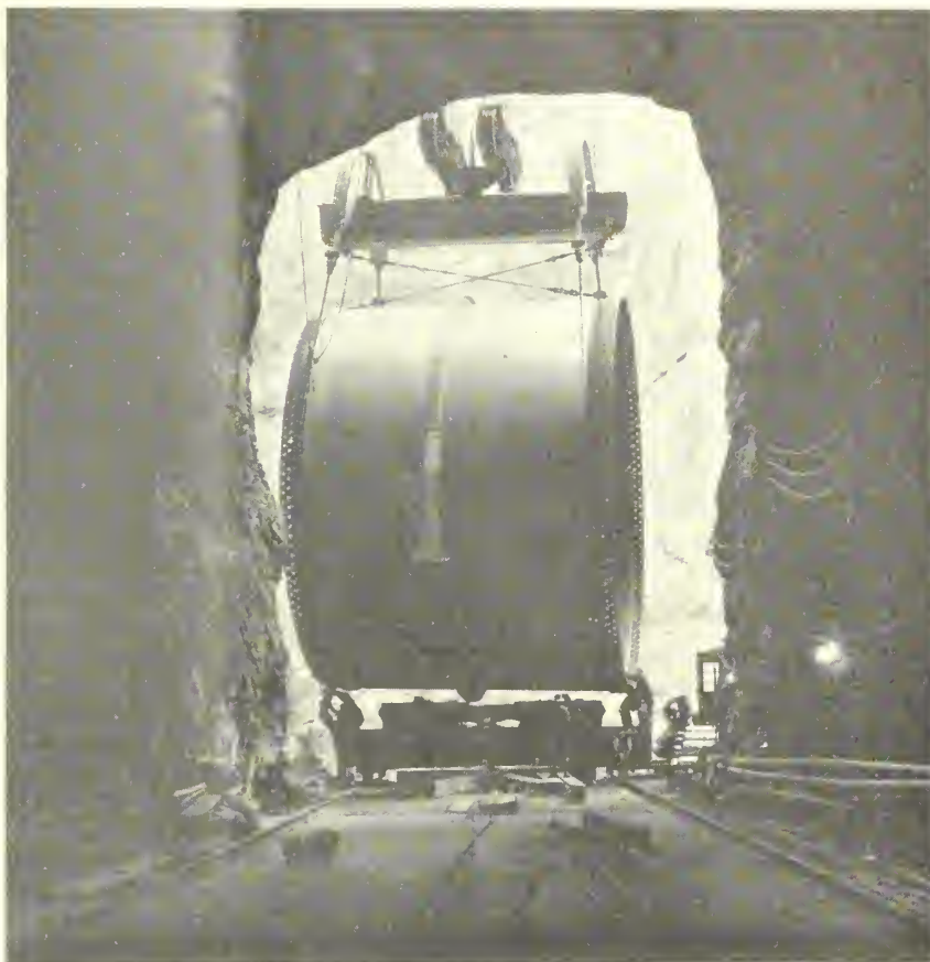
A 30-FOOT DIAMETER PIPE BEING LOWERED TO PENSTOCK TUNNEL ENTRANCE.
