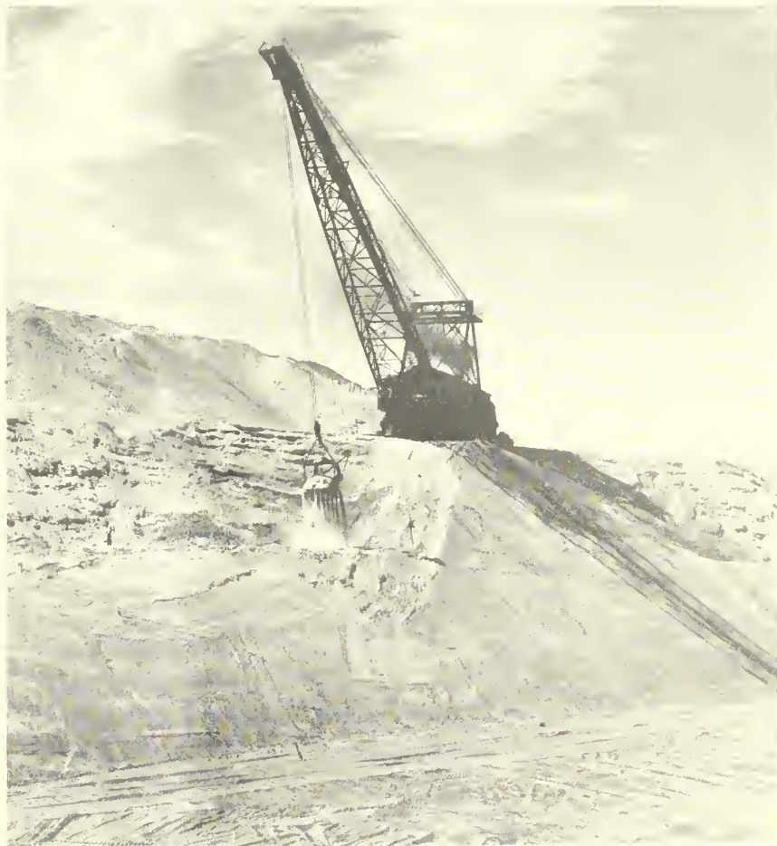
A DRAGLINE AT WORK IN A DEEP CUT ON THE ALL-AMERICAN CANAL WHERE THIS GREAT IRRIGATION DITCH PENETRATES THE DESERT DUNES ALONG THE INTERNATIONAL BOUNDARY WEST OF THE COLORADO RIVER.
