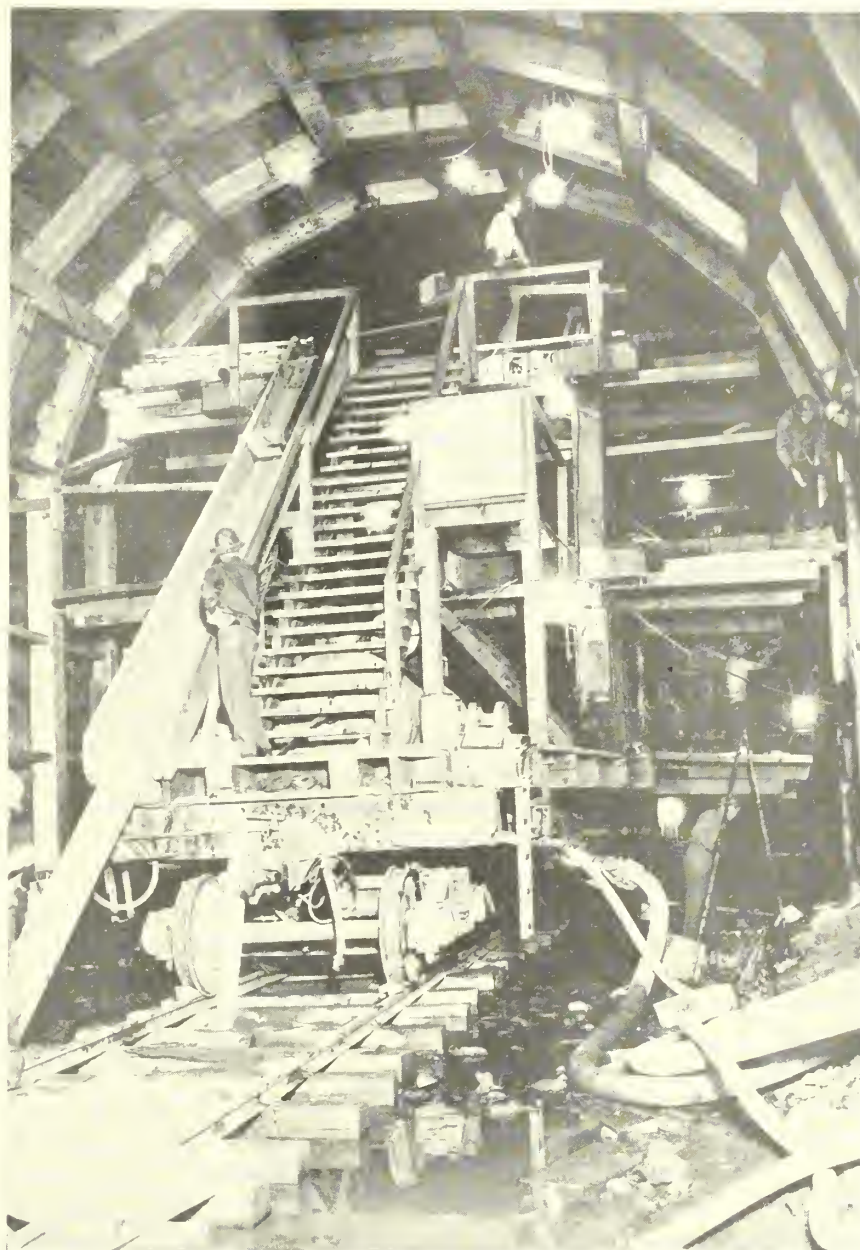
Timbering and drilling Tunnel No. 1.
