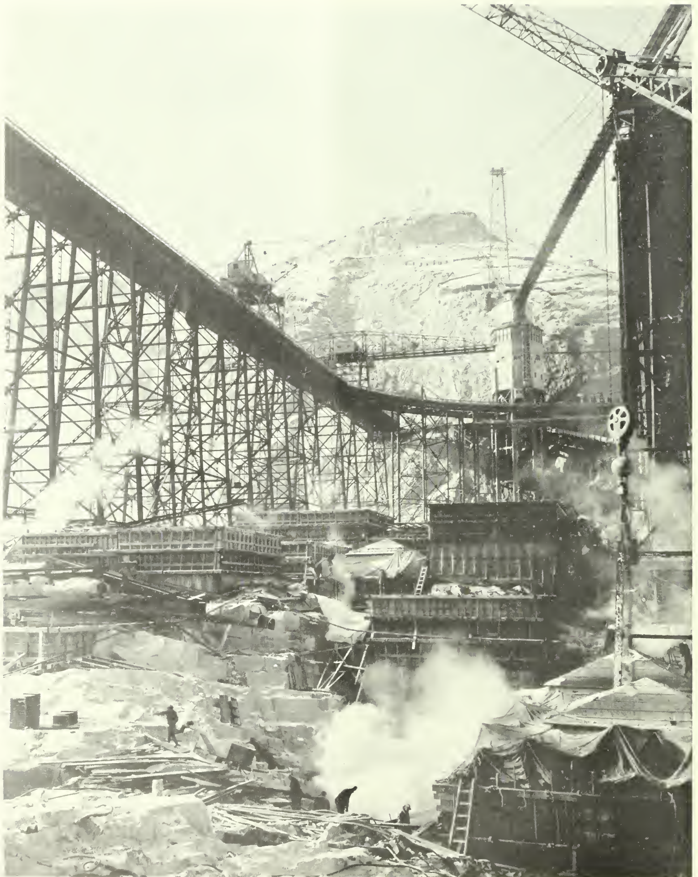
STEAM HEATING THE MOST RECENT POURS OF CONCRETE AT GRAND COULEE DAM DURING A COLD SNAP IN JANUARY
