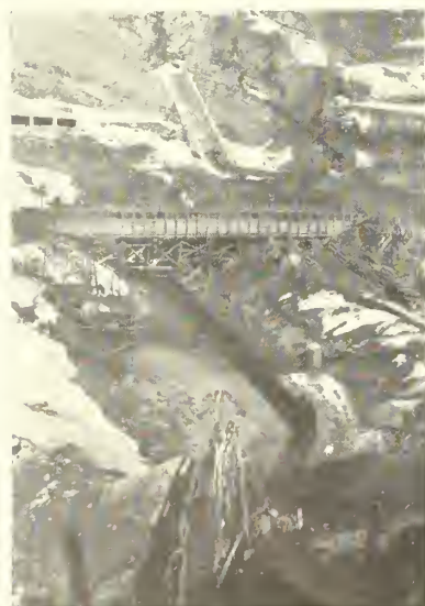
Pine View dam site, Ogden River project. Left: Looking into cut-off trench from road bridge at south abutment; center: Bridge being constructed at upper end of flume, also catwalk near Wheeler Creek; right: Trash rack spillway, and Eden Highway Tunnel portal.
