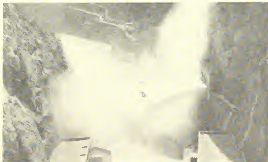
BOULDER CANYON PROJECT DISCHARGING VALVES AS VIEWED FROM CREST OF DAM
