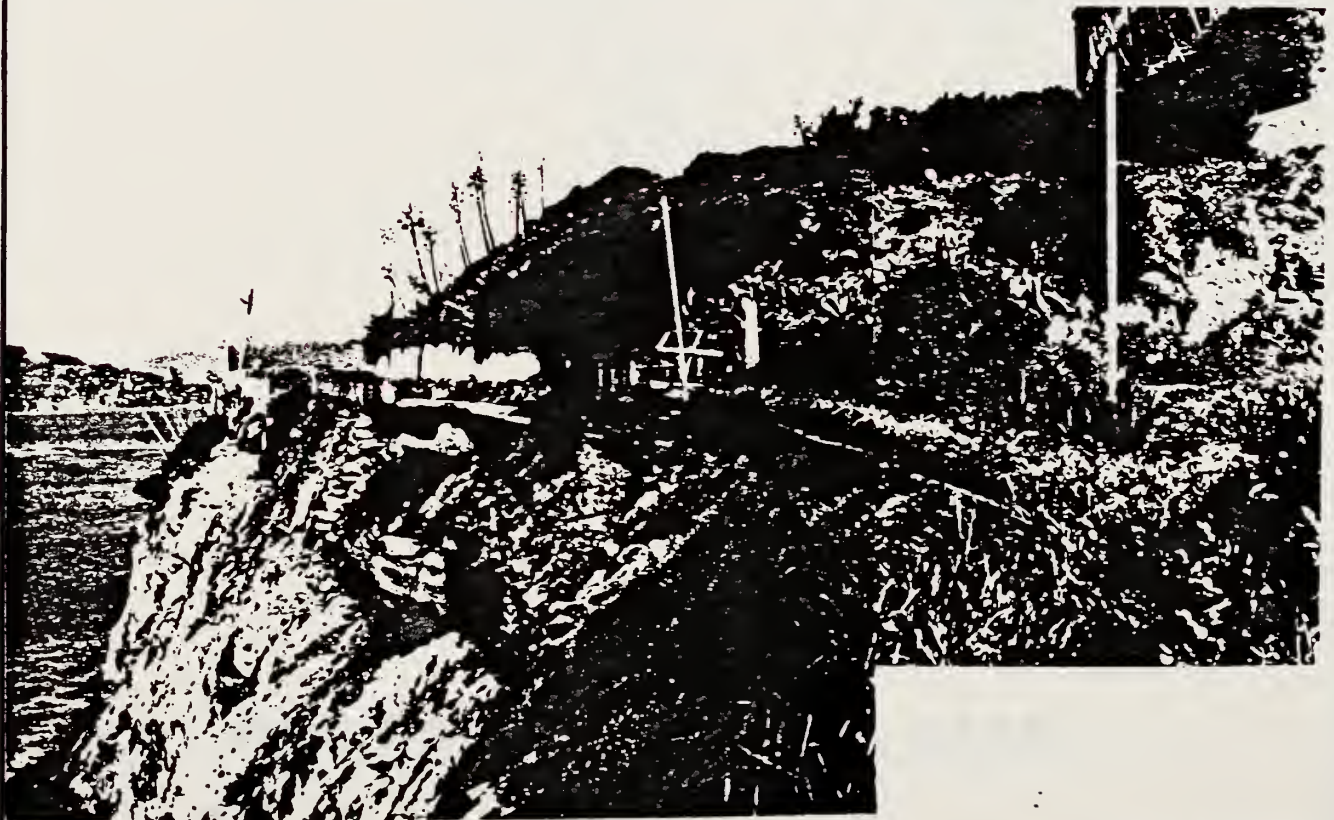
B. DAMAGE DUE TO UNDERMINING OF WEST ROAD
