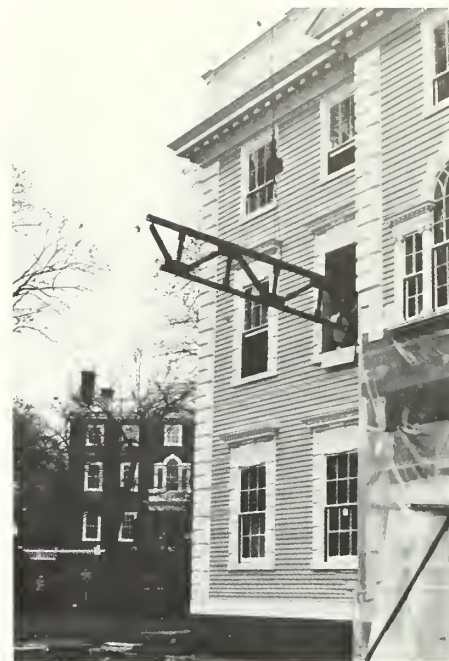
Figure 2. Because of the fire risks, open flame cutting and welding deserves careful attention both in the preparation of specifications and during the work. As much welding as possible should be done off site. For example, at the Nightingale-Brown House, several large trusses were assembled off site, then carefully hoisted through a window for installation. Photo: Irving B. Haynes and Associates.
