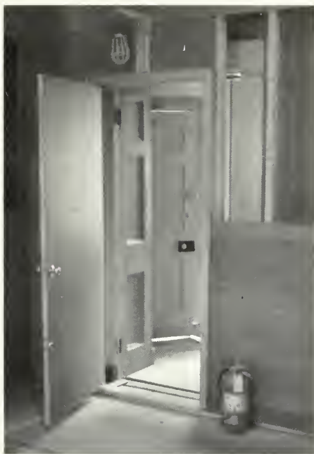
Figure 4. Temporary protection during construction can involve covering historic features, such as floors and walls, as well as using temporary doors to control the passage of workers and the inevitable dust and dirt. Prominently located fire extinguishers are mandatory. Photo: Lonnie Hovey, AIA, The Octagon.
