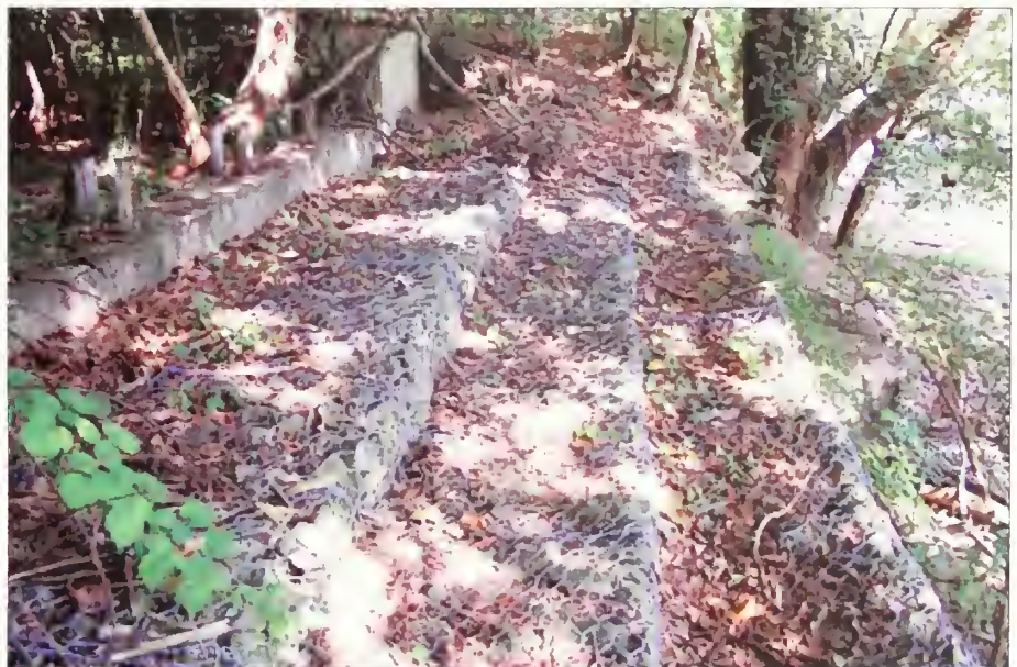
Figure 3.35. Canalway: View of gabion baskets found along portions of the breached canal structure. These features are indicative of 20th century repairs to the canal, used for electrical power generation until 1991. Non-contributing. OCLP, July, 2009.
