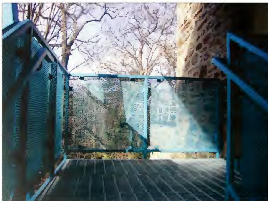
Figure 4.40. To reduce maintenance and increase longevity, metal can be utilized for steps and walkways and even handrails. In this example, the metal structure has also been painted blue. Other colors are also available. Hendrickmfg.com website.
