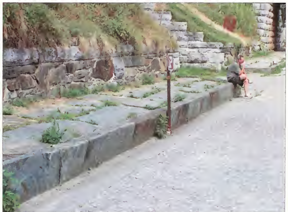
Figure 3.2. Lower Armory Grounds: Flagstone sidewalk at northern edge of Potomac Street with bluestone and granite curbing. Extant c. 1900. Contributing. OCLP, July, 2009.
