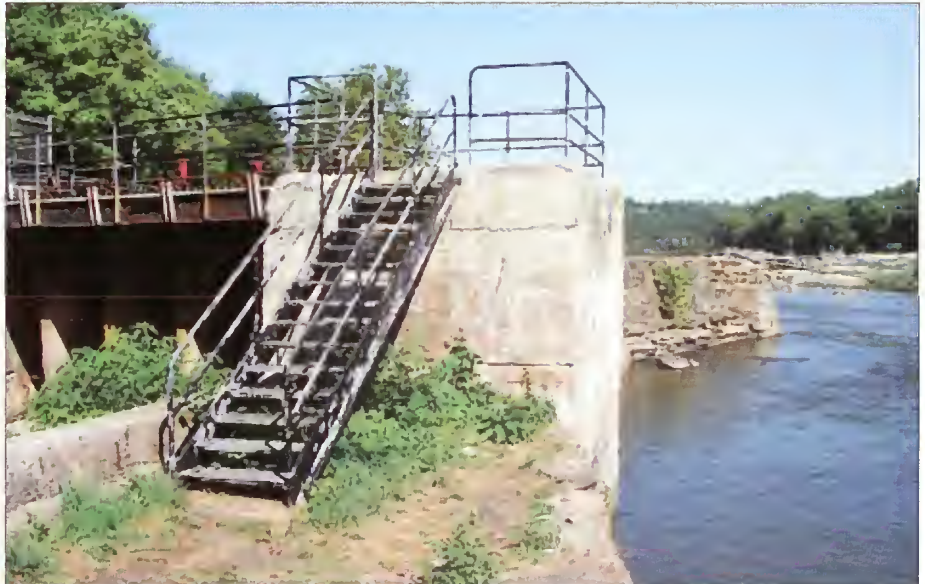
Figure 3.29. Canalway: View of contemporary 20th century canal intake structure at former Armory dam on the Potomac River. This modern construction incorporates foundation elements of early 19th century construction. Contributing. OCLP, July, 2009.
