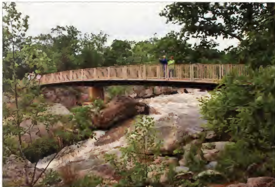
Figure 4.31. View of removable handrails installed on a bridge constructed at Olmsted Island at Chesapeake & Ohio Canal National Park. www.panoramio.com/photos/original/22366336.jpg
