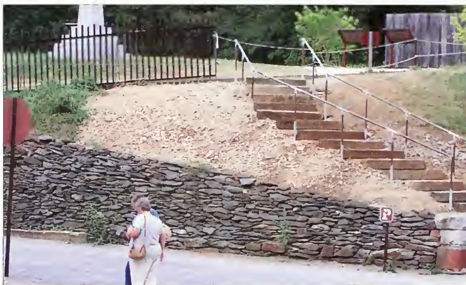
Figure 3.12. Lower Armory Grounds: View of battered dry-laid rubble retaining wall along 1892 embankment on Potomac Street. Extant c. 1900. Contributing. Above the wall, new timber steps have recently been installed. OCLP, July, 2009.
