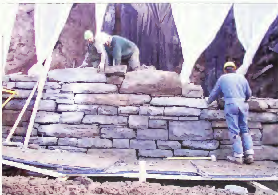
Figure 4.61. An example of dry stone wall repair work on a retaining wall at Roebling Aqueduct in Minisink, New York. http://www.drystone.org/gallery/album27/Roebling_NY_11_13_nr_023 .
