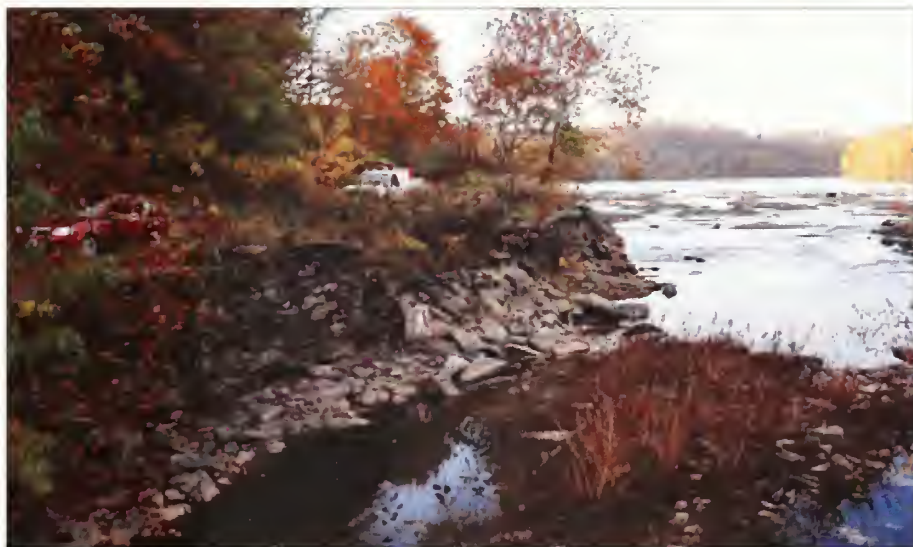
Figure 4.60. View of the retaining wall at the former Armory dam area. Severe damage has occurred in several places along this wall. OCLP, November, 2008.
