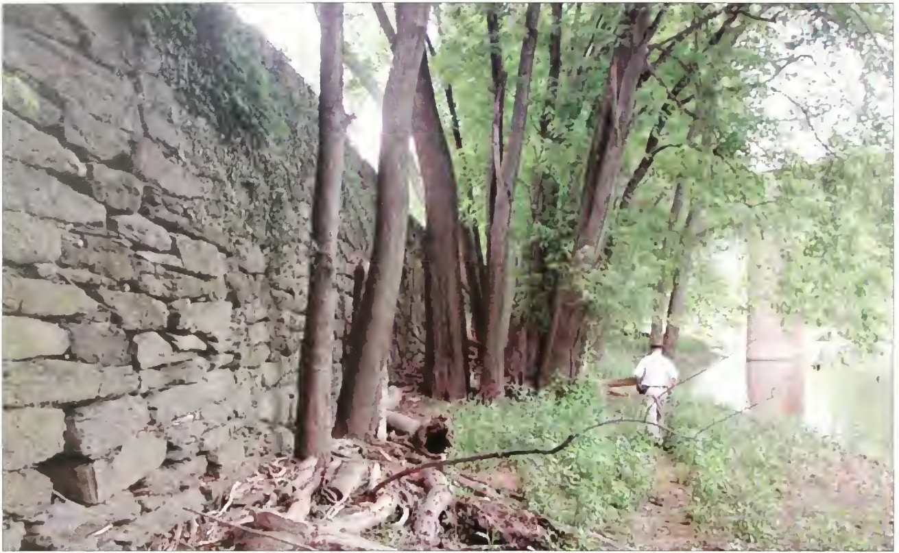
Figure 4.47. View of river wall along the edge of the Musket Factory grounds. Removing the trees would enhance the visibility of the feature and prevent structural damage. M. Joseph, June, 2006.
