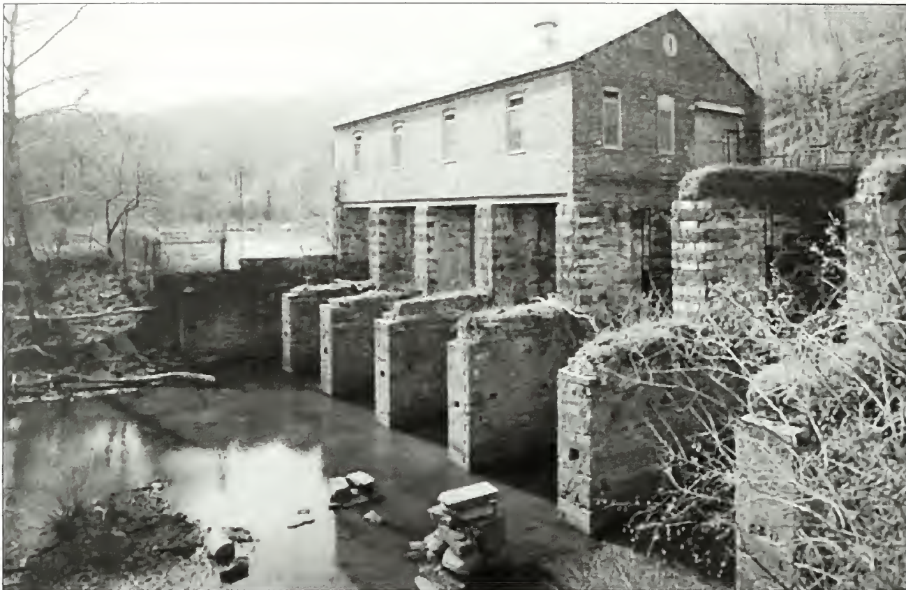
Figure 1.32. View of Harpers Ferry Power Plant constructed on top of foundations of former pulp mill which was on top of the original Armory Rolling Mill. HAER WV-61-2.
