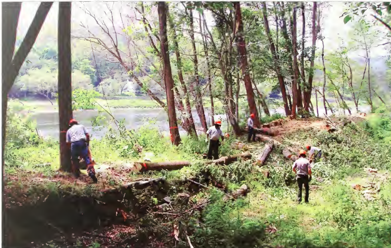
Figure 4.35. Tree cutting along the D&H Canal in New York, intending to protect the remnant structural features of the canal. A similar tree removal process is recommended for the Armory riverfront. OCLP, 2008.
