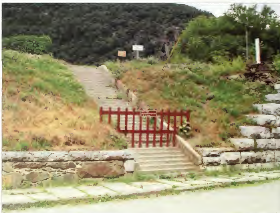
Figure 2.13. View of concrete steps at Lower Armory Grounds with flagstone sidewalk and stone retaining wall in foreground. Access is currently closed. OCLP, June, 2006.
