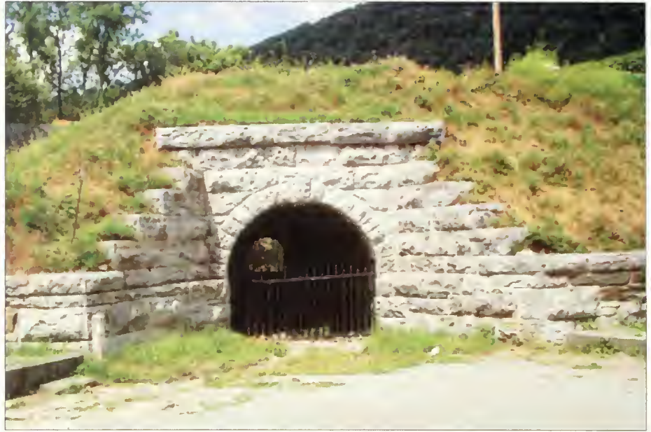
Figure 2.25. View of culvert built in 1892, along with the embankment, in order to mitigate drainage problems when the water level rose. This portion of the embankment was originally reinforced with stone. OCLP, June, 2006.
