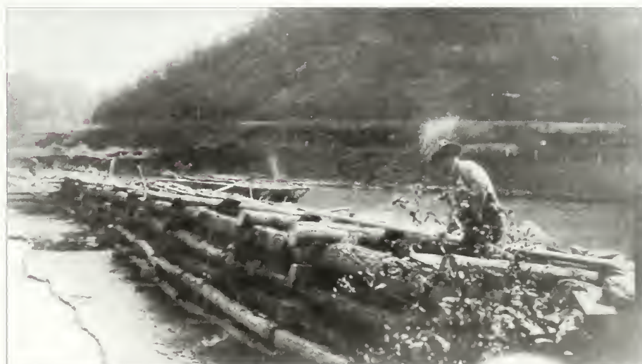
Figure 1.31. View, taken prior to 1936, shows work being done on the former Armory dam in the Potomac River. Referred to as a crib dam, the structure is built of heavy timbers in the manner of a log house and the interior is filled with earth or rubble. The heavy crib structure supported the dam's face and the weight of the water. Photo from Thomas Savery Collection 72.369, Hagley Museum and Archive.
