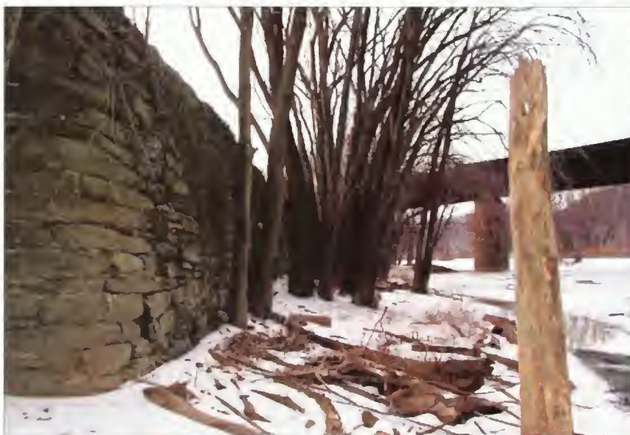
Figure 2.3. Stone retaining wall along the Potomac River at Lower Armory grounds. The change in grade is roughly twelve to fifteen feet. OCLP, February, 2007.
