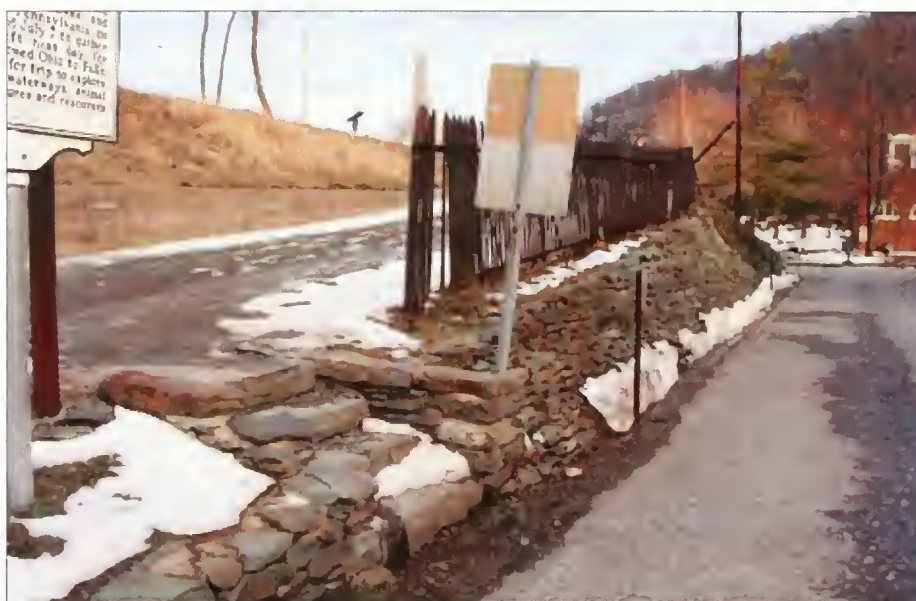
Figure 2.17. Gravel access road at the 1892 embankment. The lower portion of the embankment is retained by a stone wall while the upper portion is retained by a concrete wall and grassy slope. OCLP, February, 2007.
