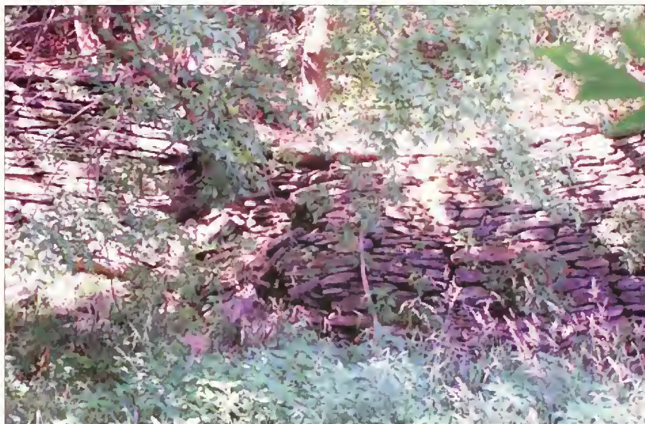
Figure 4.59. An example of erosion and deterioration of the Armory canal. The growth of woody vegetation over the years has taken a toll on several portions of the canal. OCLP, July, 2009.
