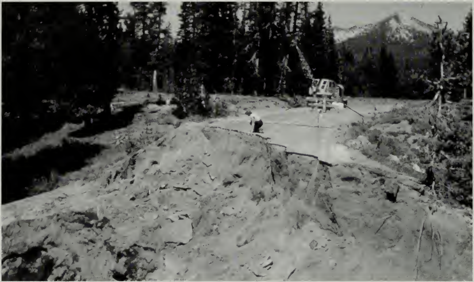
Cross drainage failure on the East Rim Drive, 1950s. CLNPMAC , 8898.
