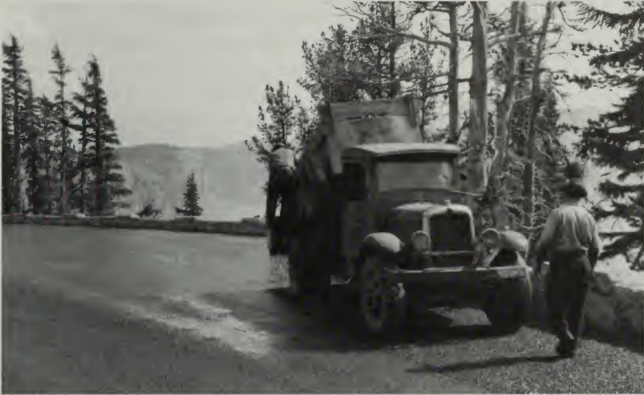
Crew paving with half-inch minus top coat, 1938. W. C. Struble, Bureau of Public Roads; courtesy of Wade Johnston, FHWA.
