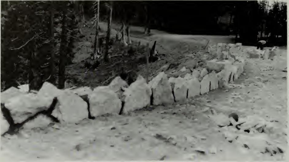
Building masonry guardrail in segment 7-B, 1934. Doerner, NARA, RG 79, SB
