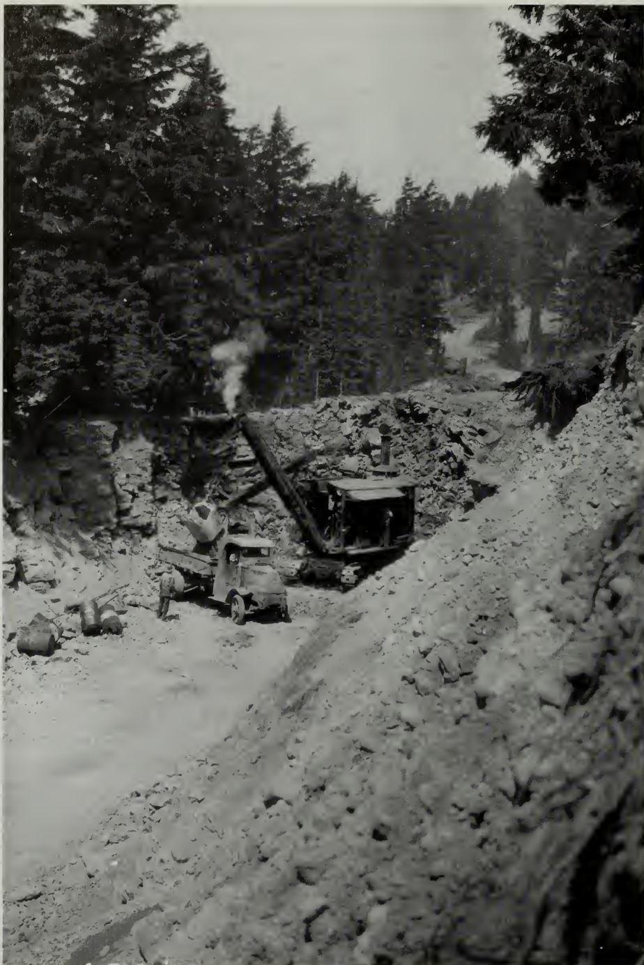
Steam shovel excavating at road station 130, segment 7-A, in 1932. Sargent, BPR-FHWA.
