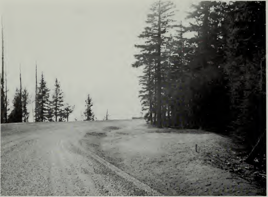
An example of a parking area unintentionally created by a low-angle cut. Lange, CLNPMAC.
