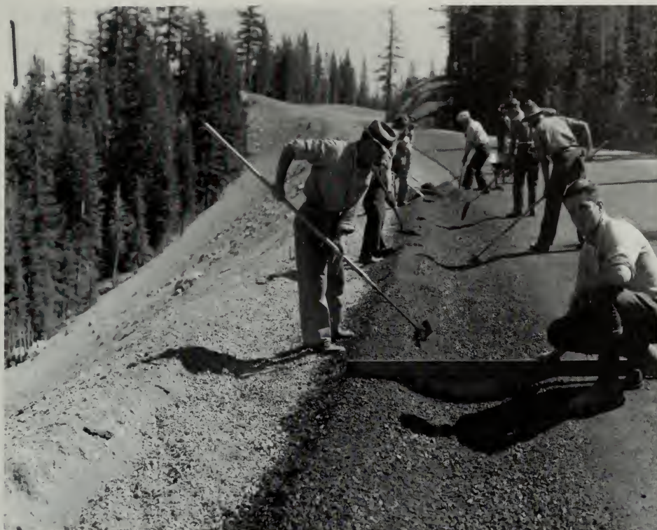
Laying and shaping a gutter section. Note template in foreground. Struble, BPR-FHWA.
