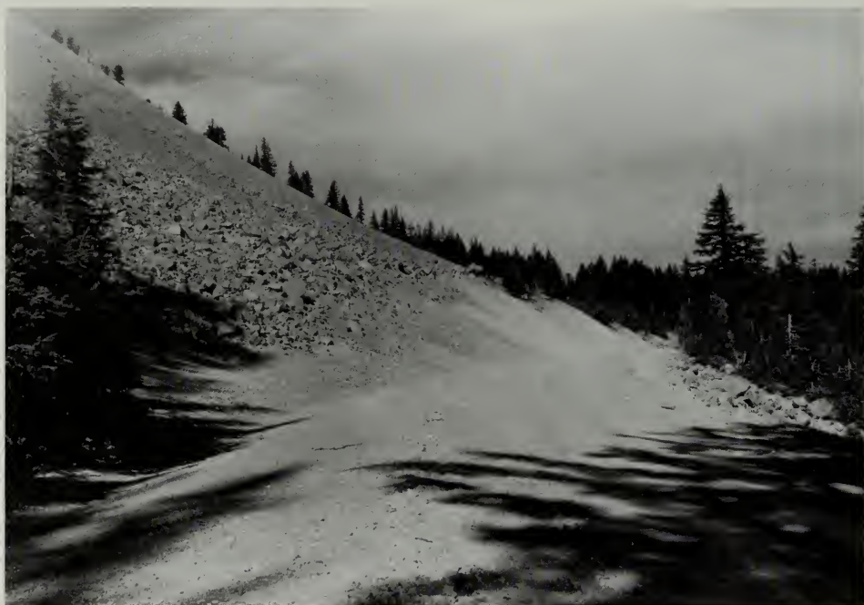
Bank sloping through a slide below Applegate Peak in segment 7-E1, 1937. Warping at road margin to the right. Lange, NARA, RG 79, SB.
