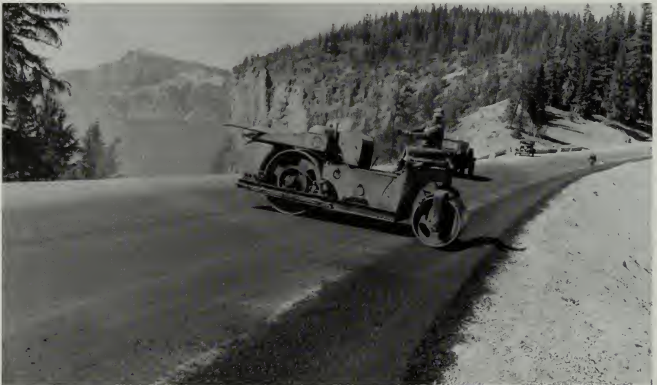
Rolling a gutter section in road segment 7-B. Struble, BPR-FHWA.
