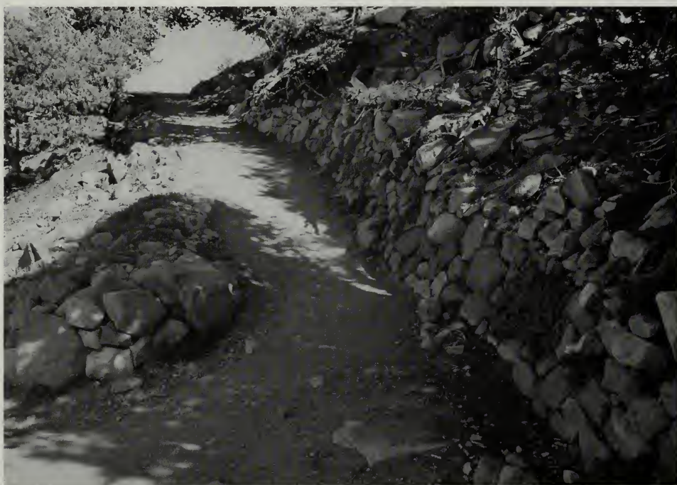
Dry laid retaining wall on the Watchman Trail. Steve Mark.
