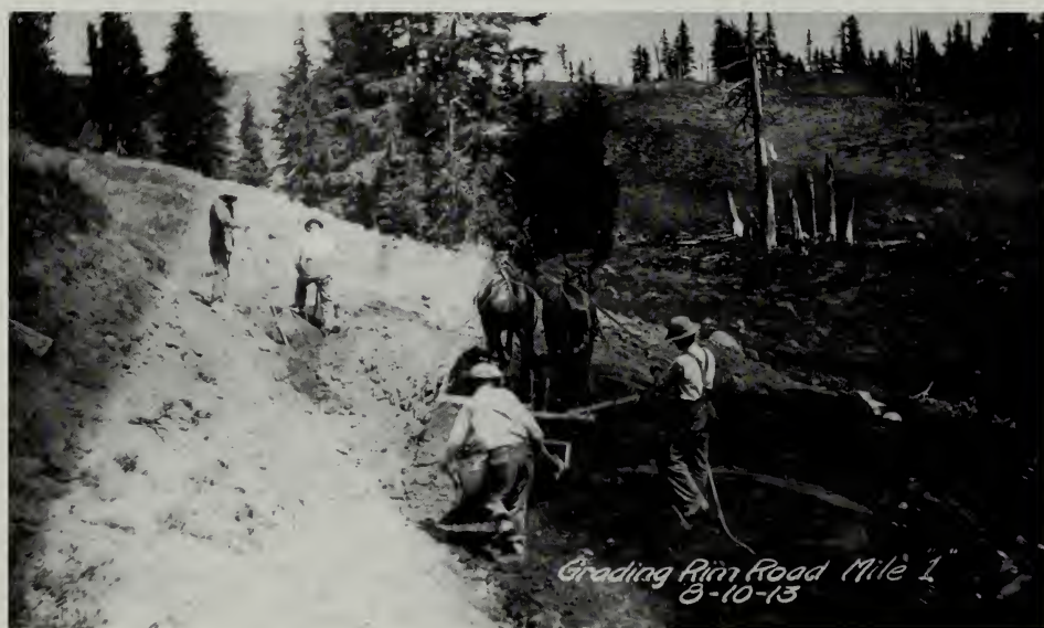
Grading with a team, note the use of a plow. National Archives and Records Administration (NARA), Record Group (RG77), Washington, DC.
