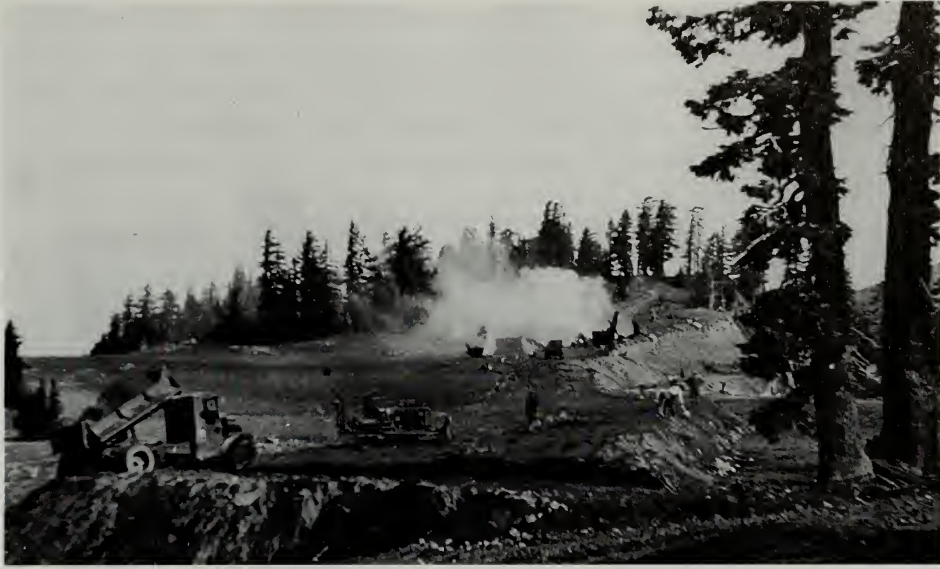
Rough grading along segment 7-A during the summer of 1932. Sager, NARA, RG 79, SB.
