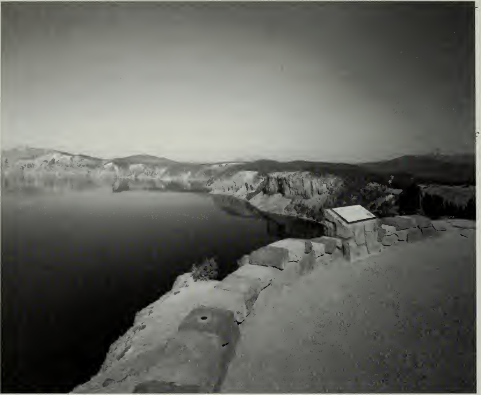
Section of parapet wall at Skell Head with the wayside exhibit mounted on a stone masonry base. Jet Lowe, HAER.
