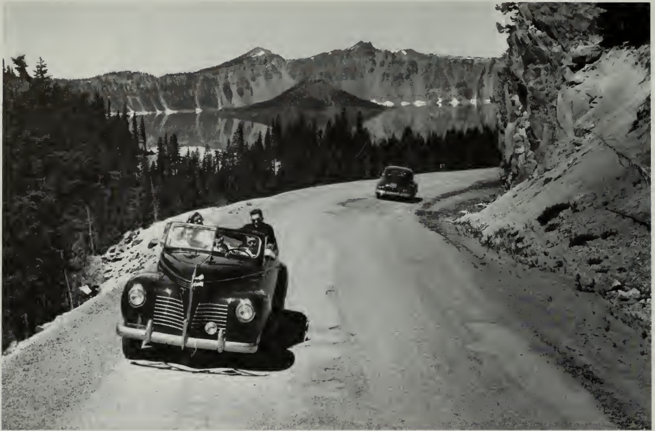
Oregon State Highway Commission publicity photo taken near Anderson Point, late 1940s. Note that the road surface is not paved but instead treated with oil. Oregon State Archives.
