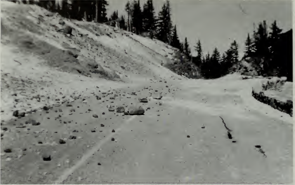
Raveling on the road cut above Cleetwood Cove. CLNPMAC 8898 .
