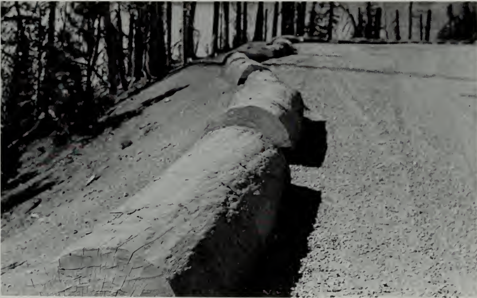
Log guardrail near road station 1045 in 1936. Lange, NARA, RG 79, SB.
