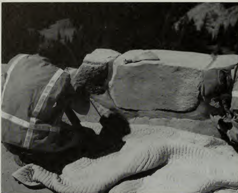
Repairing a portion of a masonry guardrail on west Rim Drive, 2002. Jerry Watson.
