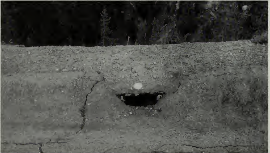
Opening for a drop inlet. Jerry Watson
