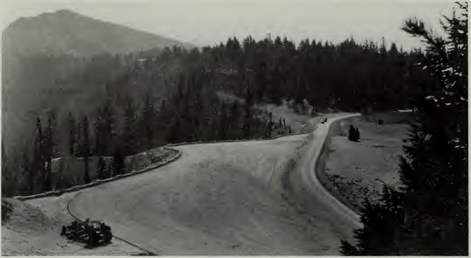
Masonry guardrail delineating the Discovery Point parking area, 1935. Lange, NARA, RG 79, SB.
