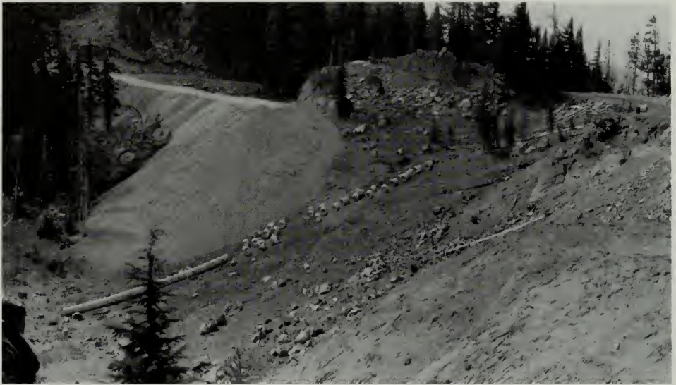
Partially assembled concrete pipe culvert near toe of fill, road segment 7-B, 1934. Doerner, NARA, RG 79, SB.
