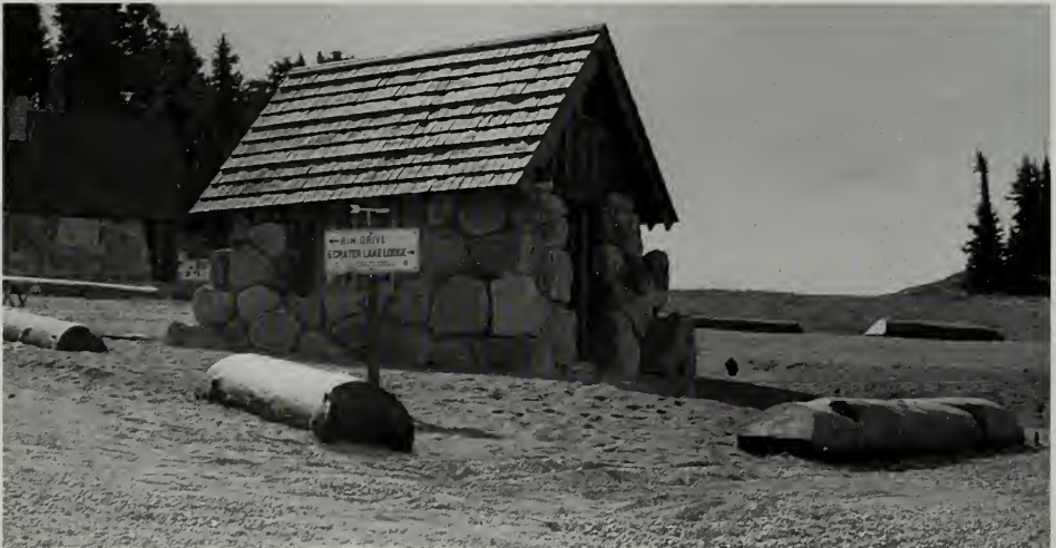
Treated logs used to define the road wye at the North Junction, 1936. Lange, NARA, RG 79, SB.
