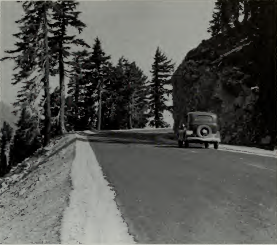
Bituminous mat at road station 260 in 1935. Lange, NARA, RG 79, SB.
