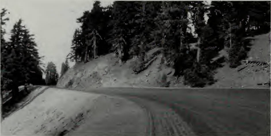
View of the adjacent road section showing finished treatment with seal coat given to both the ditch and travel lanes. Lange, NARA, RG79, SB.
