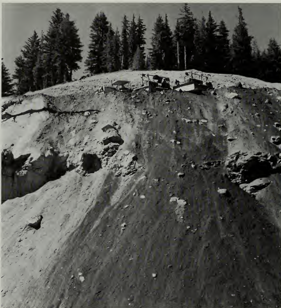
Scaling on Anderson Point, 1952. CLNPMAC , 8885-4379.
