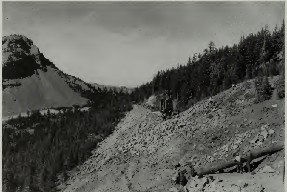
Culvert installation and rough grading on road segment 7-D (Sun Grade), 1937. Struble, BPR-FHWA.
