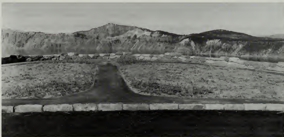
Detail of a portion of Skell Head parking overlook showing completed bituminous mat and sidewalks, 1938. Struble, BPR-FHWA.
