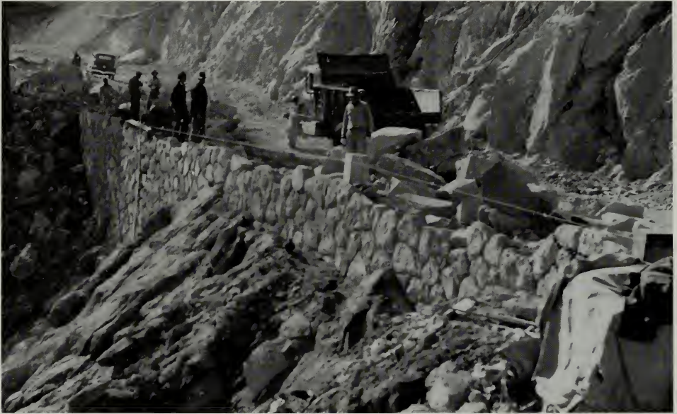
Building the retaining wall and guardrail at Scott Bluffs, 1934. Doerner, NARA, RG 79, SB.
