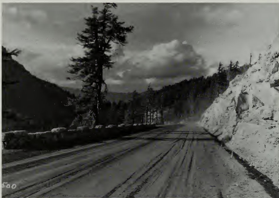
Graded road and masonry guardrail on Sun Grade, road segment 7-D, 1938. Note the “gutter line” at right. Struble, BPR-FHWA.
