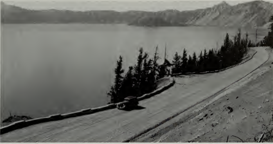
Guardrail lining Rim Drive near road station 1043 (Cleetwood Cove vicinity) during the surfacing phase of building segment 7-B, 1936. Lange, NARA, RG 79, SB.
