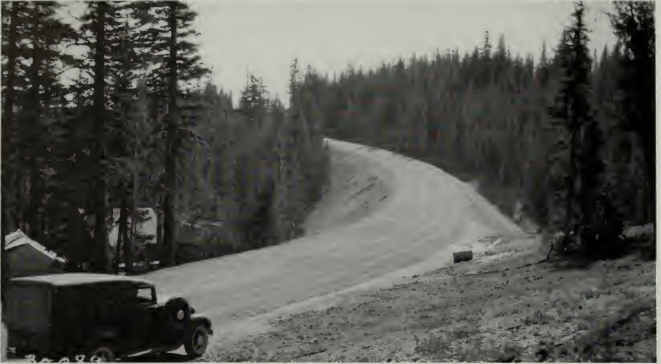
Heavy fill at Wineglass prior to surfacing. Contractor's camp at left. Struble, BPR-FHWA.
