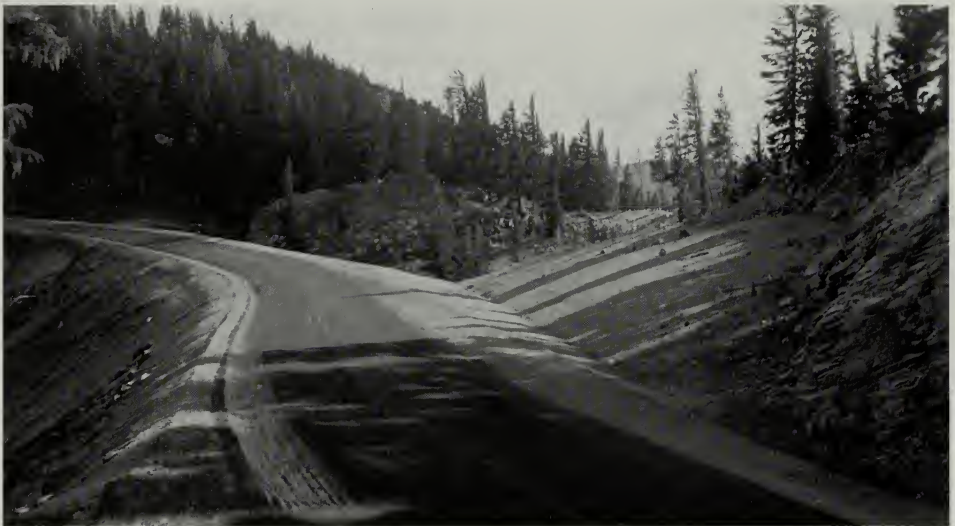
Old road obliteration through use of bank sloping along the northern part of Rim Drive. Lange photo pair, CLNPMAC.
