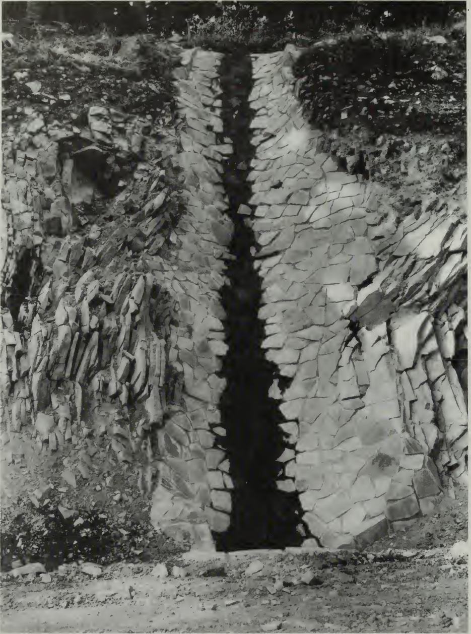
A “spillway” built in segment 7-D2, 1937. Lange NARA, RG 79, SB
