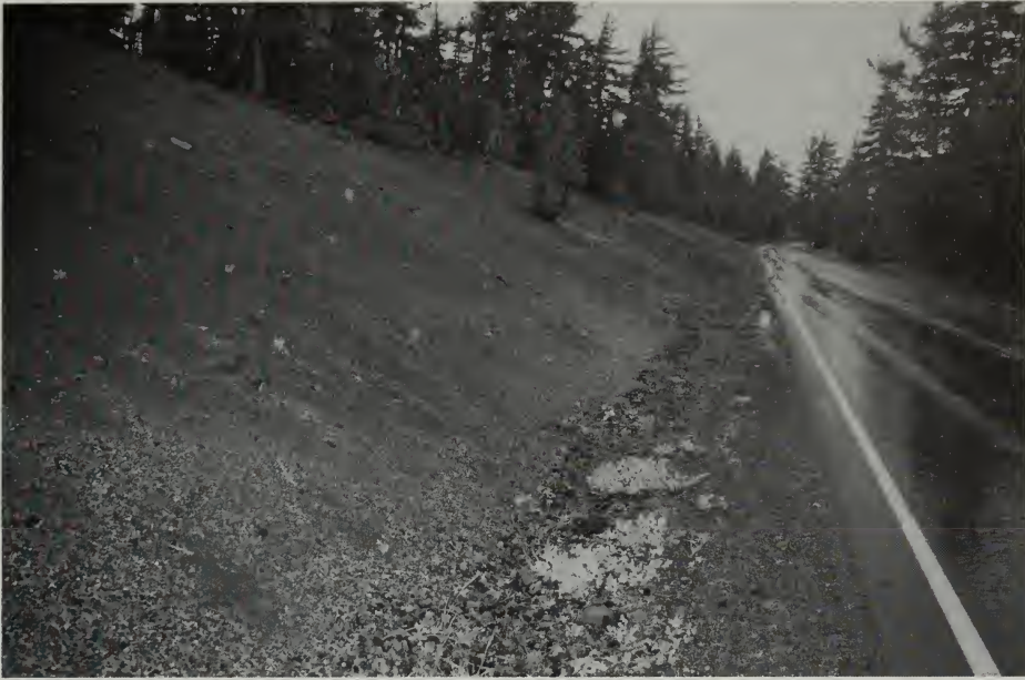
Typical section of Rim Drive showing a daylighted cut, road segment 7-B. Steve Mark.
