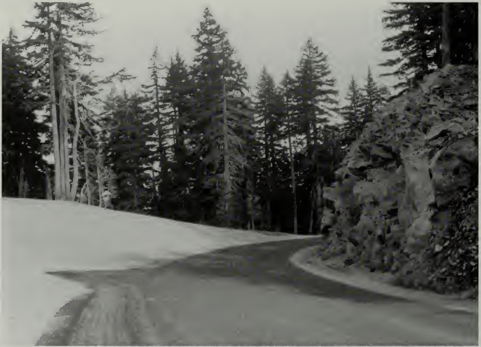
Termination of paved gutter into a catch basin at center left. Lange, NARA, RG 79, SB.
