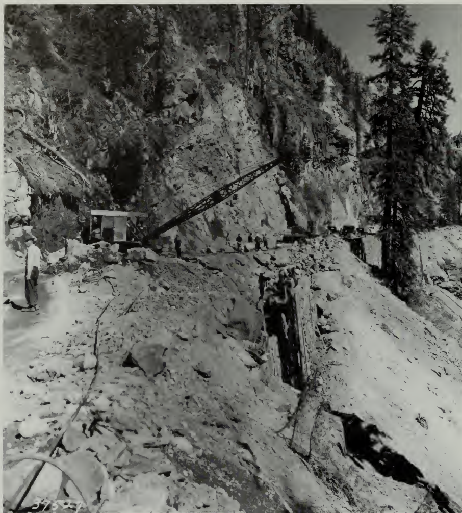
Building a retaining wall as part of grading Rim Drive on Dutton Cliff. Wendall C. Struble, Bureau of Public Roads; courtesy of Federal Highway Administration, Vancouver, Washington.
