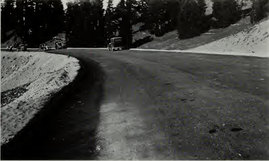
Section of ditch near the Diamond Lake Junction after an initial step in paving, the application of plant mix. Lange, CLNPMAC.
