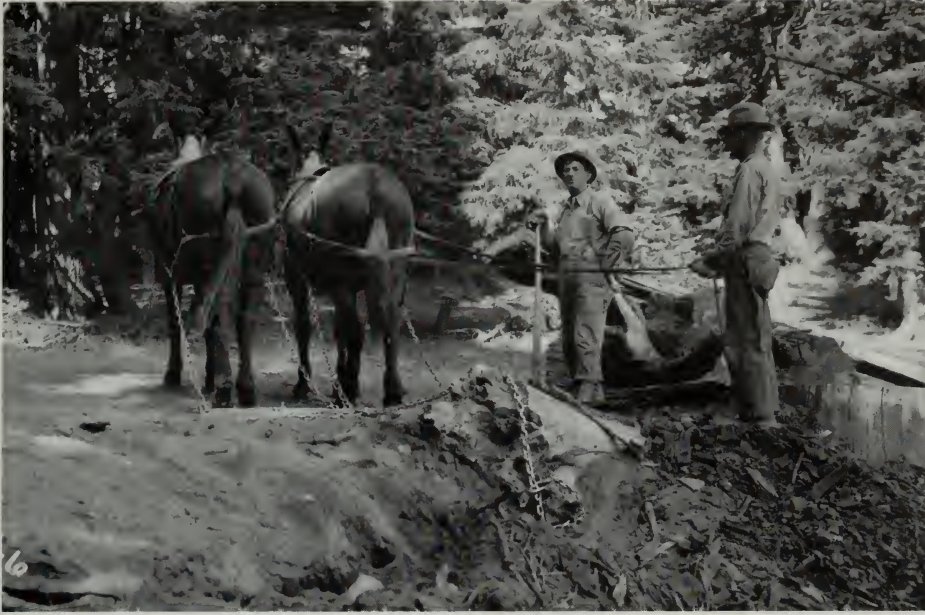
Team and hand labor method of grubbing road segment 7-B, 1933. Sargent, BPR-FHWA.
