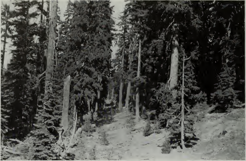
Old road obliteration through tree planting and placement of duff at road station 1140, 1935. Doerner, NARA, RG 79, SB.
