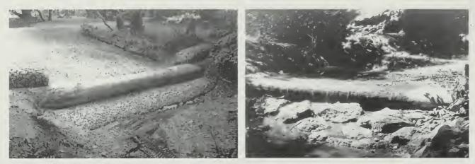
Figure 4.32 (left): Log check dam in Redwood Creek near the Emerson tree during construction, September 20, 1932. The log had a diameter of 36 inches. Courtesy Golden Gate National Recreation Area, Park Archives, box 35/5, Muir Woods Collection.
