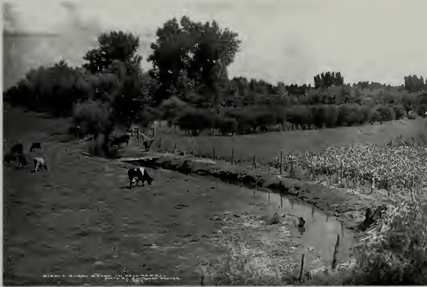
Figure 3.32: Historic photograph of an unlined, hand-dug irrigation ditch watering an orchard and pasture in the 1910s. Note the fence to exclude grazing cows from the low-headed orchard, CO (courtesy of Western History/ Genealogy Dept., Denver Public Library).
