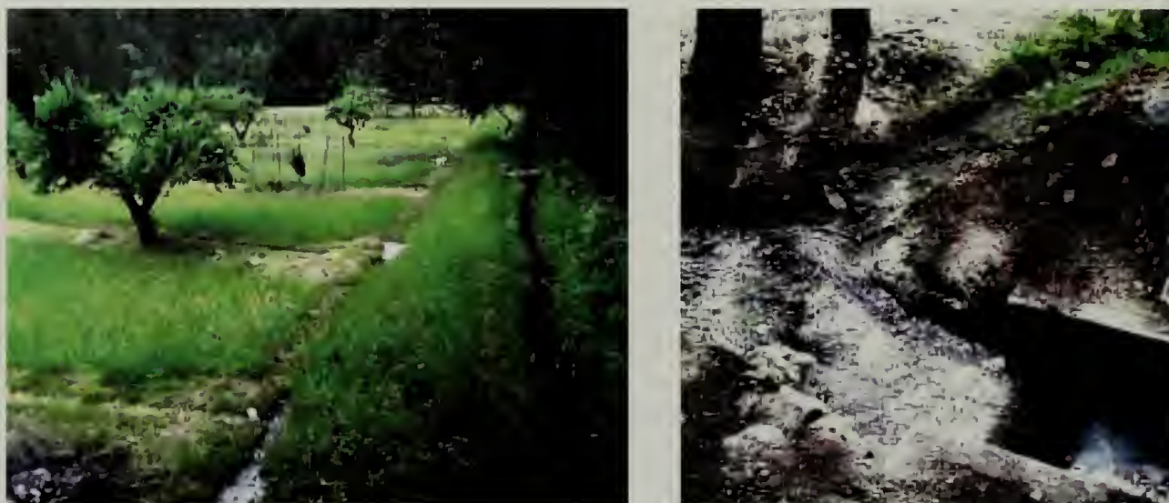
Figure 5.22: (above, left and right) Photographs of the historic irrigation system at the Buckner orchard in North Cascades National Park Service Complex, fed by a main ditch from a diversion dam on Rainbow Creek to supply a system of minor ditches or furrows (left) that line each row of apple trees. The system is controlled by concrete head gates (right) that divert water to specific ditches as needed, WA (S. Dolan, 1999).
