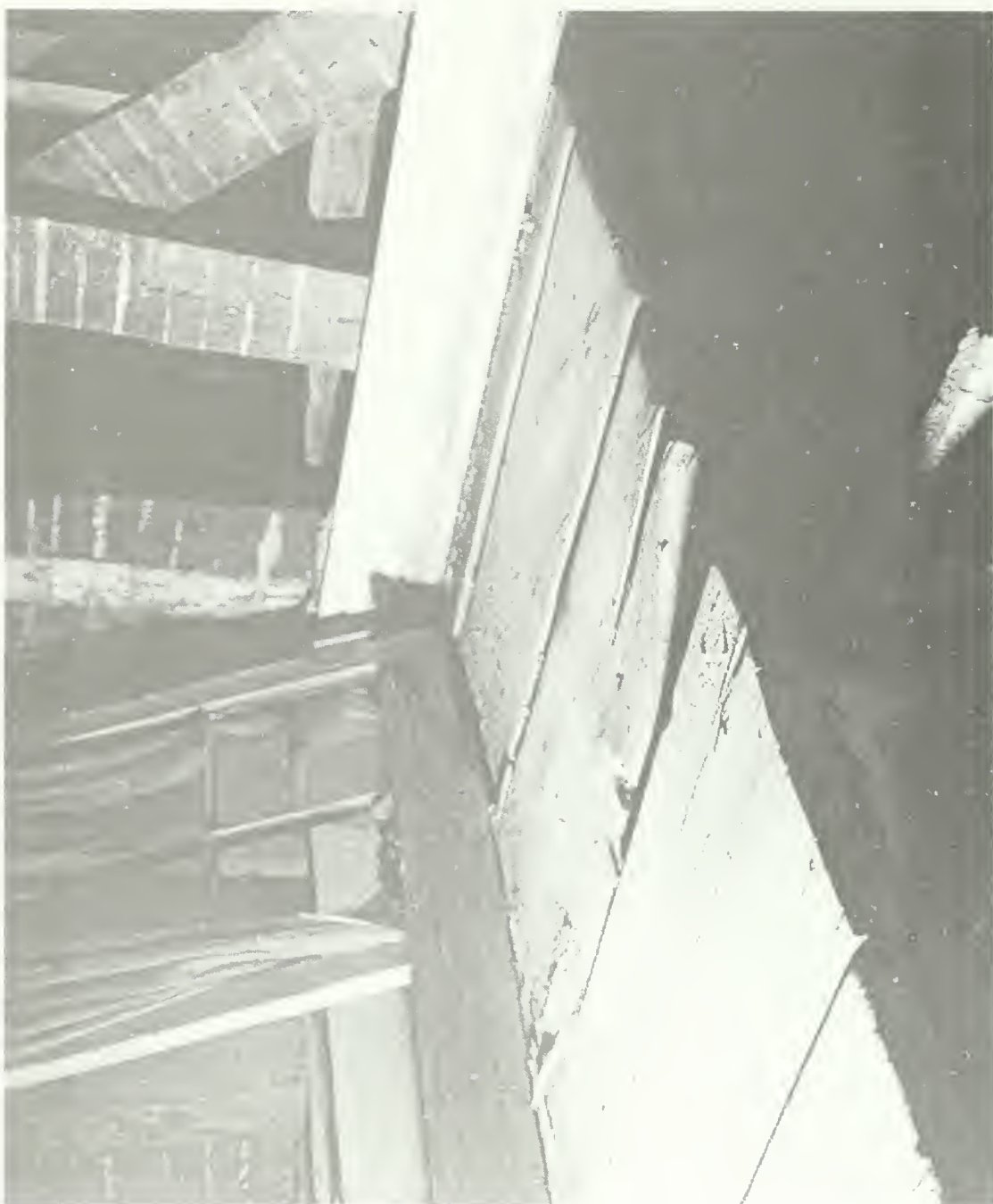
Figure 61. Schuyler House: Second story of kitchen wing after ca.-1815 lath and plaster removed; worn flooring in hall (Room 206) at location of ca.-1780 staircase landing (1958).
