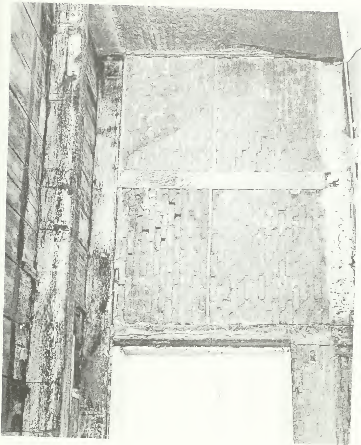
Figure 56. Schuyler House: First story of kitchen wing after ca.-1815 lath and plaster removed; north end of west wall in location of ca.-1780 storage room (1958). Window at left was originally a ca.-1780 exterior doorway.
