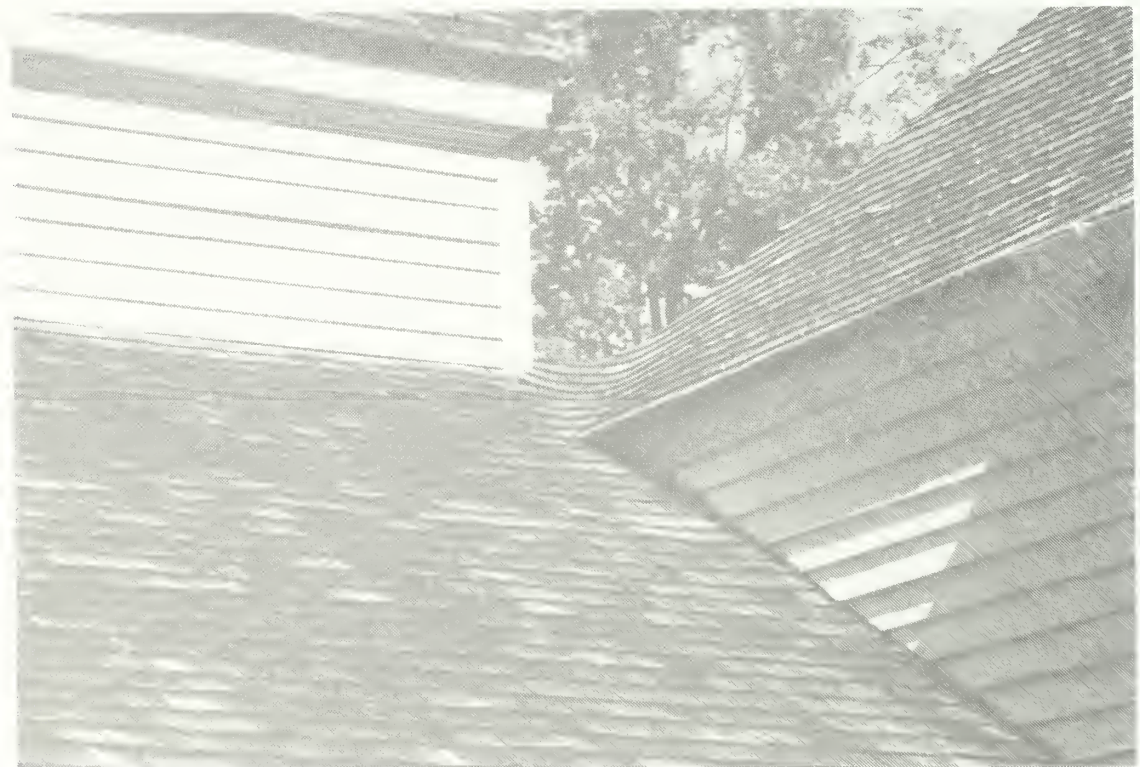
Figure 134. East elevation, cricket at junction of north-porch roof and kitchen-wing roof.
