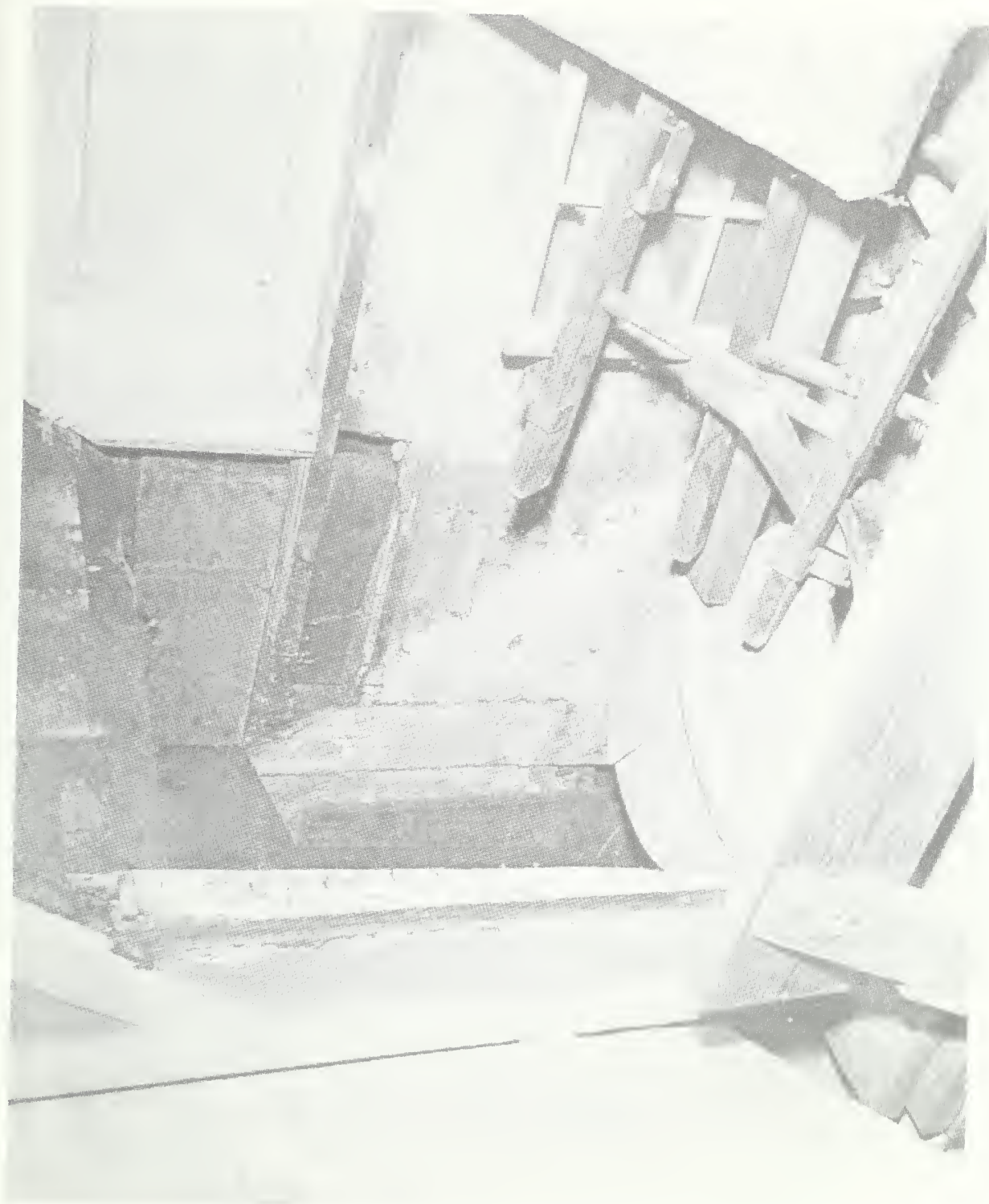
Figure 58. Schuyler House: First story of kitchen wing after ca.-1815 lath and plaster removed; west wall, area under ca.-1815 pass-through to dining-room pantry and paint line of original staircase to second story (1958).
