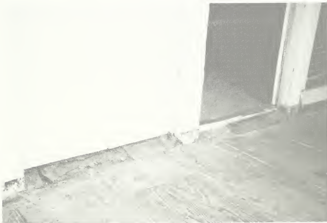
Figure 229. Second-story kitchen hall (Room 206), east wall, later flooring in adjacent rooms beveled to meet original flooring in room.
