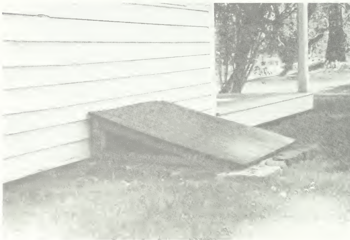
Figure 117. Main house, south elevation, window W004 areaway cover.
