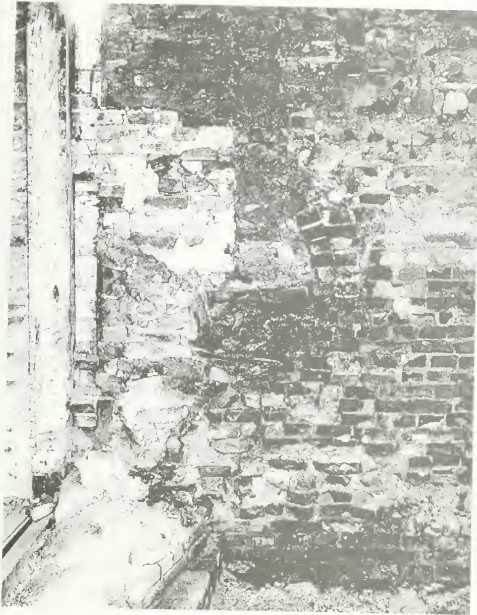
Figure 60. Schuyler House: First story of kitchen wing, east wall after post-1780 fireplace removed (1958); detail shows evidence of bake oven.
