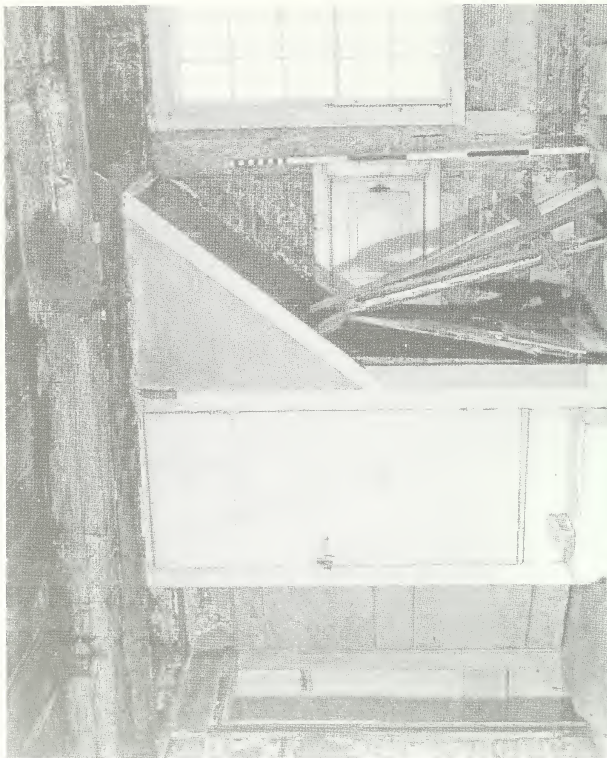
Figure 57. Schuyler House: First story of kitchen wing after ca.-1815 lath and plaster removed; ca.-1815 features at south end of west wall (1958). From left: doorway to east tier, doorway and staircase to second story, pass-through to dining-room pantry, and window in former ca.-1780 exterior doorway.
