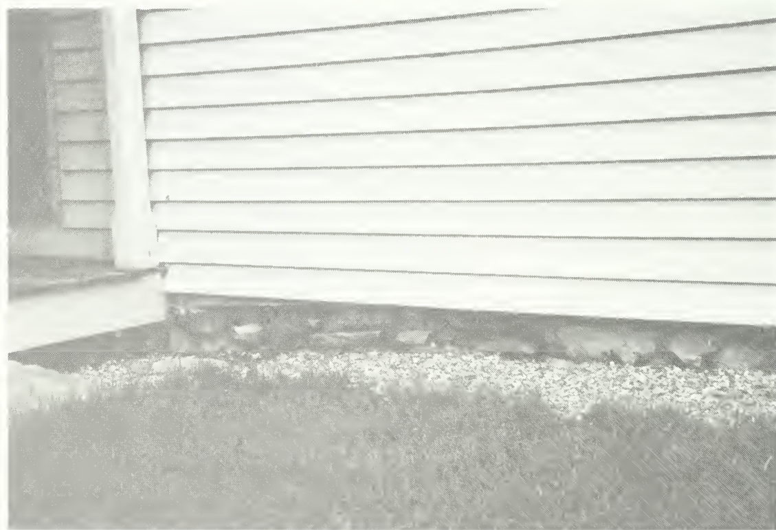
Figure 131. Kitchen wing, south elevation, fieldstone foundation.
