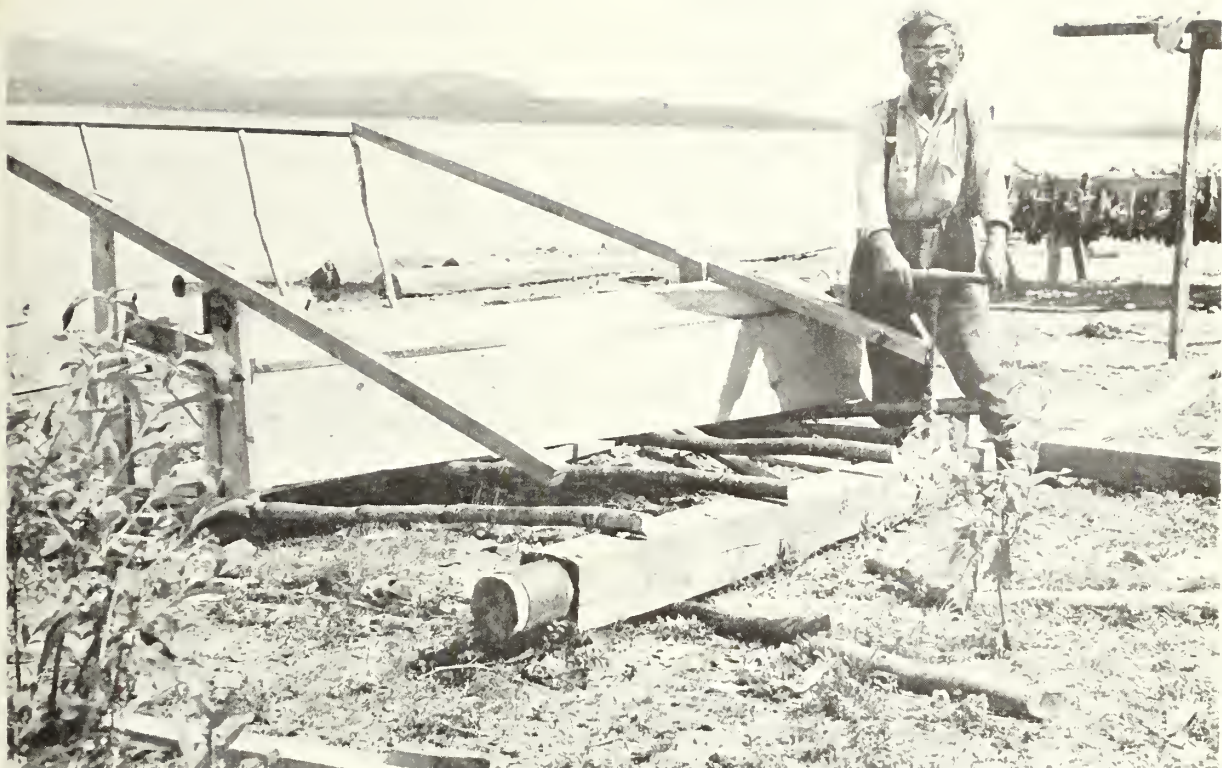
Figure 32.--This resident of Aniak on the lower Kuskokwim River is building a fish wheel from materials obtained locally--a few boards from a local sawmill and saplings from along the river.
