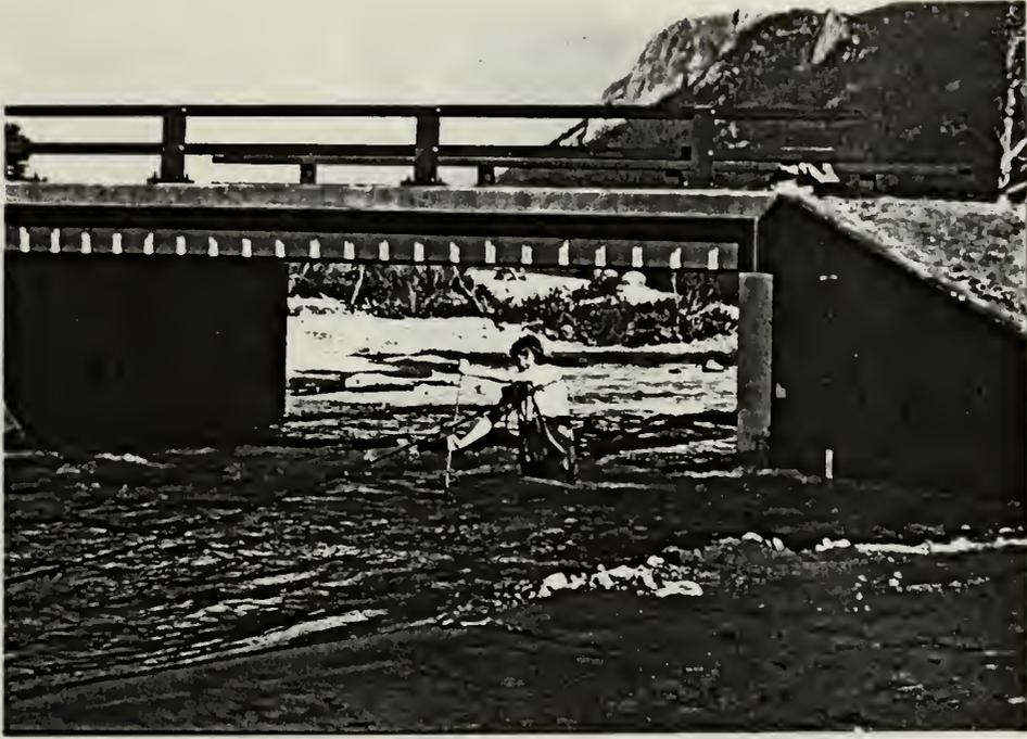
Figure 3a. Stream gaging using wading rod with rotary cup meter.
