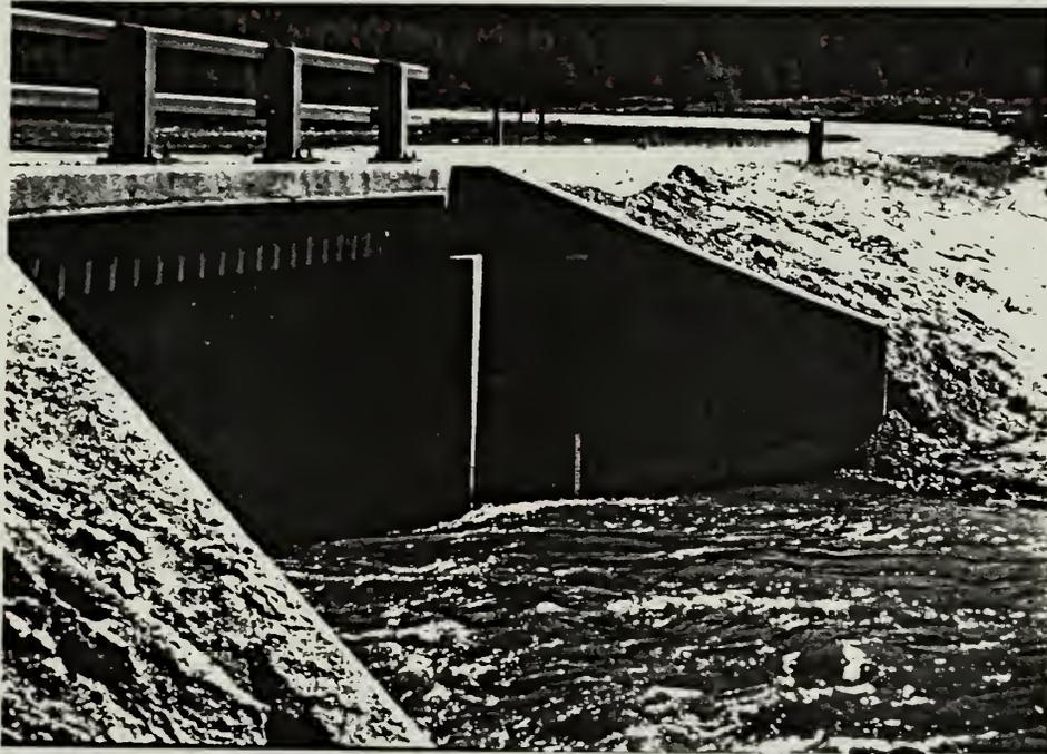
Figure 2. Gage site at Horseshoe Park. The gage staff is visible on the wing wall.
