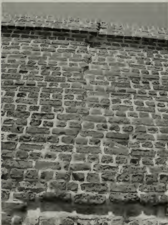
Image 5. Fort Sumter, April 2009. East elevation, example of typical brick deterioration on this elevation. Note presence of white salt crystals on surface (S) and subsequent small brick spalls, as well as the difference in rate of deterioration of brick fire skin versus interior.
