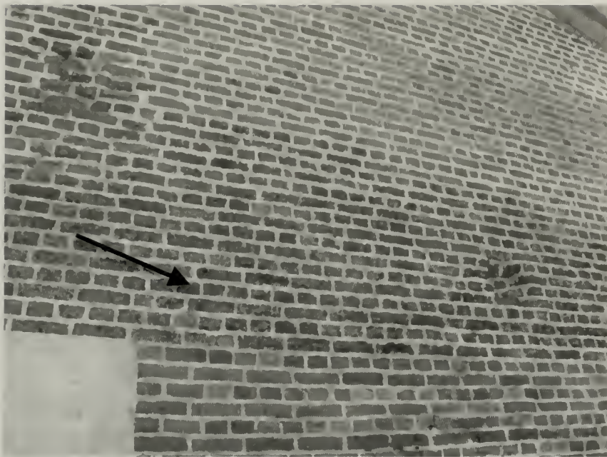
Image 3. Fort Sumter, April 2009. North elevation, showing example of modern re-pointing and condition of brick. Note more deteriorated band of brick at bottom center.
