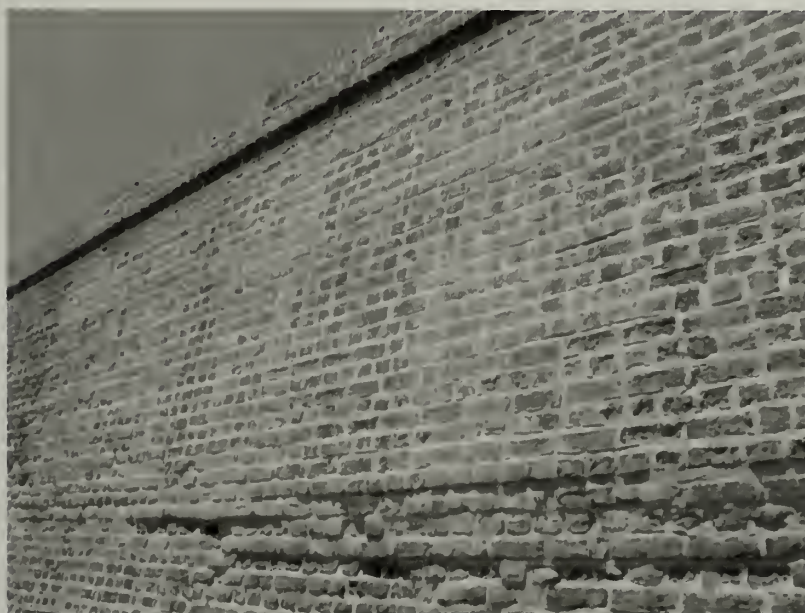
Image 12. Fort Sumter, April 2009. Southeast Elevation, area re-pointed in 2008 using Rosendale natural cement gauged with hydrated lime. The streaking on the wall is most likely due to the lime component of the mortar washing out of the mortar prior to achieving full carbonation.
