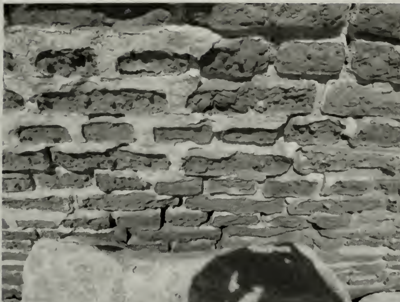
Image 11. Fort Sumter, April 2009. Exterior scarp wall, an area of prior re-pointing campaign based predominantly on Portland cement. Note condition of surrounding brick, it has weathered at a more advanced rate than the mortar, producing a characteristic “honeycomb” effect.
