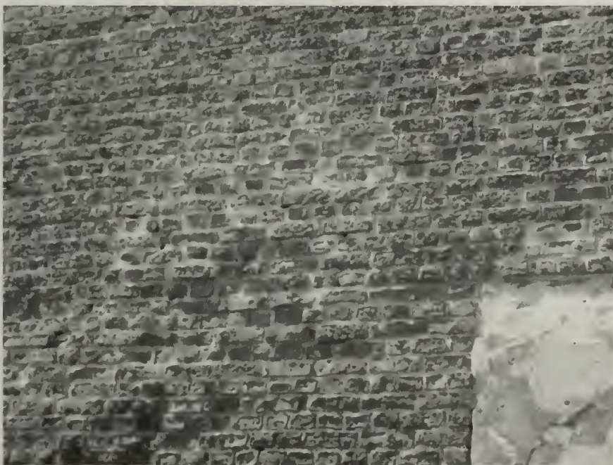
Image 4. Fort Sumter, April 2009. East elevation, detail of brick condition. This wall receives more wave impact and saturation with sea water than others and the brick is subsequently more deteriorated.
