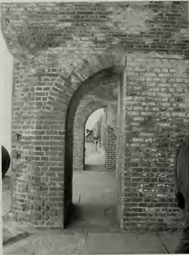
Images 1 and 2. Fort Sumter, April 2009. The first tier casemates contain areas of relatively intact interior brickwork and mortar. These brick represent the original appearance and condition of the Carolina Grey bricks.
