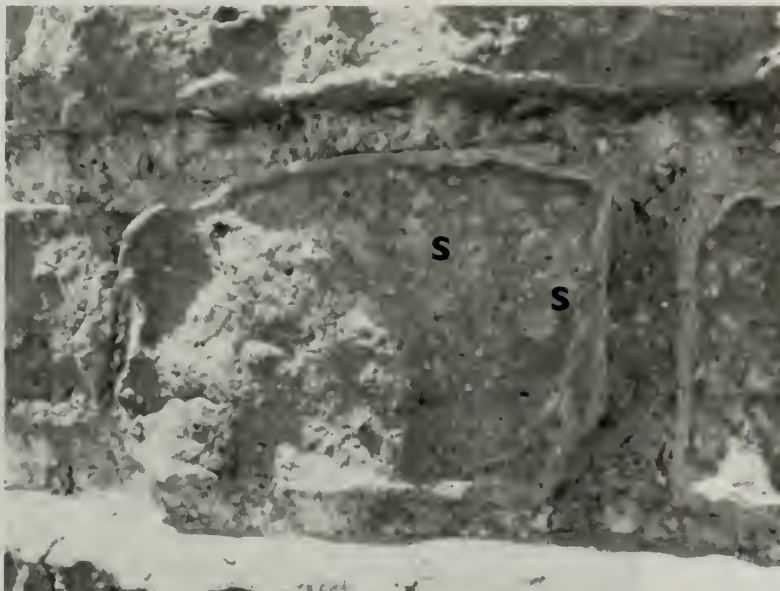
Image 5. Fort Sumter, April 2009. East elevation, example of typical brick deterioration on this elevation. Note presence of white salt crystals on surface (S) and subsequent small brick spalls, as well as the difference in rate of deterioration of brick fire skin versus interior.
