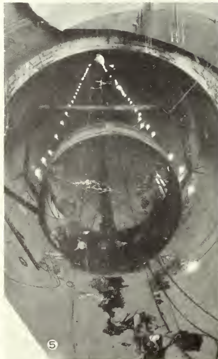
1, Thirty-foot diameter penstock pipes awaiting transportation to damsite; 2, Boulder City, Nev., as seen from air; 3, top working of dam seen from point slightly upstream on Nevada rim. Top forms at elevation 1145. Downstream Arizona intake tower in upper left; 4, downstream Arizona intake tower with the two Nevada intake towers in background, seen from Arizona canyon rim; 5, Thirty-foot diameter penstock pipe section ready for hoisting into position beneath beader tunnel No. 3; 6, looking obliquely upstream along overflow weir of Arizona spillway. View shows piers with 16 x 100-foot drum gates in lowered position.
