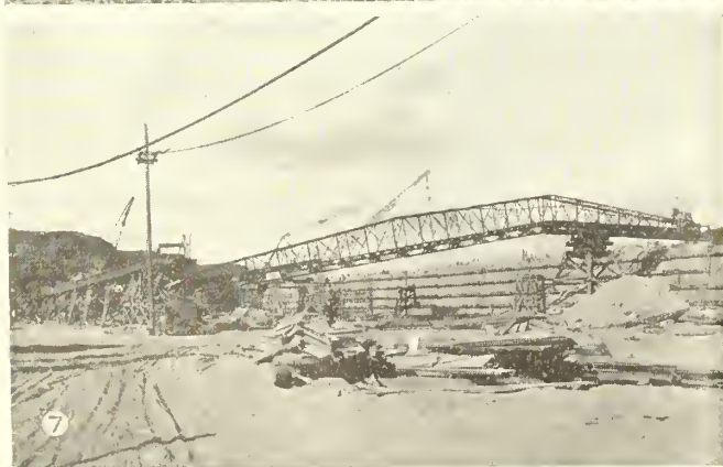
1, Main line of belt conveyor; 2, Converging conveyors from feeders Nos. 2 and 3 and central hub; 3, Bleeder and shuttle conveyors; 4, Boom of stacker unit; 5, "Spoil bank" showing a slip near stacker boom; 6, "Spoil bank" showing approximately 2\frac{1}{4} million cubic yards; 7, Shuttle and boom conveyors filling cofferdam cells; 8, Ten-yard buggies dumping into feeder No. 2.
