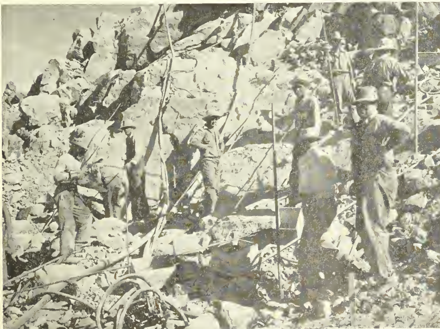
Building Boulder Dam with drills, air hose, pipe, and dynamite. These men, like those who worked in the factories from coast to coast and those who actually poured the concrete, constructed Boulder Dam.
