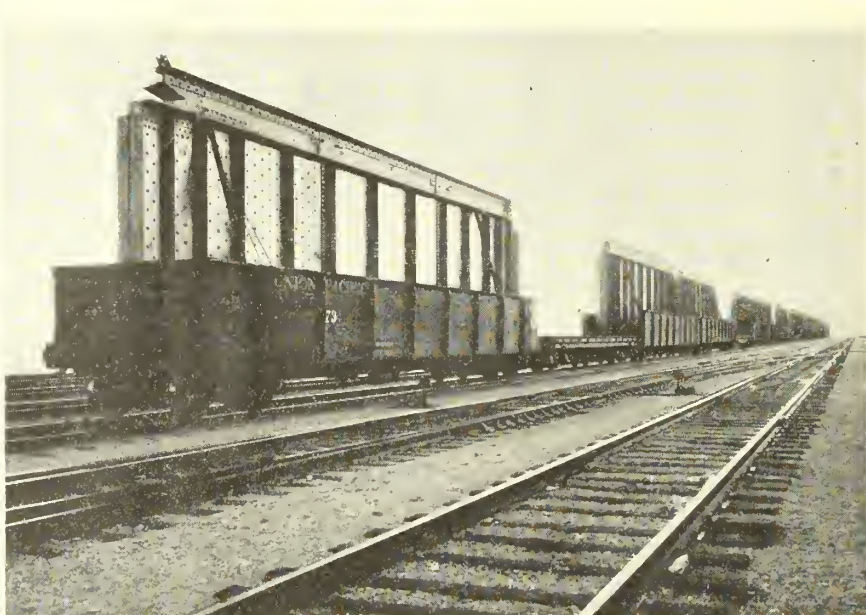
A trainload of steel on a siding at Boulder City during construction of Boulder Dam. A total of 27,092 carloads of material arrived at this yard between February 1931 and February 1935 for use in building the dam.
