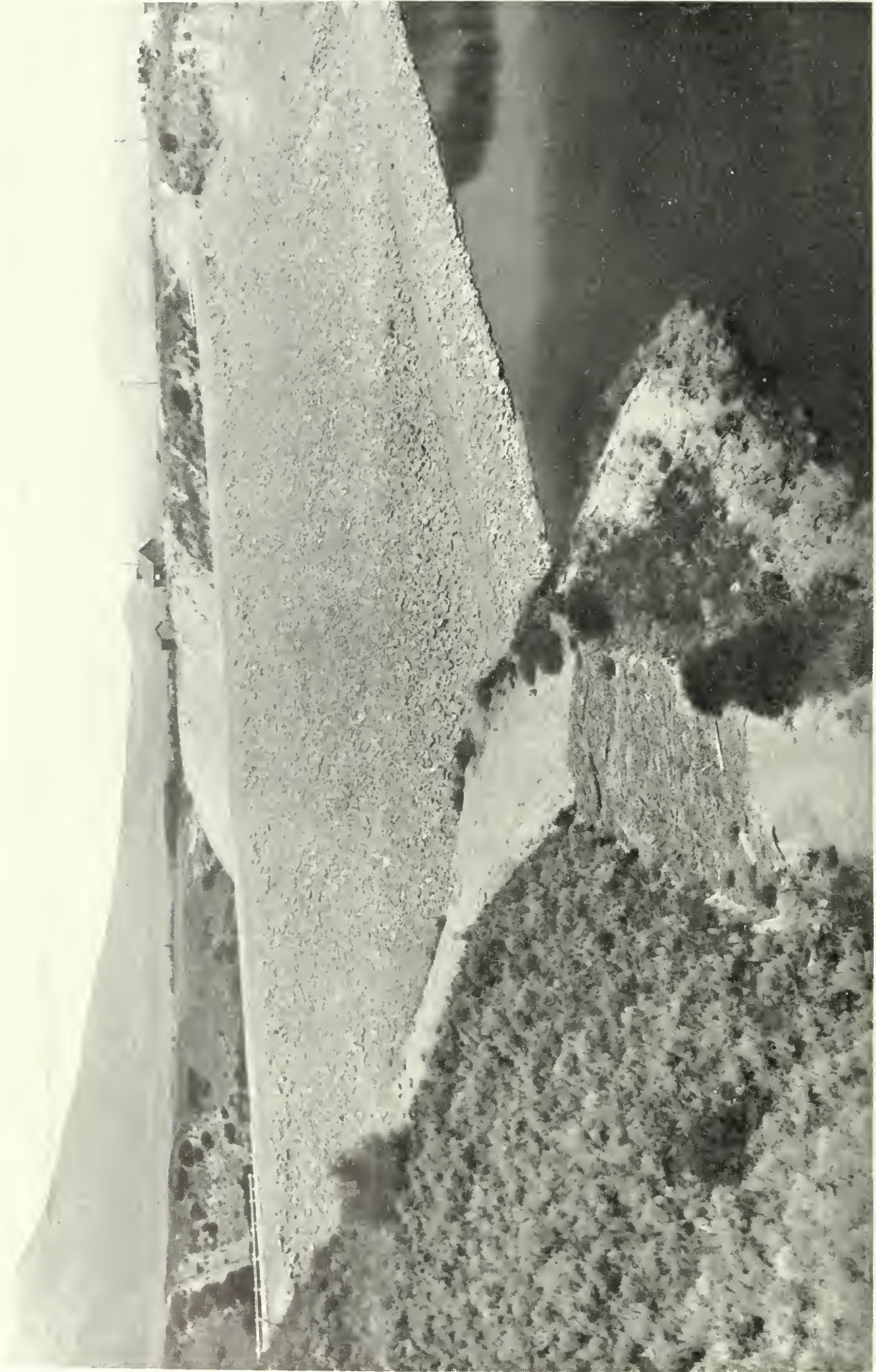
UPSTREAM SLOPE OF HYRUM DAM, HYRUM PROJECT, UTAH This 90-foot earthen structure is one of three storage dams in Utah under construction by the Bureau of Reclamation to supplement the inadequate water supply of the irrigation projects in that State
