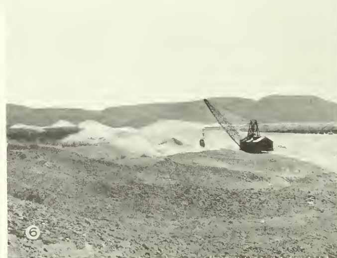
1, EXCAVATING WITH TRACTORS; 2, EXCAVATING WITH HORSES; 3 AND 4, A 12-CUBIC YARD BUCKET; 5 AND 6, EXCAVATING WITH DRAGLINES.
