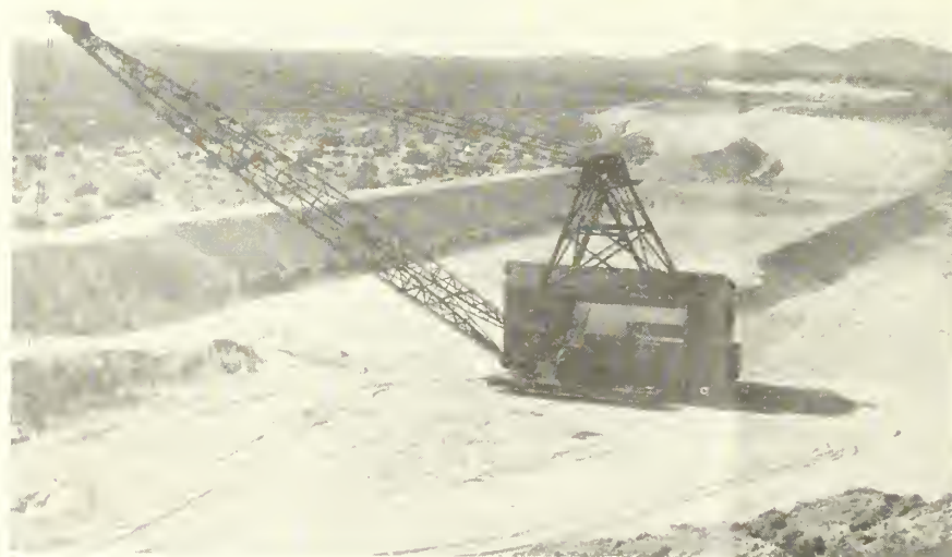
650-ton dragline at work on All-American Canal
