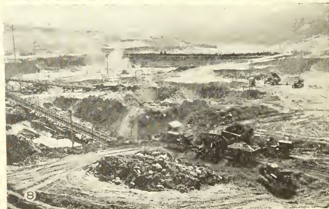
1, Main line of belt conveyor; 2, Converging conveyors from feeders Nos. 2 and 3 and central hub; 3, Bleeder and shuttle conveyors; 4, Boom of stacker unit; 5, "Spoil bank" showing a slip near stacker boom; 6, "Spoil bank" showing approximately 2\frac{1}{4} million cubic yards; 7, Shuttle and boom conveyors filling cofferdam cells; 8, Ten-yard buggies dumping into feeder No. 2.
