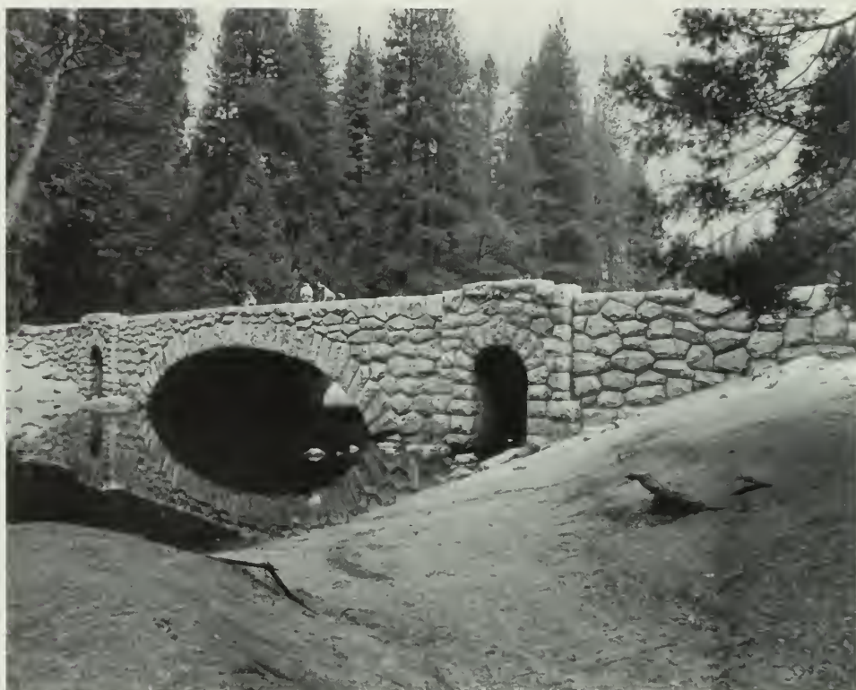
View showing the east facade of the Stoneman Bridge, Yosemite National Park, Mariposa County, California, designed and built by the National Park Service in 1933. The bridge is reinforced concrete faced with rough boulders of native granite to give it a rustic appearance. The photograph shows the exterior material very clearly and also shows significant features—the equestrian tunnels—and how they are built out from the face of the wing walls for decorative emphasis. (National Park Service, Dean Shenk, 1976)
