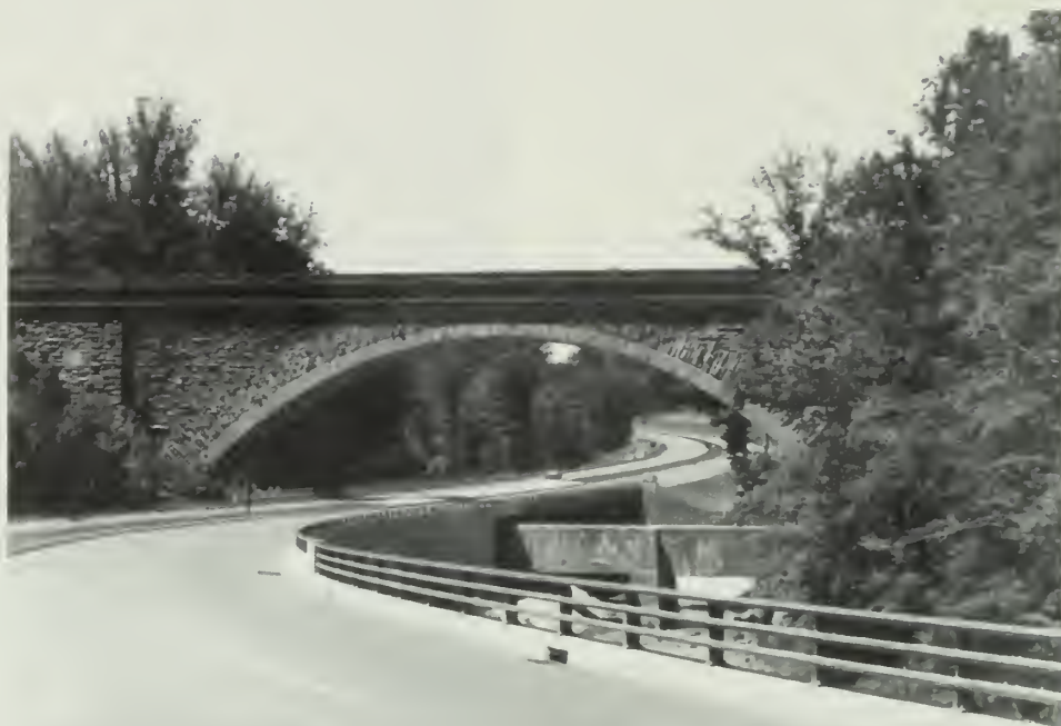
Cabin John Aqueduct, Montgomery County, Maryland. This stone arch was built in 1869 and was the world's longest until 1903. It was designed by Montgomery Meigs, U.S. Army Corps of Engineers. The aqueduct provided the principal source of water to Washington, D.C. throughout the late 19th century. (Michael Bourne, 1969)
