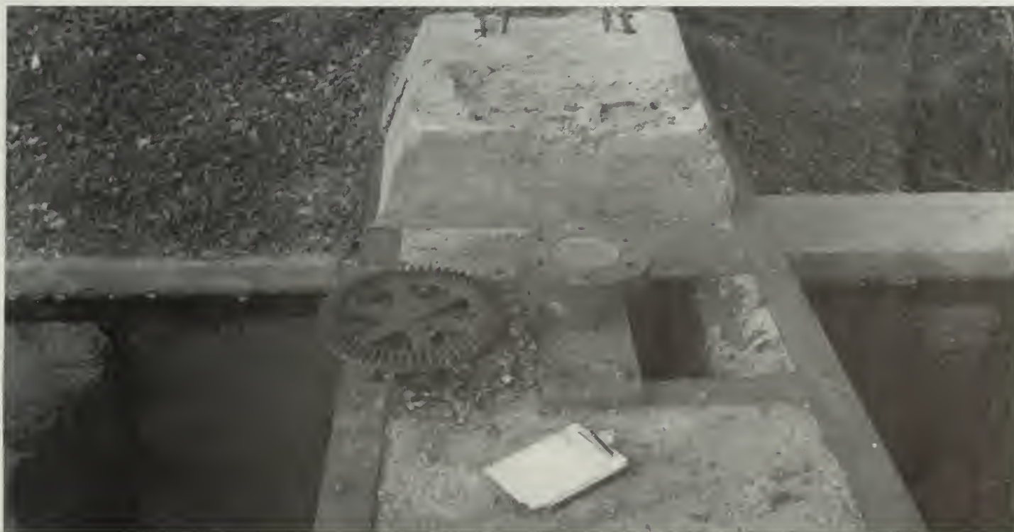
View facing north of the machinery foundation above the wheel pit at South end of ditch at the Thompson—Cape Dam and Ditch Engineering Structure, San Marcos, Hayes County, Texas. Note clipboard placed near spindle head and gear to show scale. (Texas Historical Commission. Margaret Howard, 1984)
