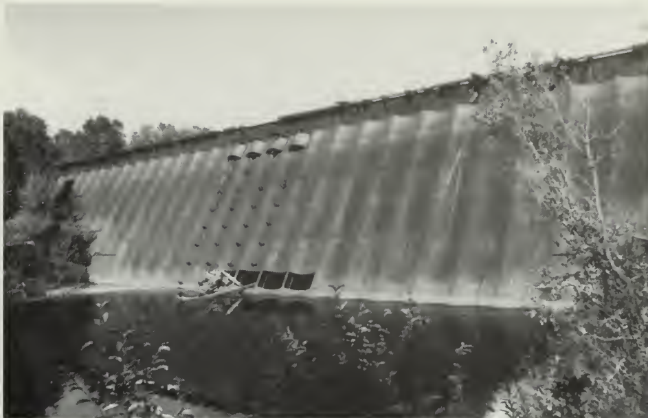
The Redridge Steel Dam, built in 1900, is one of two dams on the Salmon Trout River, near the village of Redridge, Houghton County, Michigan. A few hundred feet upstream stands an earlier stone-filled, log, crib dam built in 1894. The steel dam replaced the log one, which was submerged within its reservoir from 1901 until the reservoir was drained in 1960. (Terry S. Reynolds, 1989)
