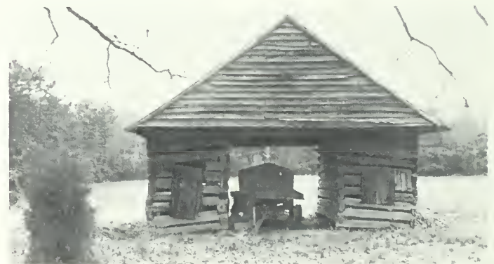
Fig. 3. This mid-19th century double-pen cornercrib on the Jamison Farm in Rowan County, North Carolina, is an example of a type of log building that did not require chinking. Photo: Denise Whitley.
