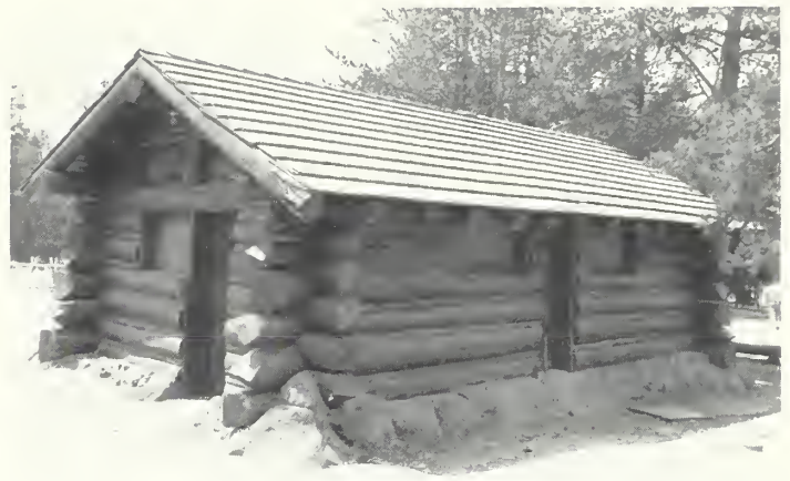
Fig. 18. Exposed roofing members of Rustic style buildings such as this structure at Yellowstone National Park are highly susceptible to deterioration. Photo: Laura Soulliere Harrison.
