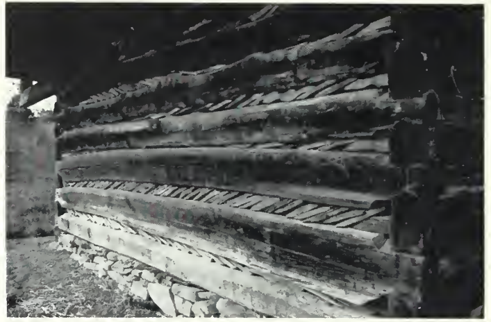
Fig. 12. The log joints have been cleaned out in preparation for new daubing exposing carefully laid stone chinking in this building in Virginia. Photo: Bernard Weisgerber.
