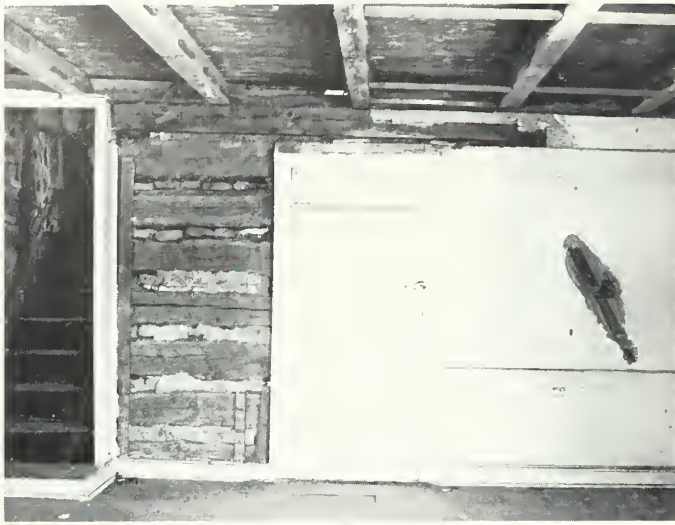
Fig. 16. This photograph of the interior of a 1793 log house in Maryland reveals much about historic log building construction and interior finish treatments. To the left of the plank door plaster has been removed exposing the stone chinking and lathing; remnants of vertical furring strips attached to the logs show evidence of traditional horizontal lath, while the hole broken through the plaster wall on the right shows the use of diagonal lath. The open door reveals a very steep, enclosed stairway typical of many early log houses. Although plaster has been removed from the ceiling, the wall to the right of the door shows the original plaster finish and fine woodwork including beaded chair rail, floor and door molding. Photo: National Park Service Files.
