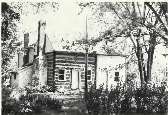
Fig. 13. Historic wood clapboard siding originally applied to conceal the fact that this house was built in two sections of different materials has been inappropriately removed from the 1793 log portion. Photo: National Park Service Files.
