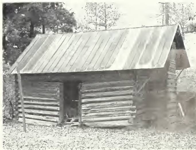
Fig. 15. The mid-19th century O’Quinn House, Moore County, North Carolina, provides a rare surviving example of a clay-lined log chimney. Although the logs of the house are saddle-notched, the chimney logs are “V” notched. The roof was extended out over the chimney to protect the daubing from the weather, and the chimney stack would have originally projected through a hole in the roof. Photo: Michael Southern.
