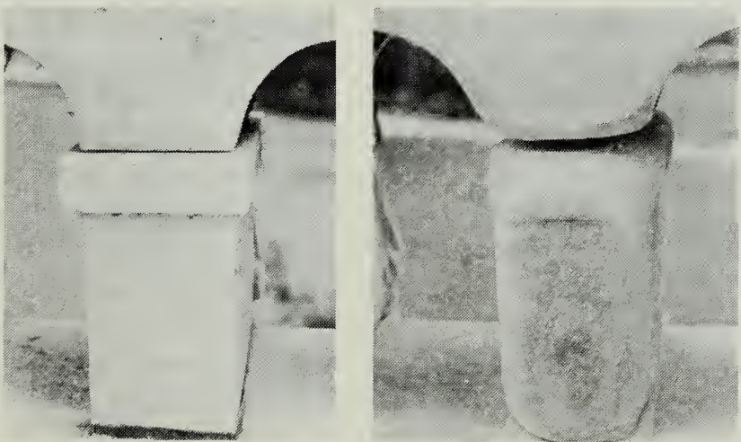
Weathering has reduced the formerly sharp edges and rounded the corners of this marble baluster. Photograph: John H. Myers.
