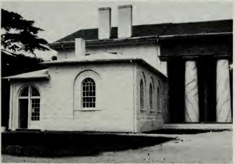
Paint used as a purely decorative aspect to simulate marble on a stucco surface. Photograph: National Park Service.
