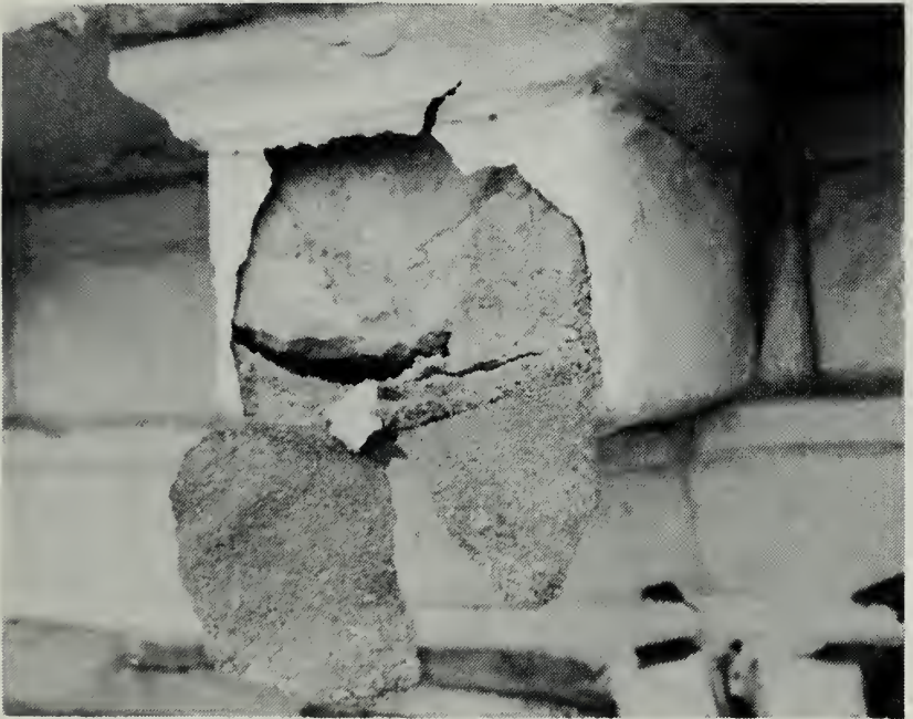
A neoprene coating over a limestone cornice has trapped water (which entered through leaks in the parapet) inside these stone dentils. The built-up water pressure has finally forced the coating to pop off, taking with it pieces of the stone. Photograph: National Park Service.
