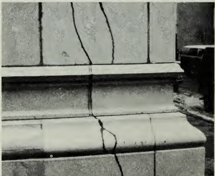
Cracking of glazed terra cotta. Photograph: National Park Service.
