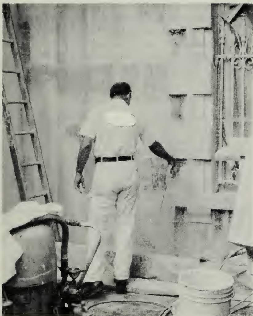
Paint removal from sandstone. Photograph: Baird M. Smith, AIA.
