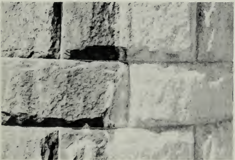
Chemical cleaning to remove urban dirt and pollution from granite without causing damage or abrasion to the surface of the stone.
