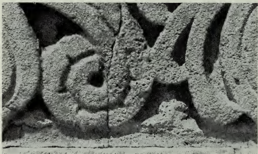
Cracking of limestone. Photograph: John H. Myers.
