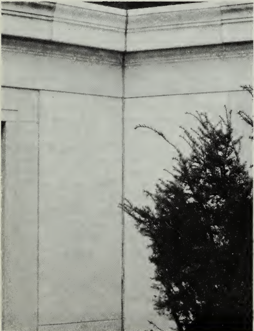
The two sections in the center have been replaced with marble matching the original. Photograph: Anne E. Grimmer.
