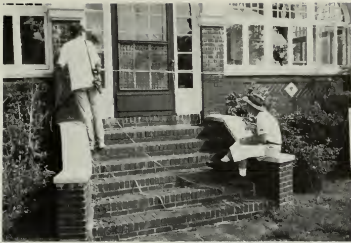
Figure 4. Documenting the building's history, preparing schematic plans, and assessing the condition of the building will provide necessary information on which to set priorities for stabilization and repair prior to securing the building. Photo: Frederick Lindstrom, HABS.
