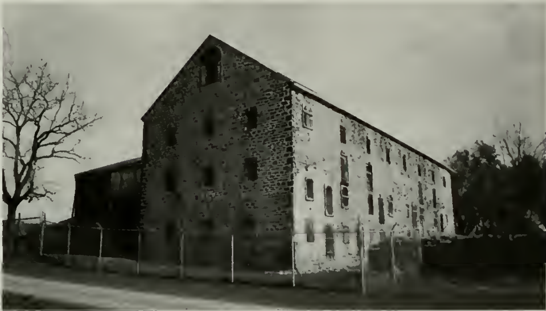
Figure 24. Once mothballed, a property must still be monitored and maintained. The openings in this historic barn have been modified with a combination of wood louvers and metal mesh panels which require little maintenance. The grounds are regularly mowed, even inside the chain link security fence. Photo: Williamsport Preservation Training Center, NPS.
