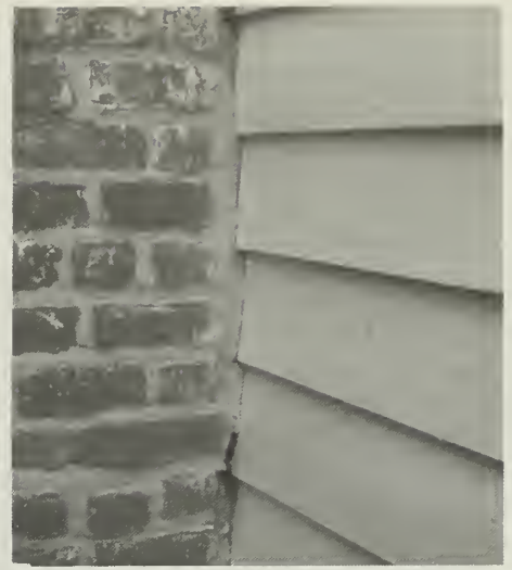
Figure 8. Appropriate mortar mixes should be used when masonry repairs are undertaken. In this case, a soft lime based mortar is used as an infill between the brick and wooden elements. When full repairs are made during the restoration phase, this soft mortar can easily be removed and missing bricks replaced.
