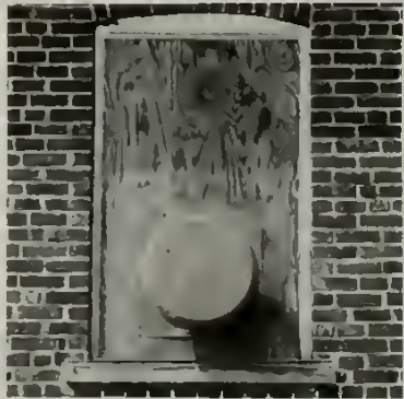
c. The exhaust fan has tamper-proof housing.
