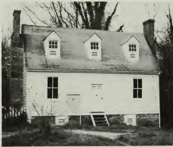
Figure 10. Regrading around the Booker Tenement at Colonial Williamsburg has protected the masonry foundation wall from excessive damp. This building has been successfully mothballed for over 10 years. Note the attic and basement vents, the temporary stairs, and the informative sign interpreting the history of this building.
