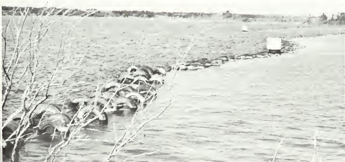
Floating tire breakwater used to improve recruitment of young largemouth bass in a wind-swept cove (to the right of the photograph) of an Oklahoma reservoir. Oklahoma Cooperative Fishery Research Unit photo.
