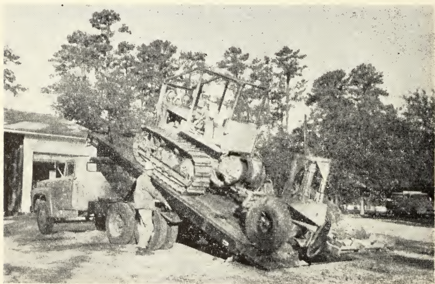
FIGURE 3.—Tractor and plow being unloaded from tilt bed. Operator is manipulating controls. This is the maximum elevation of bed. Tractor and plow are descending slowly; held back by cable. Operator can ease the tractor unit down. Weight and momentum of tractor-plow unit permit sufficient descent until all except the last cleat of tractor is on ground. Momentum is not sufficient to have all of the treads flat on ground. Note approach plate is parallel.
