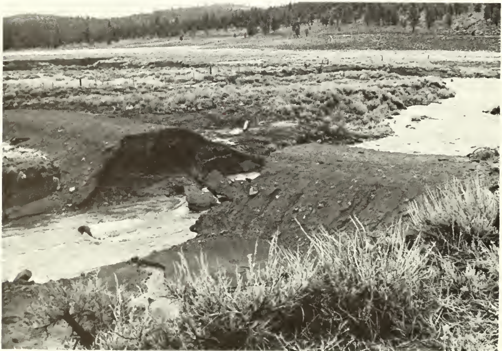
Figure 3.--A Dog Valley erosion control dam destroyed during 1963 winter flood. The flow shown here on February 1 was less than half that during the flood peak.
