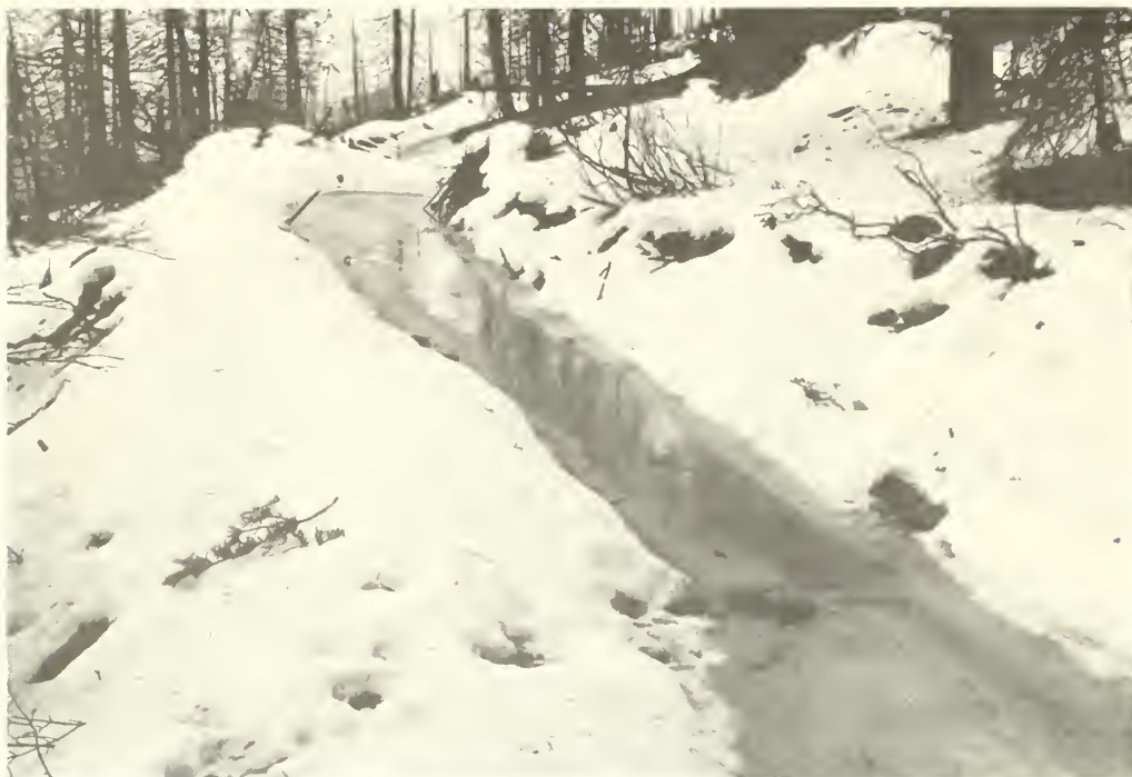
Figure 4.--Water from the 1963 flood-producing storm trapped in a portion of one contour trench in the Dog Creek watershed. Detention storage of this type should reduce flooding downstream.
