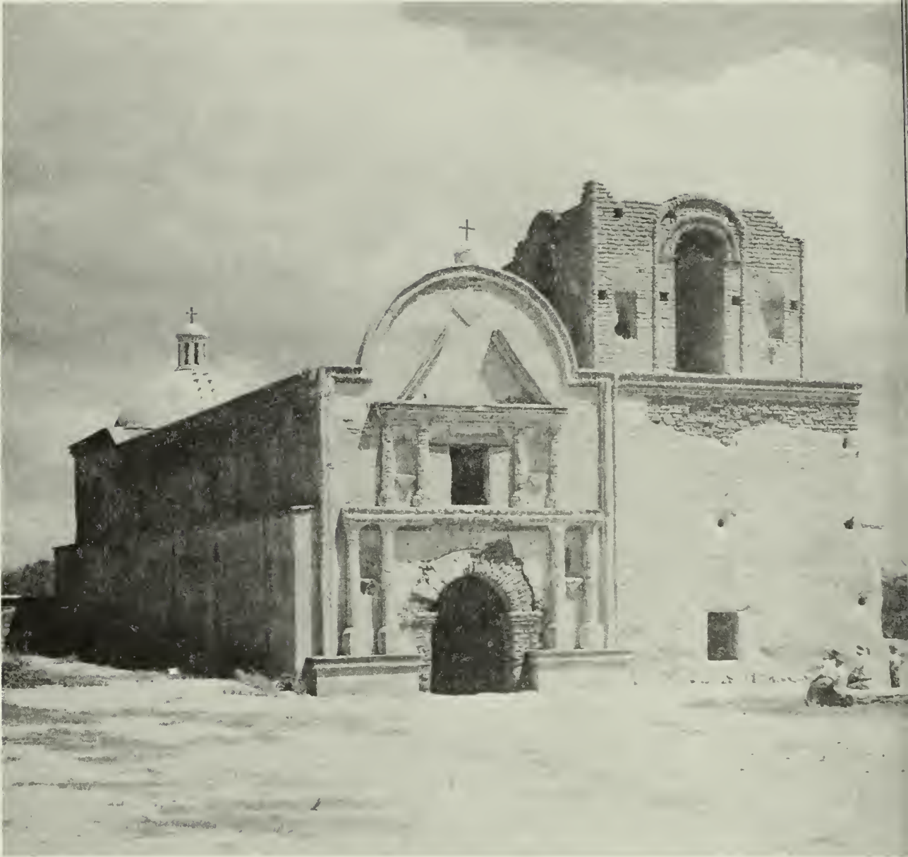
The Mission Church, Tumacacori National Monument, Tumacacori, Arizona. Comprehensive stabilization, repair, and partial restoration of the Mission Church was performed in 1921 by Frank Pinkley. Lower portions of the columns and bases of the facade were restored in 1945. Since that time, all efforts by the National Park Service have been directed to preserving existing original construction. Replacement plaster, where required to cover eroded original lime plaster and adobe brick surfaces, consists of a tinted cement-lime-sand mortar employed with a bonding agent.
