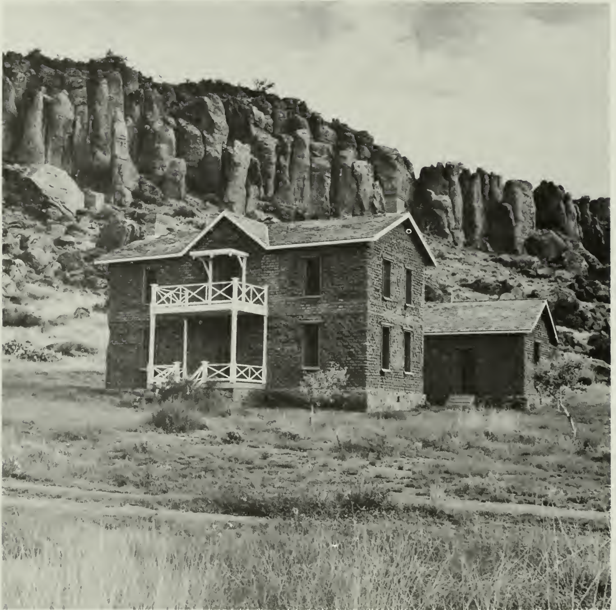
FIGURE 59. Building HB-15 and its outbuilding, a kitchen, following modified restoration by the National Park Service. Soil-cement adobes simulating original adobes were used as modular units of repair. Compare with figure 58.
