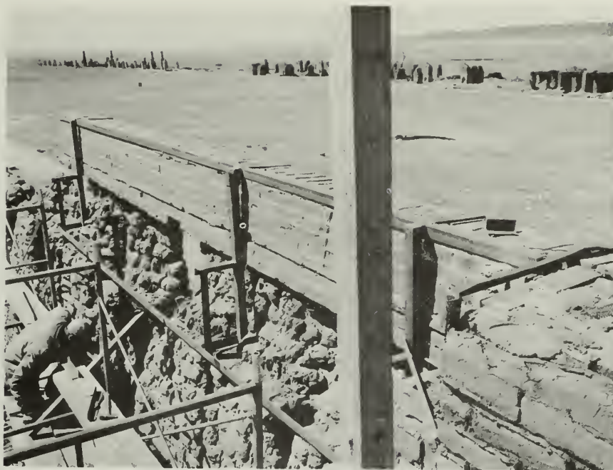
FIGURE 67. Building 3-440, coping on west wall, during stabilization. Fort Union National Monument.
