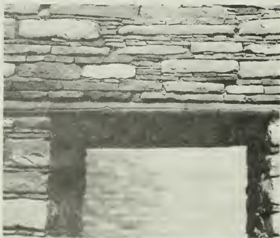
FIGURE 37. The cast concrete lintels have the same appearance as the originals from which they were cast. (Chetro Kettle Ruin, Chaco Canyon National Monument, N. M.)
