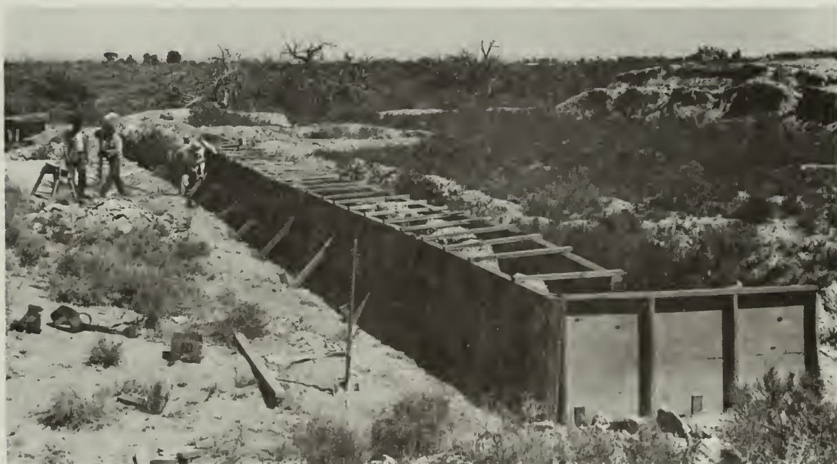
FIGURE 52. Placement of forms for stabilization of a wall with caliche-based soil cement. The forms are braced at the sides and tied at the top. (Compound B, Casa Grande Ruins National Monument, Ariz.)
