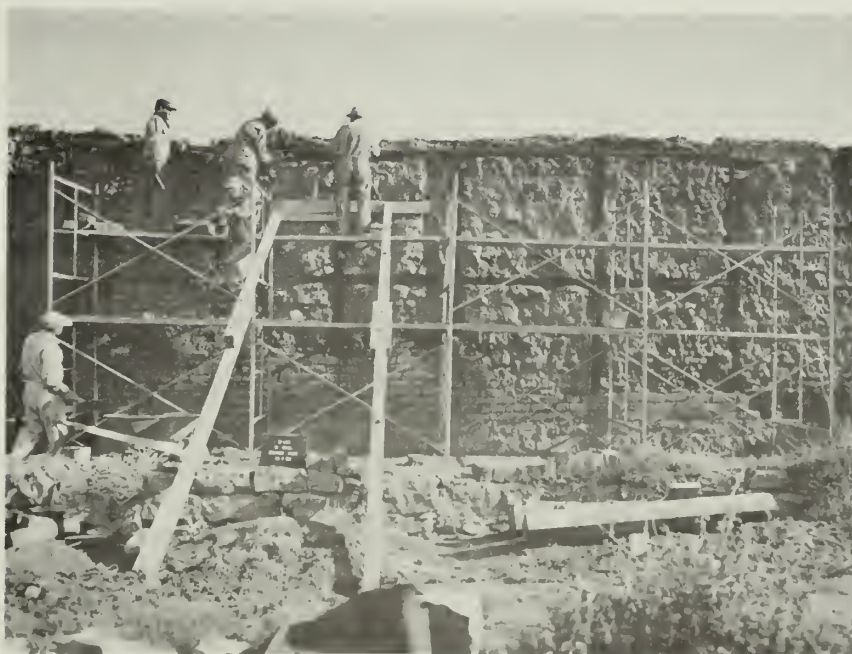
FIGURE 84. Building 3-450, Room 451, north side of south wall, during stabilization. Fort Union National Monument.
