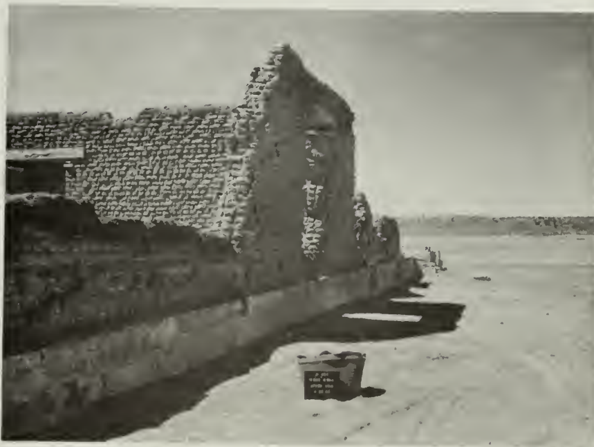
FIGURE 92. Building 3-450, Room 451, north side of north wall, after stabilization. Fort Union National Monument.
