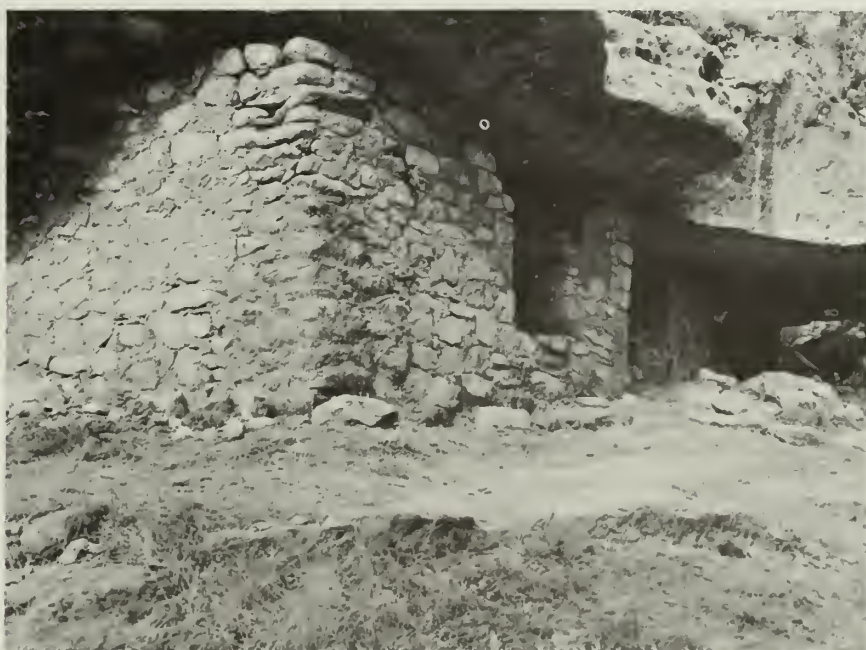
FIGURE 126. Room 1, east exposure, after replacement of fallen corner. The deeply eroded wall base was grouted, and the area above the doorway was partially reset. (Walnut Canyon National Monument)
