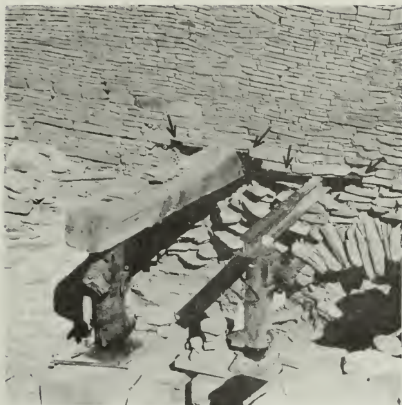
FIGURE 29. A second beam resting on jacks is placed through the wall depicted in figure 28. Arrows indicate extent of steel plates above the beam. The area of settling was reduced with upward pressure.
