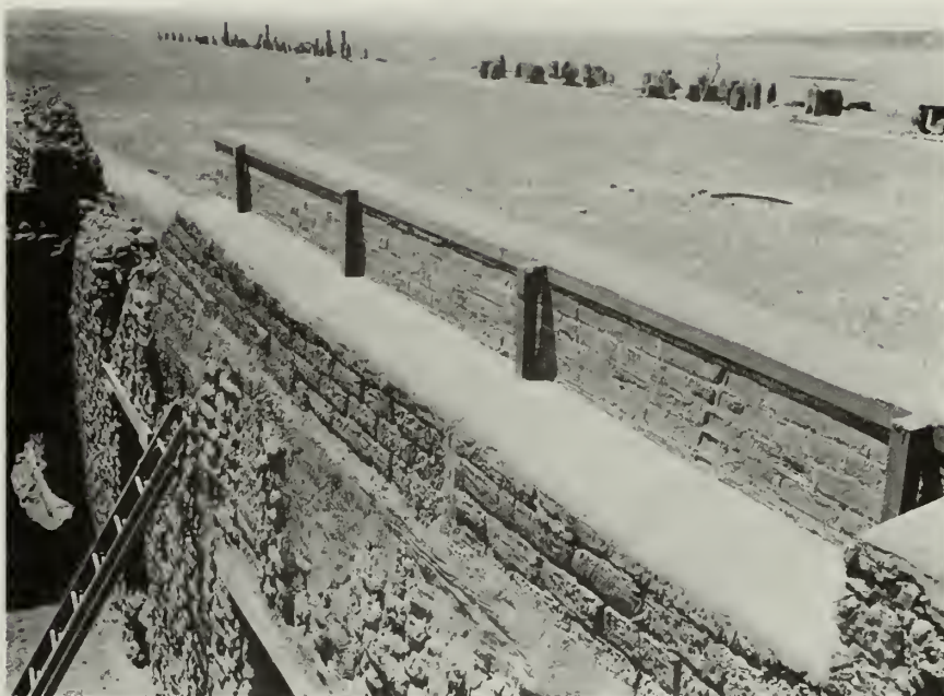
FIGURE 70. Building 3-440, south half of coping on west wall, during stabilization. Fort Union National Monument.
