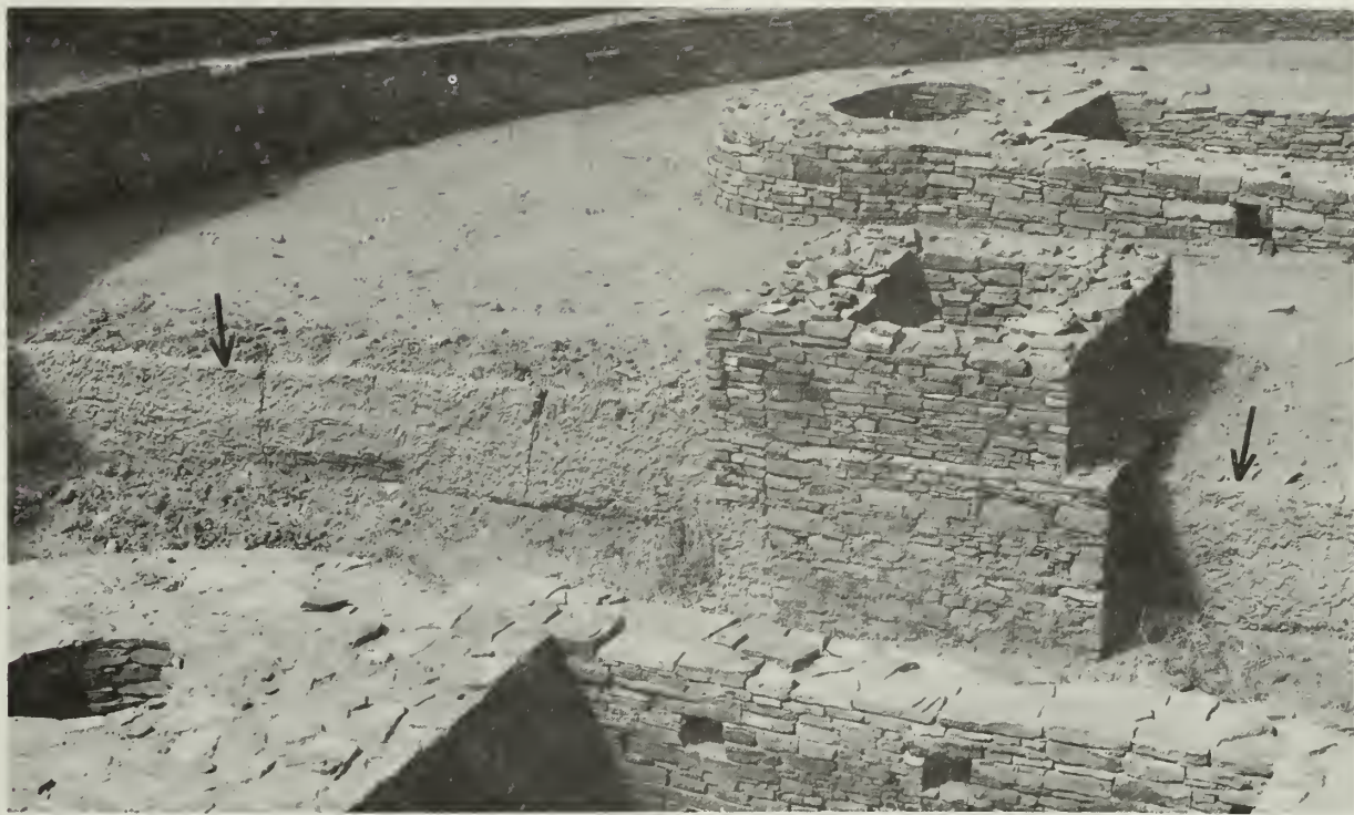
FIGURE 10. Formed soil-cement in retaining sections of fill which must be stabilized to show portions of structures on varying levels. (Great Kiva in the plaza of Chetro Kettle Ruin, Chaco Canyon National Monument, N. M.)
