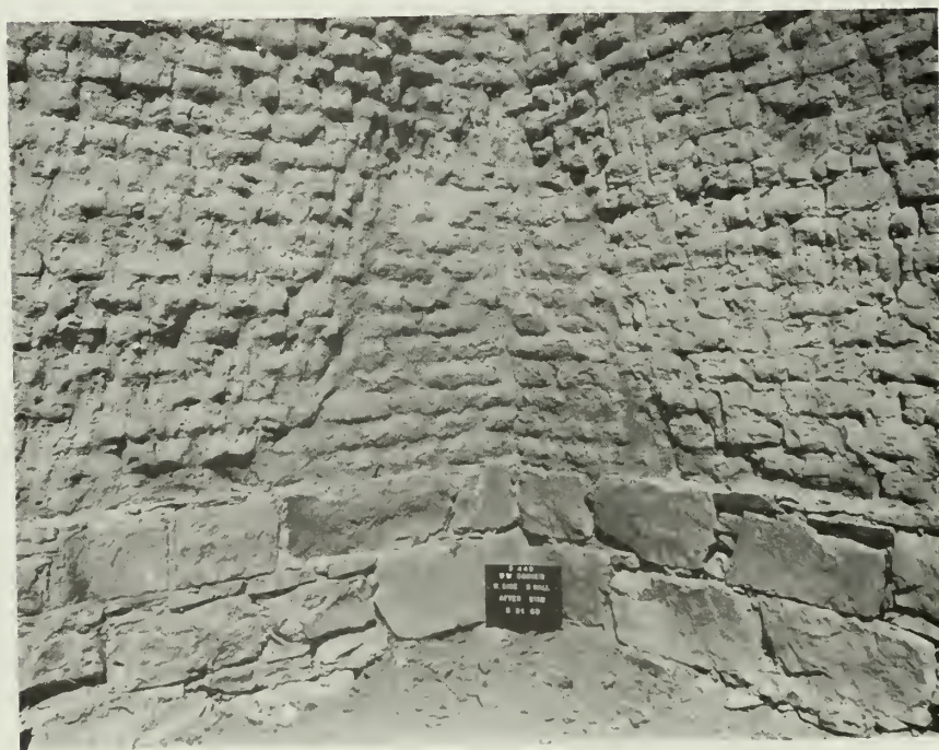
FIGURE 76. Building 3-440, southwest corner, after stabilization. Fort Union National Monument.
