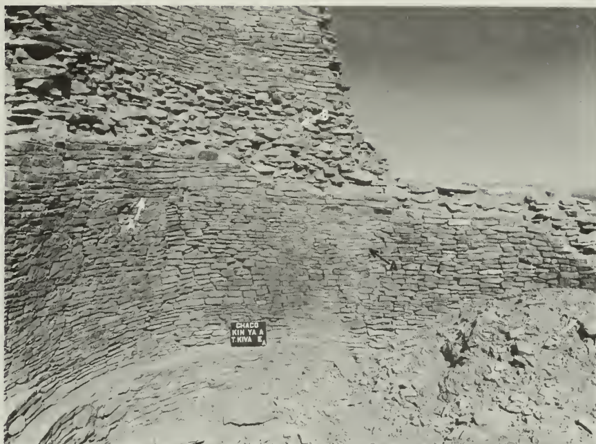
FIGURE 106. Lower portion of Tower Kiva, north and east segments, after stabilization. Offset ledges repaired, holes filled with repair masonry, facing reset (arrows A), top capped and inset core (arrow B) grouted.
