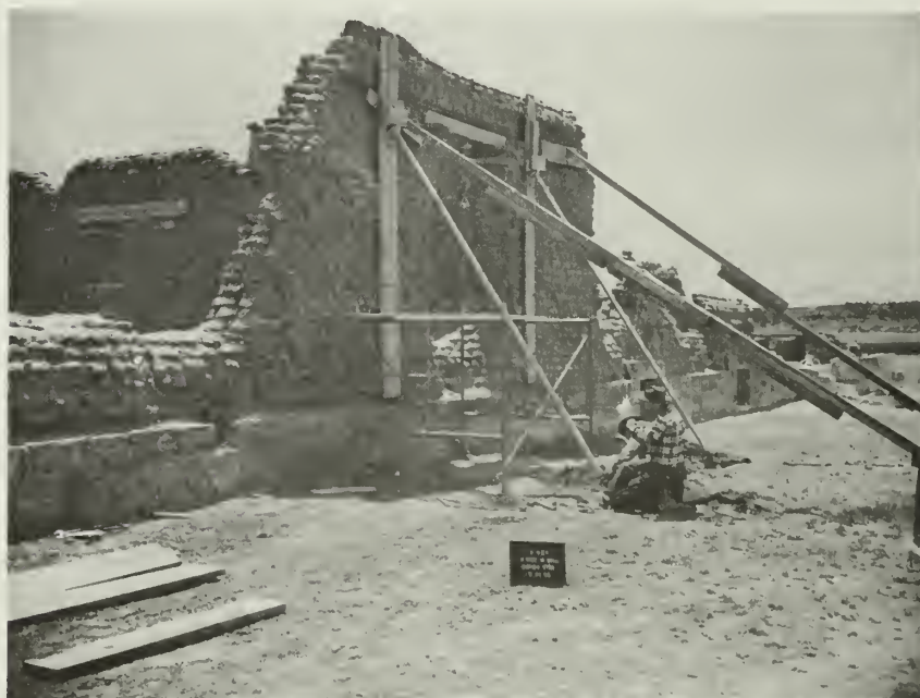
FIGURE 90. Building 3-450, Room 451, south side of north wall, during stabilization. Fort Union National Monument.
