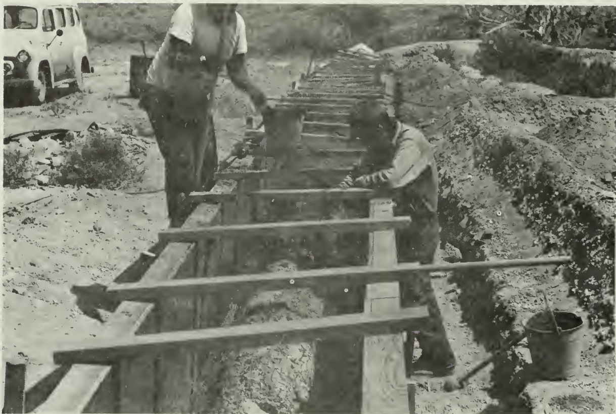
FIGURE 53. The start of placing caliche-cement mix over the wall depicted in figure 52. Note that the forms follow the irregular line of the wall.
