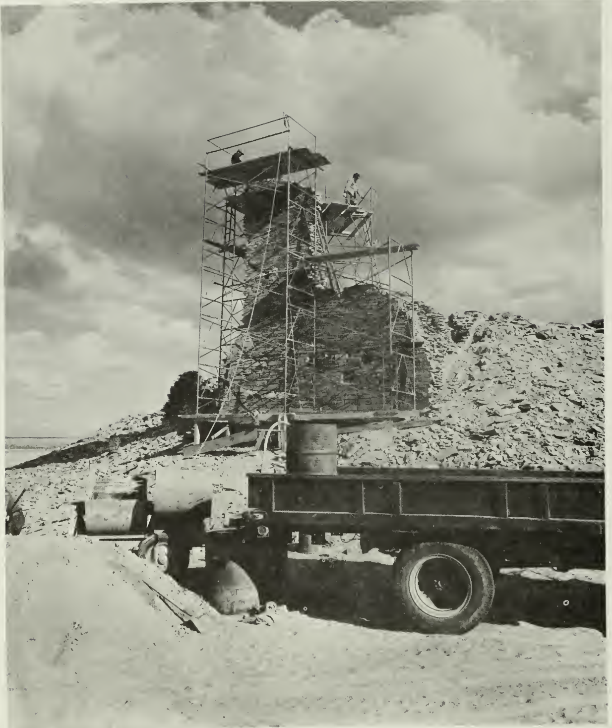
FIGURE 118. Work on the highest portion of the tower. The scaffolding completely surrounded the structure. To provide maximum safety for the workmen, the three sets of scaffolding were anchored at the bases and across the top and through midsections.
