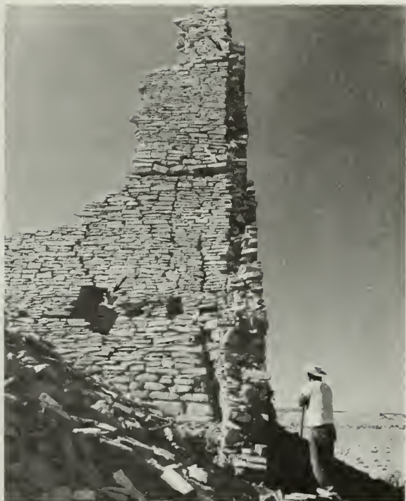
FIGURE 112. Tower Kiva, east wall exterior at juncture with north wall stub (at sign). Note the vertical cracks, eroded savino sockets (arrows) and loose, fragile spire. Portions of 4 stories are visible.
