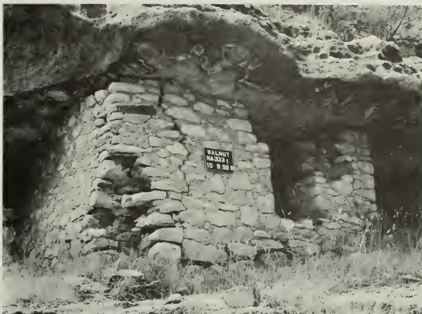
FIGURE 125. Room 1, east exposure, before replacement of fallen corner. (Walnut Canyon National Monument)
