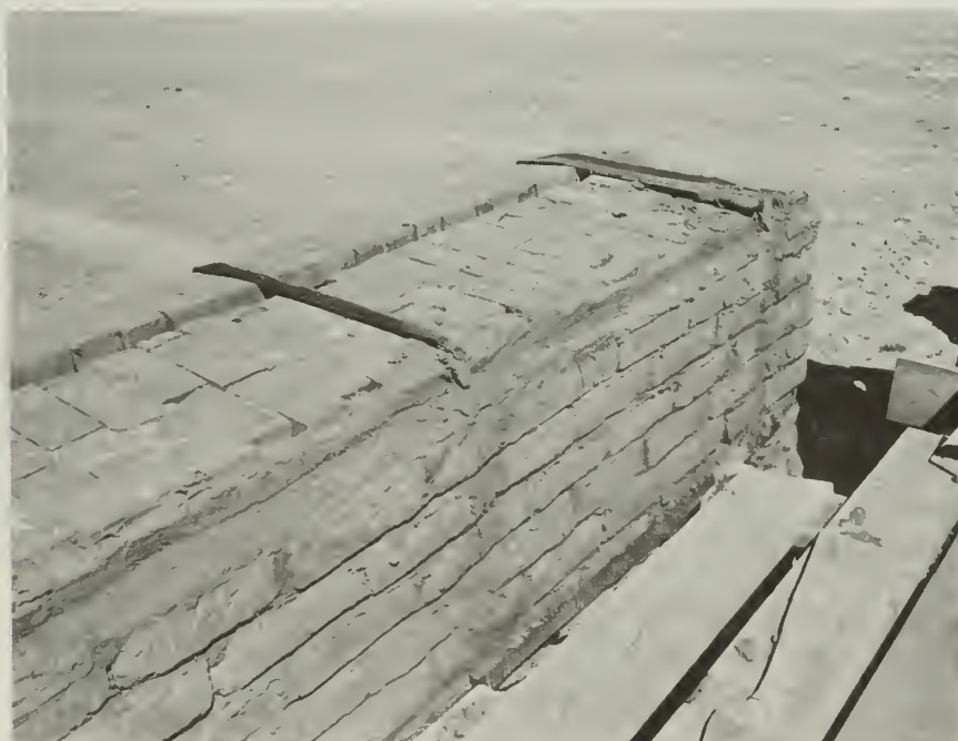
FIGURE 68. Building 3-440, coping on west wall, during stabilization. Fort Union National Monument.
