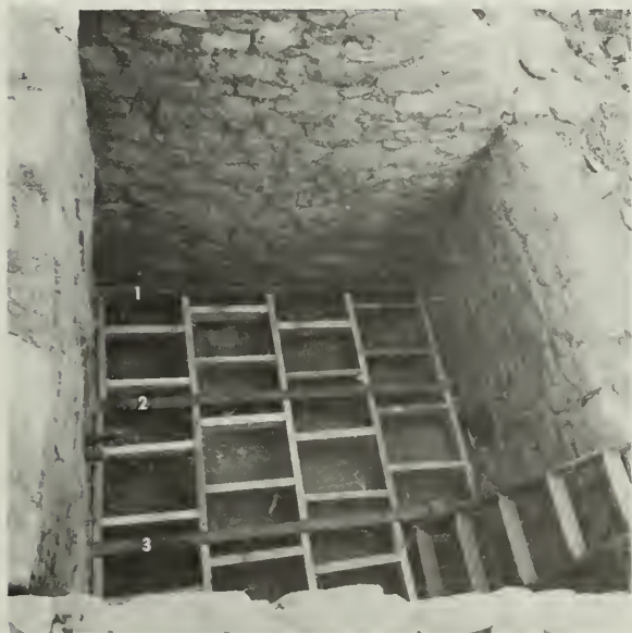
FIGURE 51. Construction of a slab covering. The numbered members are I-beams run through heavy masonry walls. The longitudinal members are 2 x 4's inset in the I-beams as purlins. Corrugated metal decking will be nailed to the wood as a base for a concrete slab. A covered vent will be provided through the concrete. Drainage will be provided by tile line through the wall at the right. (East Ruin, Aztec Ruins National Monument, N.M.)
