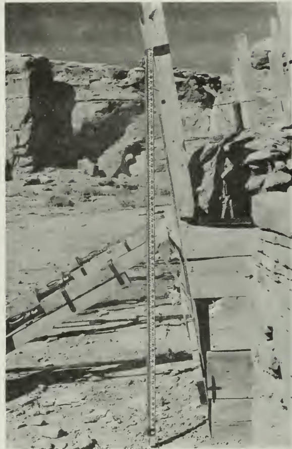
FIGURE 34. Realignment of wall depicted in figure 33. The framework is in place on both sides and is tied together. Frame lined with asphalt paper, space between frame and wall packed with sand. Note that the five screw jacks in sleeves bear against a 4 x 4 timber to distribute pressure.
