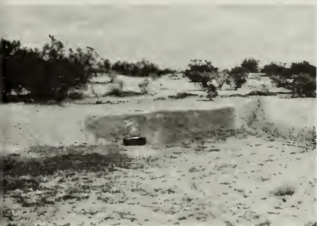
FIGURE 13. West wall of Compound A immediately after a rain. The light areas treated with silicone repelled water. The darker areas were untreated and absorbed moisture rapidly. (Casa Grande Ruins National Monument, Ariz.)
