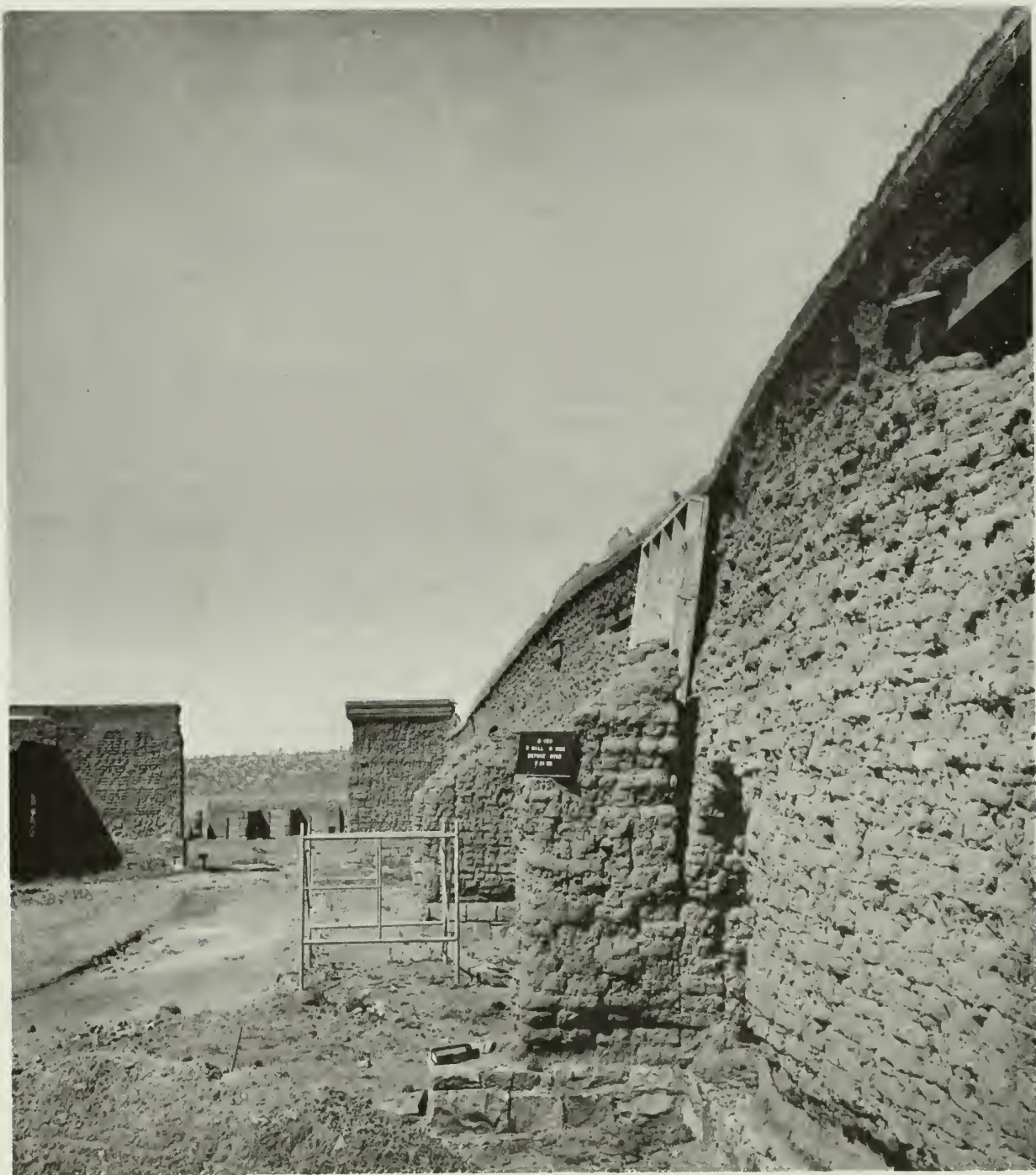
FIGURE 77. Building 3-450, Room 451, south side of south wall, before stabilization. Fort Union National Monument.
