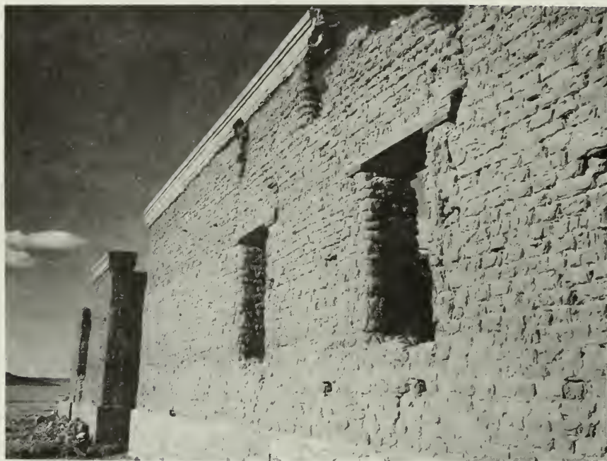
FIGURE 65. Building 3-450 (left) and building 3-440, west walls and coping, before stabilization. Fort Union National Monument.
