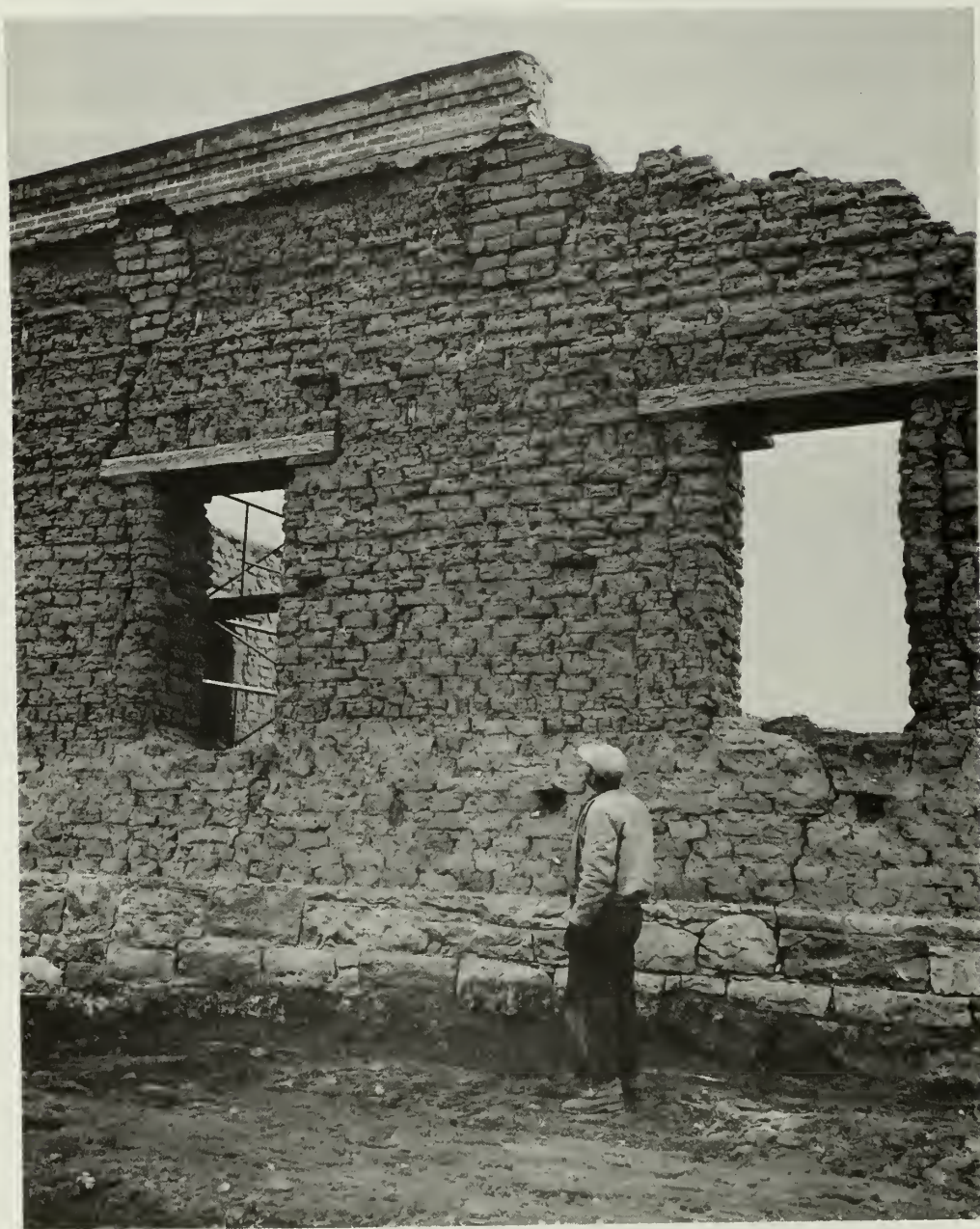
FIGURE 69. Building 3-440, west wall and coping, during stabilization. Fort Union National Monument.
