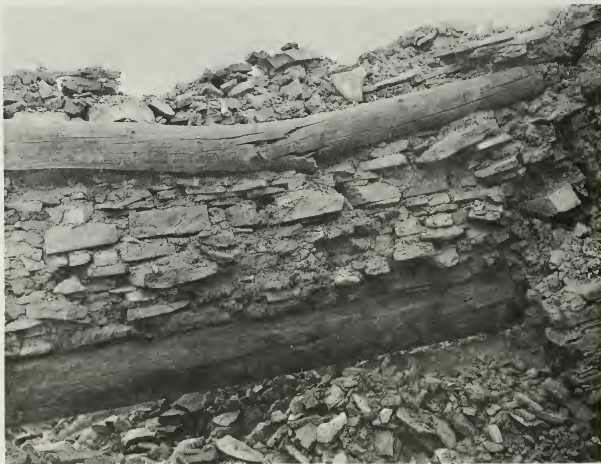
FIGURE 3. The inclusion of heavy timbers within cored-type walls was a usual practice of prehistoric builders. Collapse of walls from flood damage at Chetro Kettle exposed 300 logs similar to those above. (Chetro Kettle Ruin, Chaco Canyon National Monument, N. M.)
