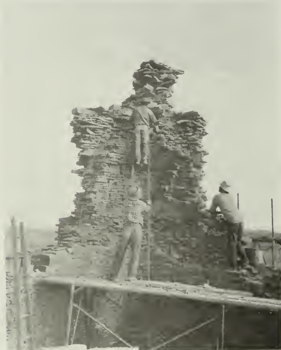
FIGURE 43. The placement of reinforcing in the third story portion of the structure shown in figure 42. The purpose is to reinforce heavily the vertical capping which will be placed up exposed ends of the wall to prevent further erosion, and to tie this part of the wall together.
