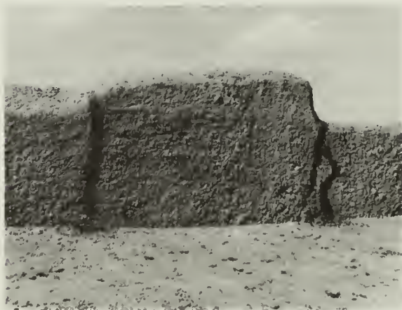
FIGURE 14. West wall of Compound A one year after the application of silicone waterproofing. Two hairline cracks were filled. The untreated smears of plaster have absorbed moisture, while the treated wall remains dry. (Casa Grande Ruins National Monument, Ariz.)
