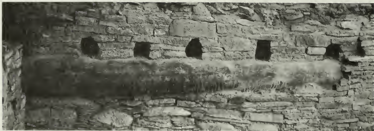
FIGURE 38. A horizontal cast log replaces the original timber which had rotted on the interior and in the embedded portions. (Chetro Kettle Ruin, Chaco Canyon National Monument, N.M.)
