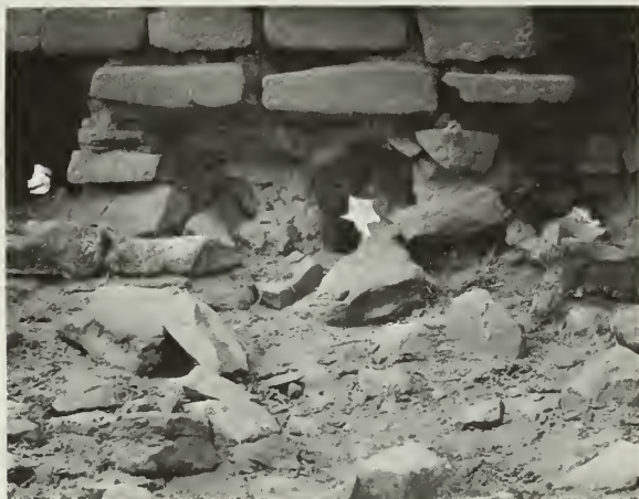
FIGURE 18. The severe undermining and basal erosion of a wall resulting from capillary moisture. If left untreated, such walls soon collapse. (West Ruin, Aztec Ruins National Monument, N. M.)
