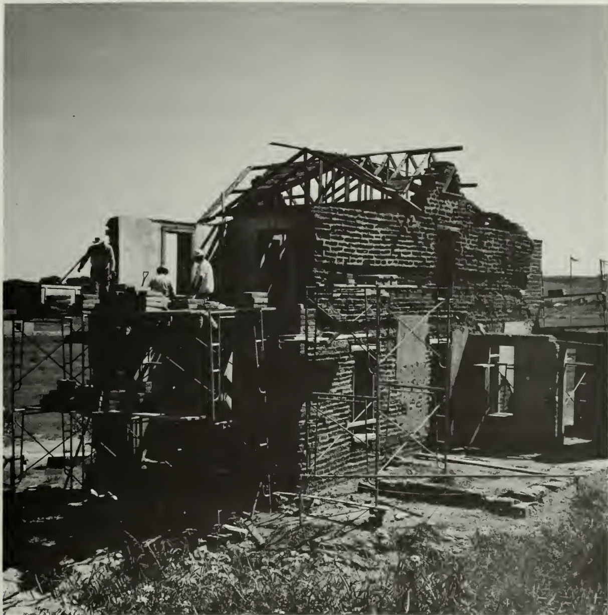
FIGURE 56. Stabilization and modified restoration in process at HB-14, shown in figure 55. Soil-cement adobes were used for repairing walls. A concealed integral bond beam was installed around the building between the first and second story levels. Concrete bearing beams were installed at roof line to support restored roof.
