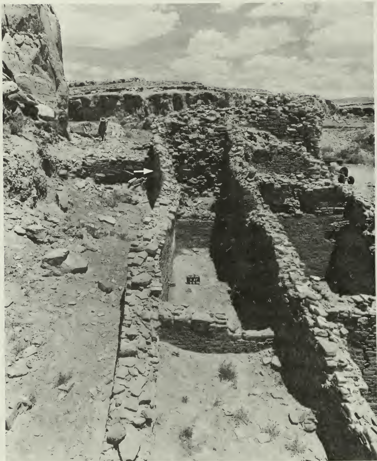
FIGURE 120. The wall between Rooms 27 and 28, Talus Unit No. 1, was distorted and pushed out of line by pressure of fill, often damp, at left. Arrow shows direction of force. The purpose of the stabilization was to strengthen the wall against the pressure.
