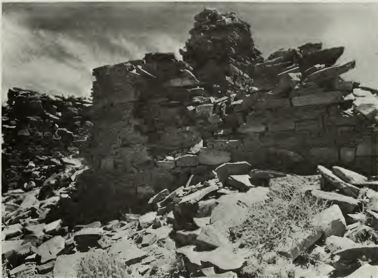
FIGURE 23. An example of soft, pecked and dimpled stone in random areas over wall surface. Replacement of the stone requires extreme care if the character of the wall is not to be changed. (Peñasco Blanco Ruin, Chaco Canyon National Monument, N. M.)
