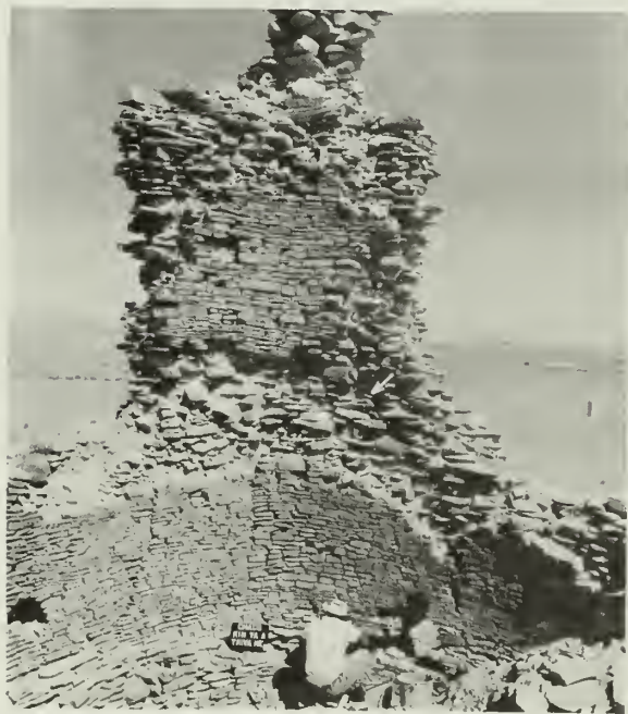
FIGURE 103. General view of northeast interior of Tower Kiva at start of project. The circular wall is stepped back or inset at two points: (1) at narrow ledge or bench where workman is beginning repairs, and (2) where facing is gone, exposing core (arrow).
