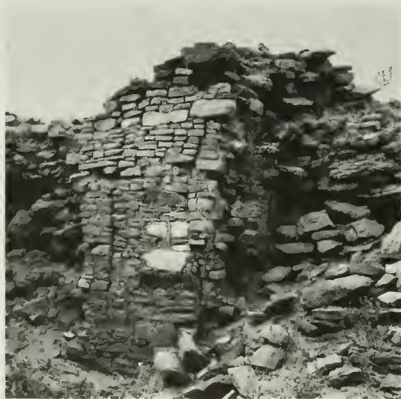
FIGURE 46. A good deal of repair masonry must be laid to fill breaks and support undercut areas in this wall at Pueblo del Arroyo. Some support must also be provided for the embedded timbers. Soil or masonry cement mortars may be used for the major part of this work. The upper courses however must be laid in concrete mortar as capping to halt further washing from the top. In this example, damage was started by surface water from adjacent, unexcavated fill and every effort should be made to prevent erosion.
