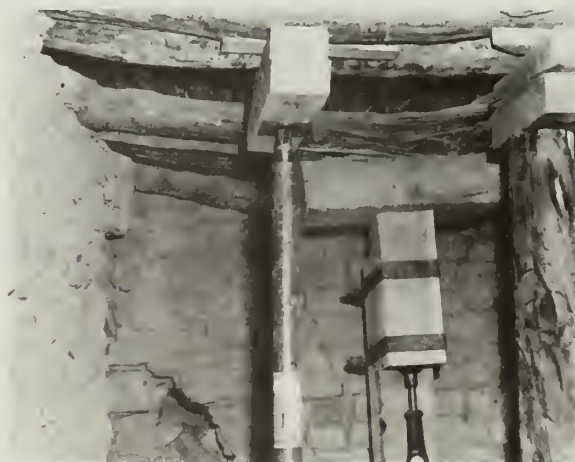
FIGURE 47. Temporary support of cracked and broken roof beams by means of jacks and timber props. Approximately 6 feet of overburden lay on this ceiling. The temporary supports were in place for several years before the overburden could be removed and a protective roofing constructed. (East Ruin, Aztec Ruins National Monument, N.M.)
