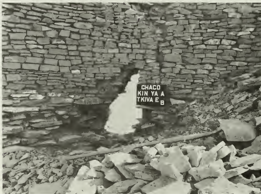
FIGURE 105. Detail of hole in Tower Kiva caused by breakdown of savino sockets. The beams for the sockets extended part way into this wall from the opposite side, and originally supported the ceiling of the adjacent room.
