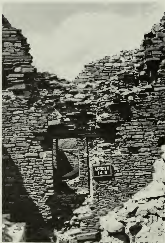
FIGURE 25. Repair at the position of the arrows will be based on a very small area in comparison with the total size of break. Every effort should be made to tie such patches securely to the existing wall. (Pueblo del Arroyo Ruin, Room 14, north wall, Chaco Canyon National Monument, N. M.)
