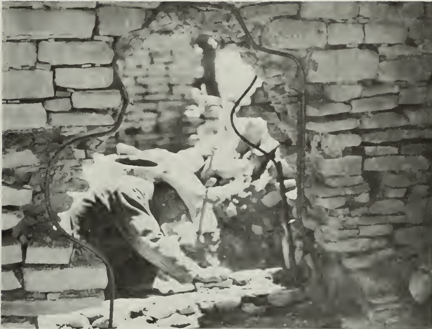
FIGURE 39. Integral members. Starting a reinforced arch section, rods have been bent to fit the contours of the break and are wired in place. The workman is laying the courses across the bottom of the break in concrete mortar to provide a solid base for the reinforced section. Above this level, masonry on the perimeter of the hole will be laid in concrete mortar which will also surround the steel rods. Masonry in the center of the hole will be laid dry or with a minimum of soil mortar; its only function will be to support masonry laid in cement until the latter has set. This dry masonry will then be removed. (Pueblo Alto, Chaco Canyon National Monument, N. M.)
