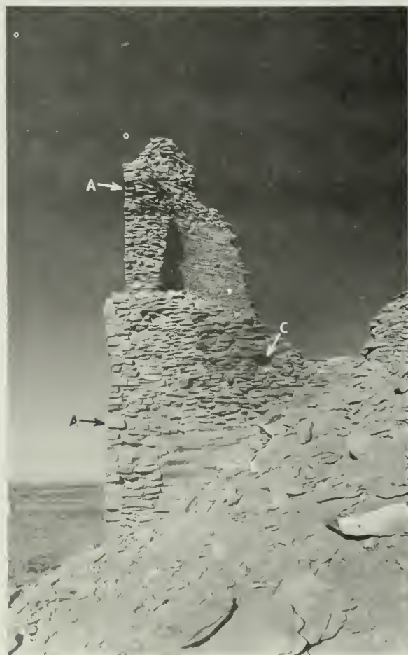
FIGURE 116. North wall stub capped (arrows A), lower portion of west wall facing reset (B), and exposed portion of thick core grouted (C).
