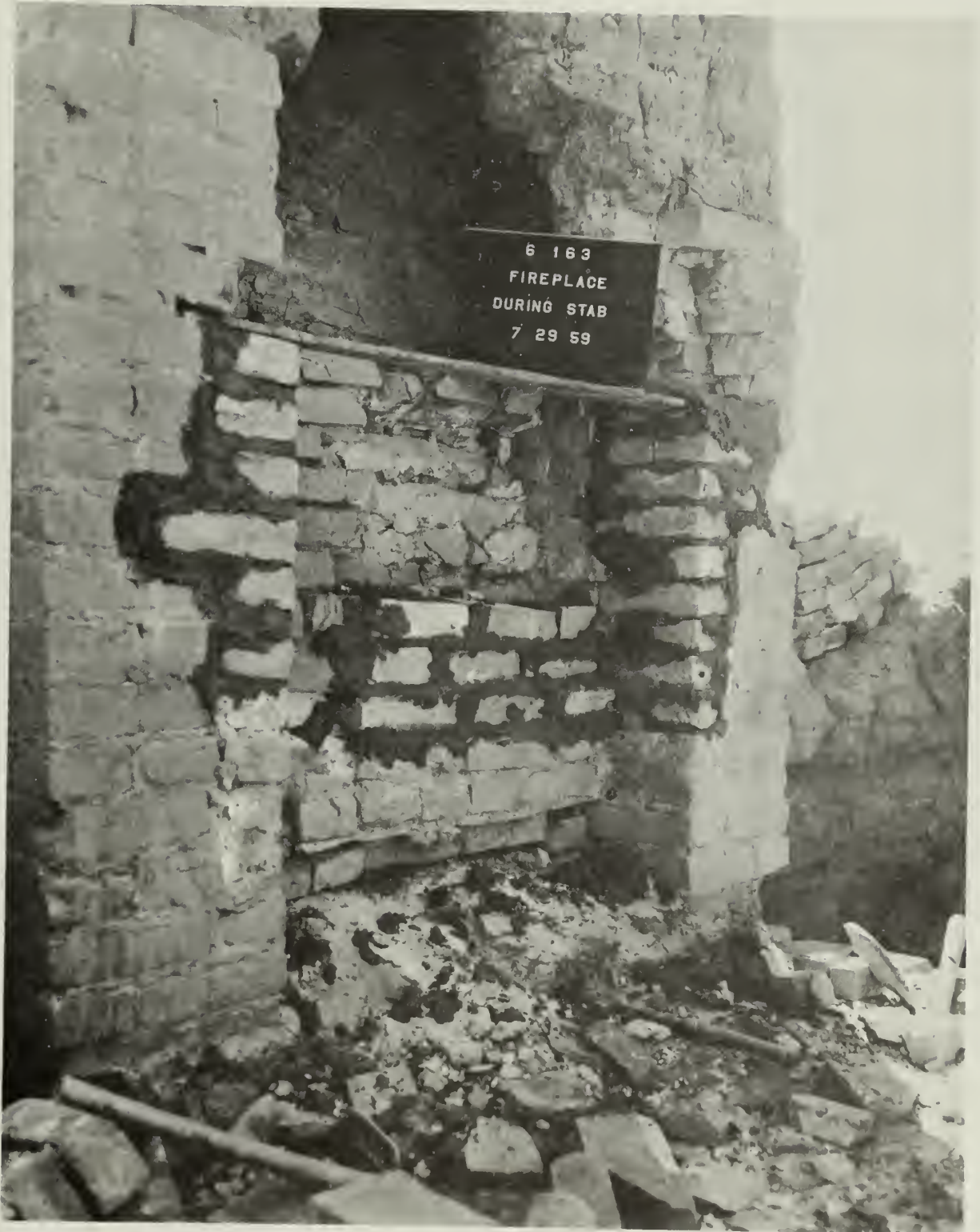
FIGURE 94. Building 6-160, Room 163, fireplace in east wall, during stabilization. Historic bricks are being reset in soil-cement mortar. Fort Union National Monument.
