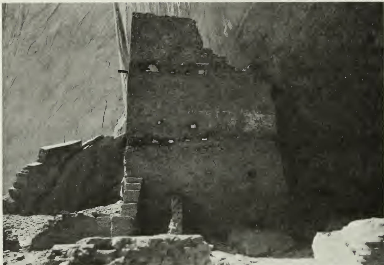
FIGURE 1. Settling caused by lack of foundations and unstable fill. Bond between stone and soil mortar is poor. Holes are caused by decay or theft of wood members. (Antelope House Ruin, Canyon de Chelly National Monument, Ariz.)
