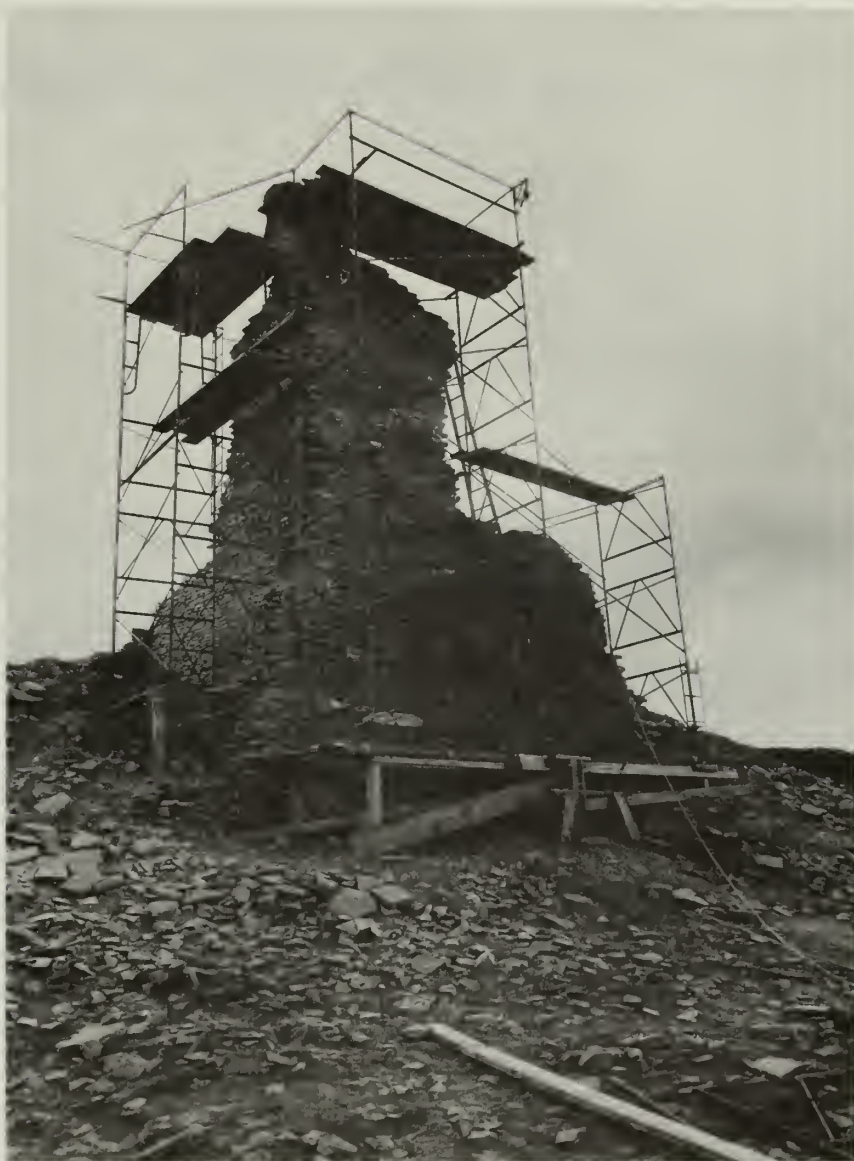
FIGURE 119. Tower Kiva. Scaffolding was anchored on firm and level bases built of heavy timbers.
