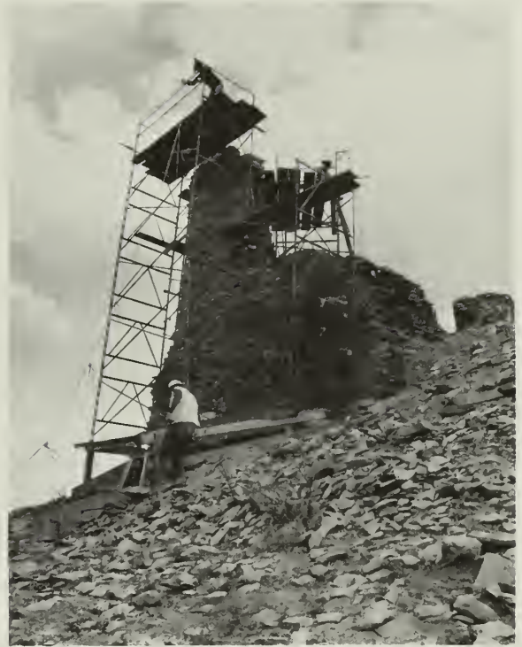
FIGURE 42. Reinforced integral members are important in the stabilization of spirelike structures such as this at the Tower Kiva, Kin Ya-a Ruin, Chaco Canyon National Monument, N. M. Considerable strength must be added without serious or objectionable alterations of the original profile.
