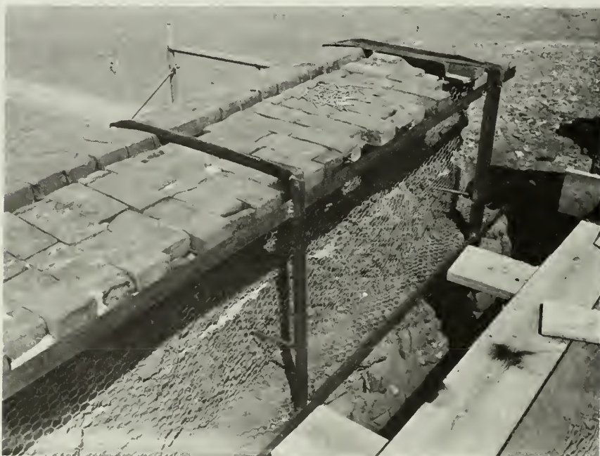
FIGURE 66. Building 3-440, coping on west wall, during stabilization, Fort Union National Monument.
