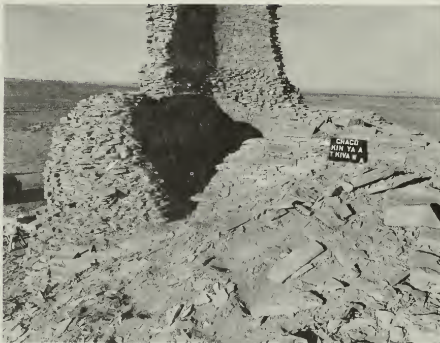
FIGURE 117. Tower Kiva, west wall. This fragmentary section of the square tower enclosing a round one was repaired by resetting the facing (arrow A), capping and grouting the thick core (B).
