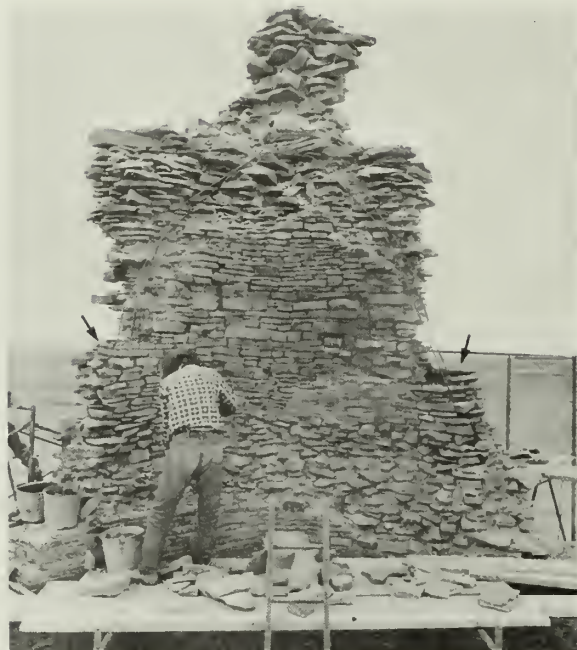
FIGURE 109. Beginning the vertical, reinforced capping (arrows).
