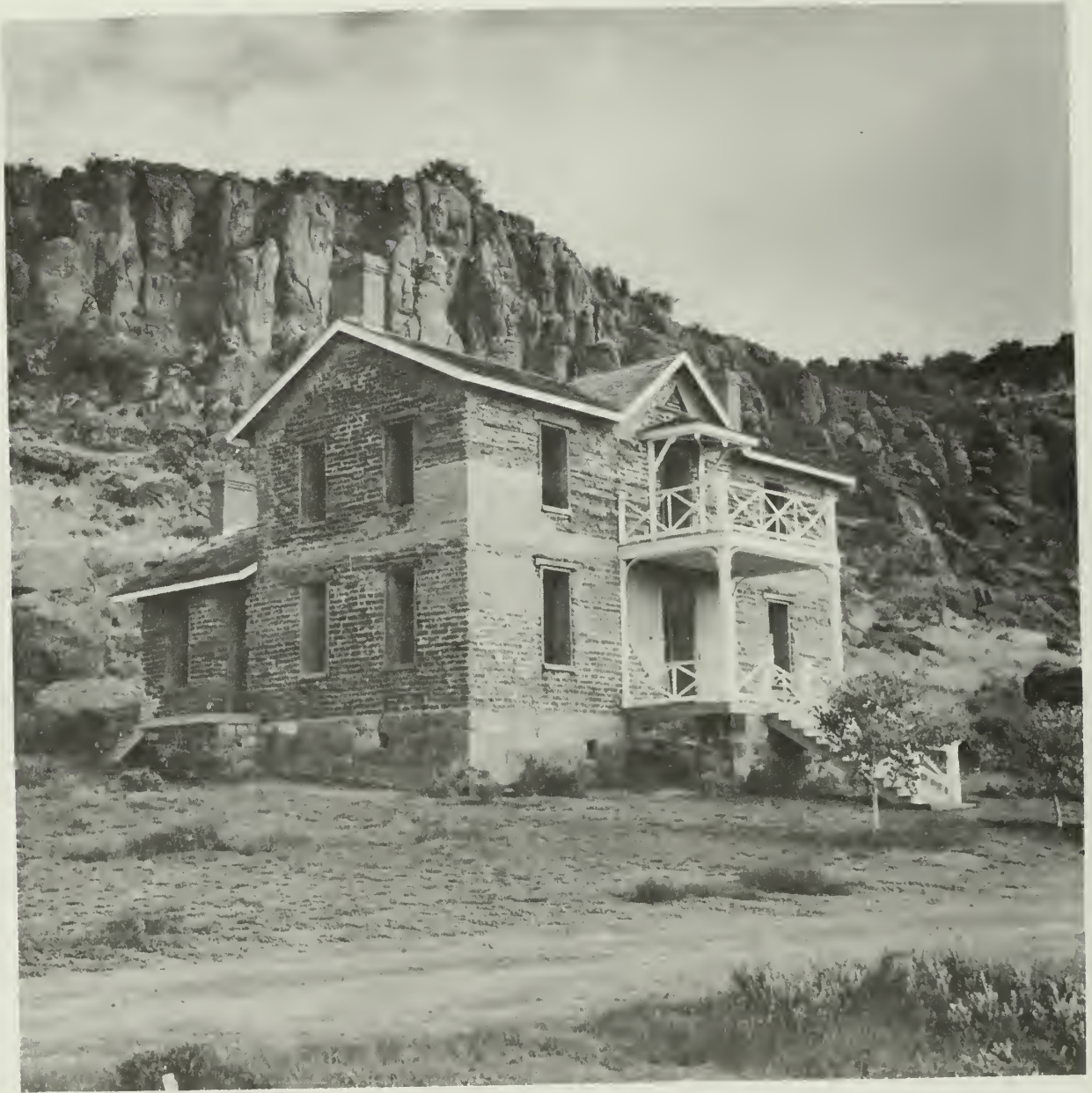
FIGURE 57. The completed stabilization and modified restoration of building HB-14, Fort Davis National Historic Site. Compare with figures 55 and 56.
