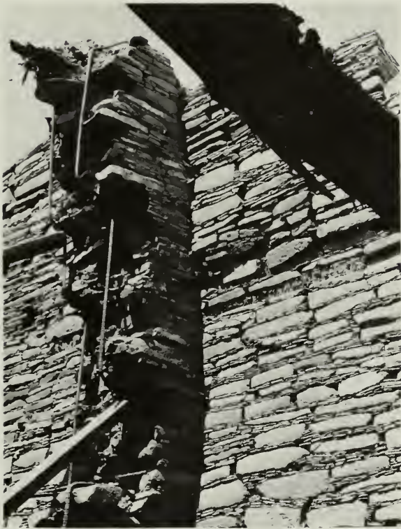
FIGURE 41. Integral members; steel in place for a narrow vertical section. The steel must be tied in securely to the cross wall at the top to provide support for the overhanging area. Some support will be required for the vertical strip of masonry as it is being laid, and until the concrete mortar has set. (Chetro Kettle Ruin, Chaco Canyon National Monument.)
