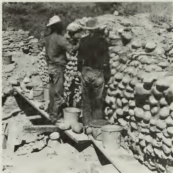
FIGURE 26. Deep grouting with soil-cement on the badly weathered face of this cobblestone wall will not change its appearance, but will halt the rapid rate of erosion. (East Ruin, Aztec Ruins National Monument, N. M.)
