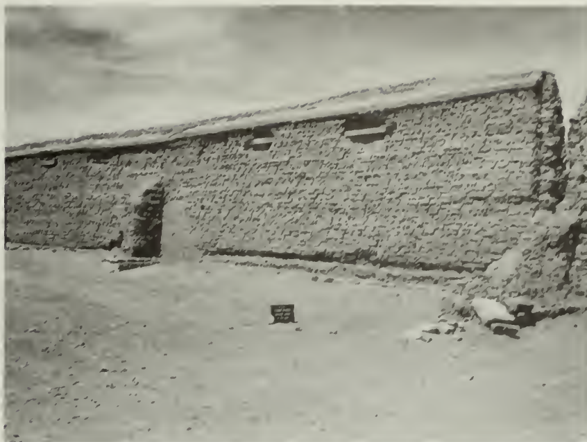
FIGURE 81. Building 3-450, Room 451, south side of south wall, after stabilization. Fort Union National Monument.
