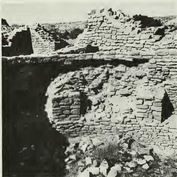
FIGURE 15. Damage caused by outward movement of moisture from fill behind kiva wall. The most severe disintegration is at the limit of capillary rise, just below the concrete capping. (Clan Kiva, West Ruin, Aztec Ruins National Monument, N. M.)
