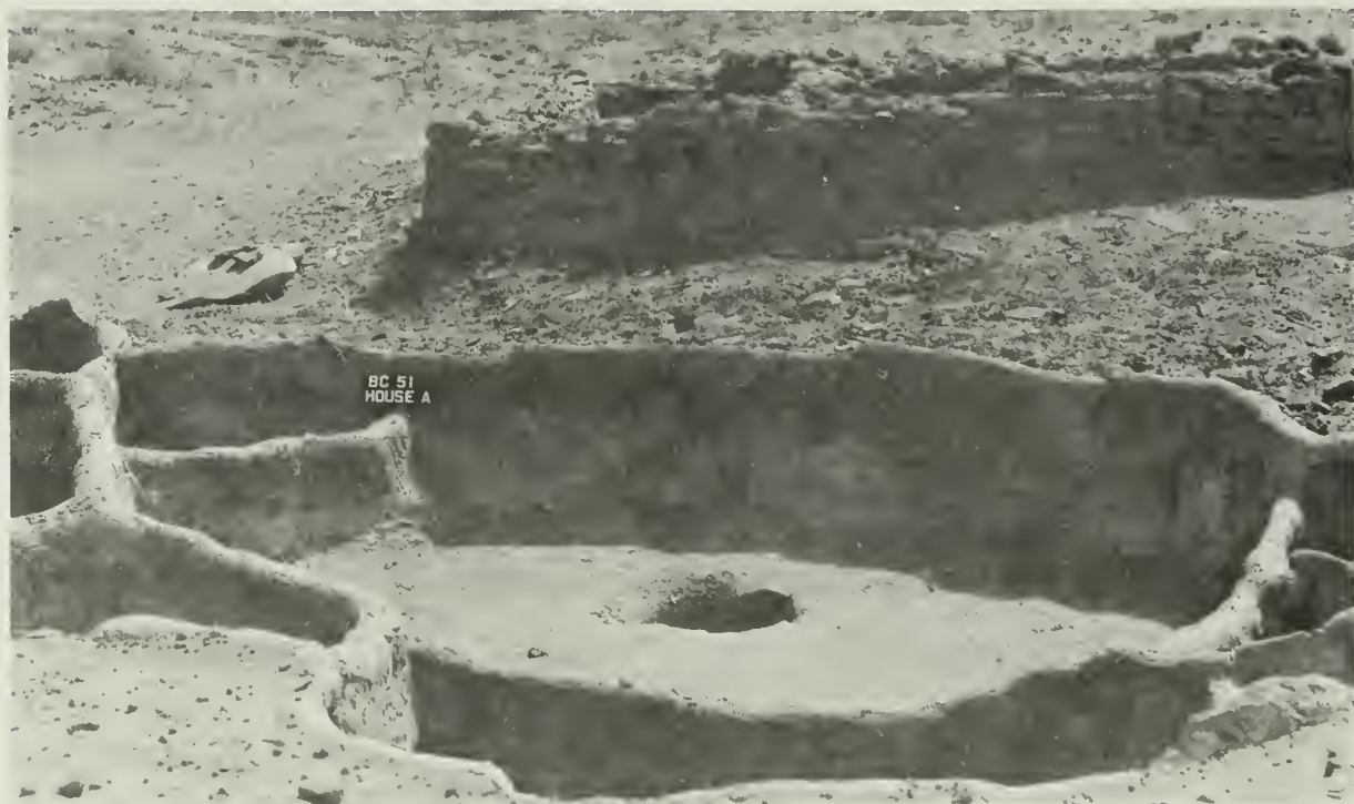
FIGURE 9. Soil-cement in heavy cross section; shown here for the repair of slab-house walls. (Basket Maker III pithouse, Site Bc-51, Chaco Canyon National Monument, N. M.)
