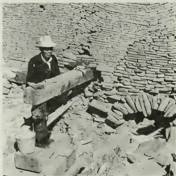
FIGURE 28. The temporary support of a heavy wall with timber. The arch at lower right was constructed in the 1920's as a repair measure. The first step in stabilization involved the placing of a beam through a hole adjacent to the arch. Not of aboriginal origin, the arch was subsequently removed. (Room 1, Chetro Kettle Ruin, Chaco Canyon National Monument, N. M.)
