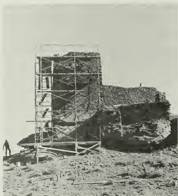
FIGURE 27. Scaffolding in place at completion of respalling and grouting large wall surfaces. (Wukoki Ruin, Wupatki National Monument, Ariz.)
