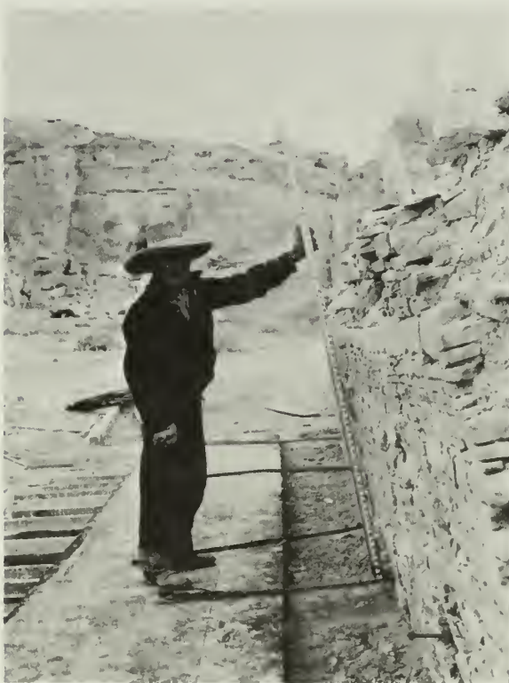
FIGURE 33. Beginning realignment. Cables have been placed through the base of the wall to be tied to the jacks. Note bolt, lower right, for holding frame against wall. (Pueblo Bonito, Chaco Canyon National Monument, N. M.)
