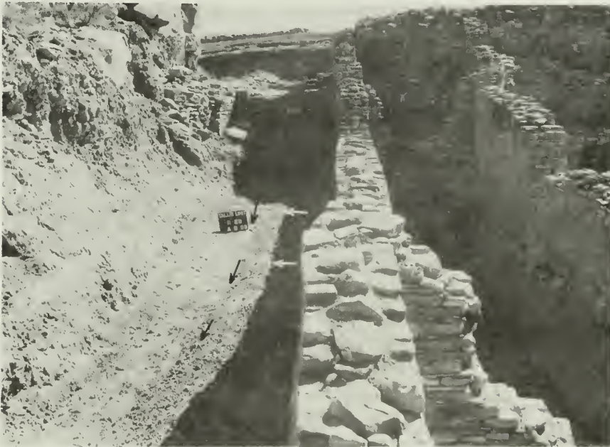
FIGURE 123. This wall in Talus Unit No. 1 has been pulled back into line; the capping is straightened up. The concrete beam dug into Room 28 is covered and the surface of this room (arrows) is graded to carry surface runoff away from the damaged wall.
