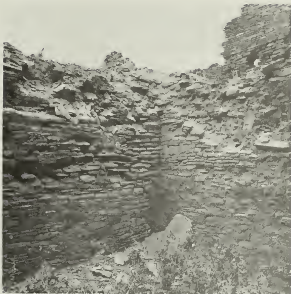
FIGURE 44. In many cases such as that depicted above it will be difficult to draw a distinction between general wall repairs and capping. This wall will have to be carried up to the level of the outside fill to prevent further washing over the top. Whatever type of mortar is used for such wall repairs, the top courses must be set in a cement mortar to provide as durable and waterproof a cap as possible. (Pueblo del Arroyo, Chaco Canyon National Monument, N.M.)
