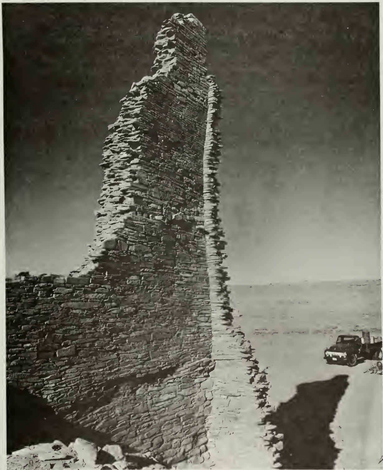
FIGURE 114. View of Tower Kiva showing north wall stub buttressed, cracks repaired, savino sockets re-molded, and facing grouted.
