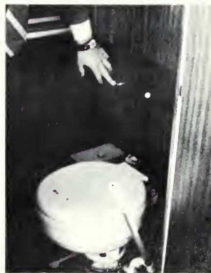
Top: Gaddis inspects a treatment device which uses an ammonium compound to break down wastes. This model, the Raritan Crown Head, is considered one of the best devices available.
