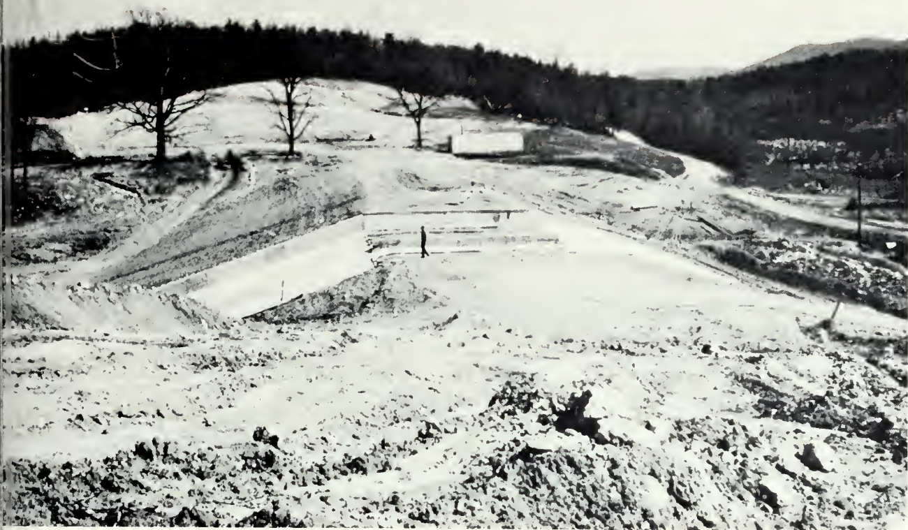
he area to the right of this dam, now under construction, will be covered by a 40-acre lake. The road in the picture will be replaced by a road over the dam. The dam at the future site of the Chattooga County Public Fishing Area is 202 feet wide and 100 feet long with a 100-foot spillway. (Photo by Ted Borg)
