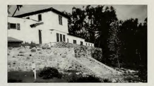
Figure 23. View of the north side of the clubhouses showing new terrace and stairway built by the CCC, 1935. The new features are in the foreground and the original wall and steps constructed in 1928 are of the darker stone behind the new steps. (NARA, RG79.)
