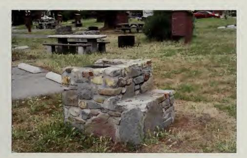
Figure 59. View of one of the stone cook stoves featuring a blocky design with vertical sides and a pot ledge on the back. (OCLP 2009.)
