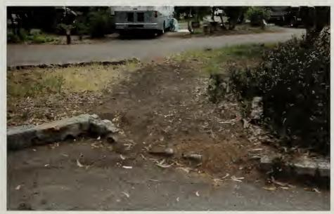
Figure 78. View of curb damage at the southern end of the campground. (OCLP 2009.)
