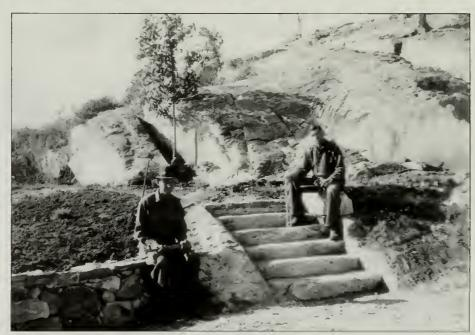
Figure 22. View of the stone retaining walls (seen in the left foreground) and steps carved out of a cleft in the rock in the clubhouse parking area, south of the clubhouse, 1935. (NARA, RG79.)
