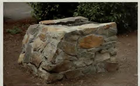
Figure 58. View of one of the stone cook stoves showing one of several designs within the campground featuring a battered rear elevation and a flush top. (OCLP 2009.)
