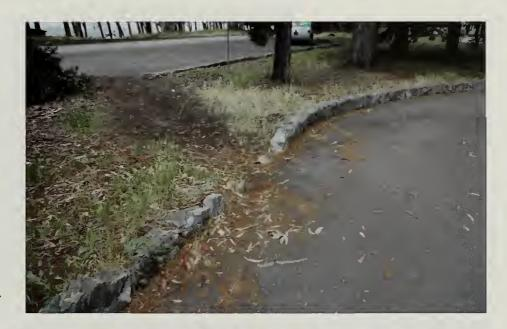
Figure 77. Repair and preserve stone curbs. Place natural objects and vegetation as barriers to prevent pedestrian crossing or provide a more formalized crossing. (OCLP 2009.)
