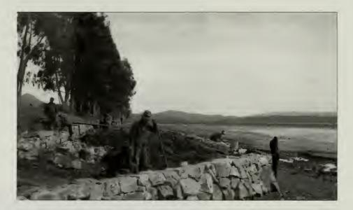
Figure 18. View of construction of the retaining walls at the beachfront picnic area, 1935. (NARA, RG79.)
