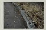
Figure 55. View of the stone curb at the southern end of the campground. The stone curbs originally lined the campground entrance road, as well as the parking on State Park Road and the walkways around Combination Building #1. (OCLP 2009.)
