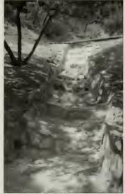
Figure 15. View of stone-lined spillway in Chorro Creek, 1934. Flood and erosion control also included the construction of stone and earth dams and the channelization of Chorro Creek. (NARA, RG79.)
