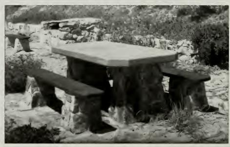
Figure 19. View of one of the picnic table designs constructed at the beach-front picnic area, 1935. The table featured a stone base with a rectangular concrete top and wooden seats. (NARA, RG79.)
