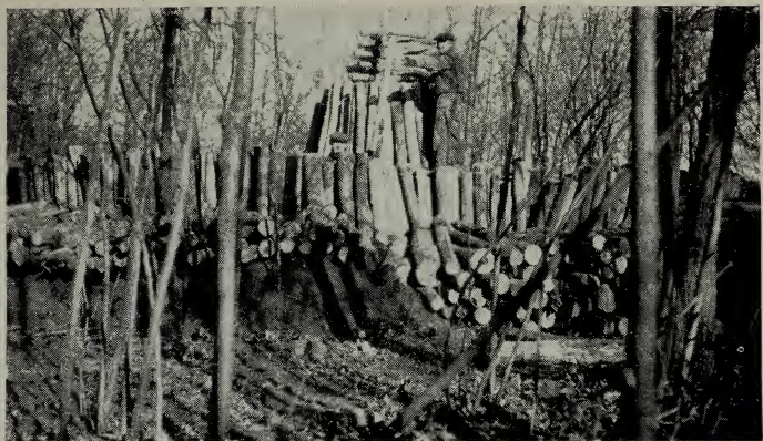
Constructing the chimney
