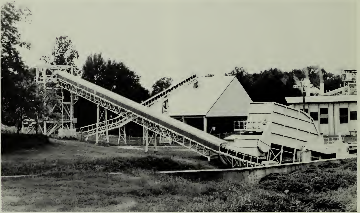
This recently completed wood heating complex at Central State Hospital is an example of the dramatic increase in the use of wood as fuel. The system is designed to burn wood chips that provides steam for heating, cooling and domestic hot water for numerous buildings at the institution.
