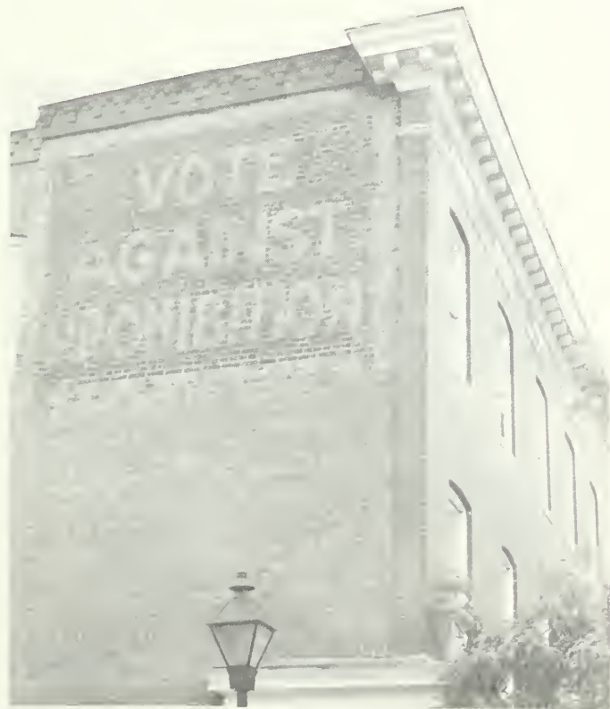
10. This fading sign was painted in Baltimore in 1931 or 1932. It survives from the campaign to enact the 21st Amendment to the United States Constitution, which repealed Prohibition. Such fading brick wall signs are known as "ghost signs." Photo: Thomas C. Jester.
