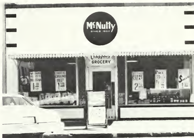
7. In the 1930s and 1940s, signs built into storefronts became popular. This example is from Guthrie, Oklahoma. Photo: H. Ward Jandl.
