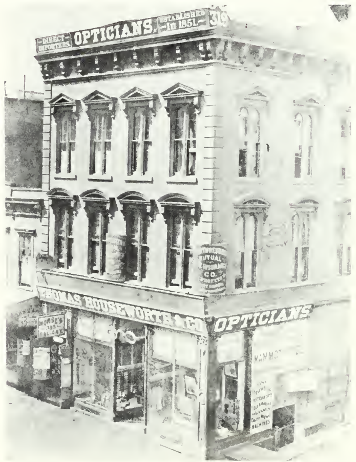
4. This circa 1866 view of a San Francisco building shows the range of signs used in the nineteenth century: Symbolic signs (the spectacles over the entrance); fascia signs; plaques, often in the shape of shields and normally used by insurance companies, in part to symbolize the protective function of insurance; posters, wall signs, window signs, hanging signs, and rooftop signs. Photo: Library of Congress.
