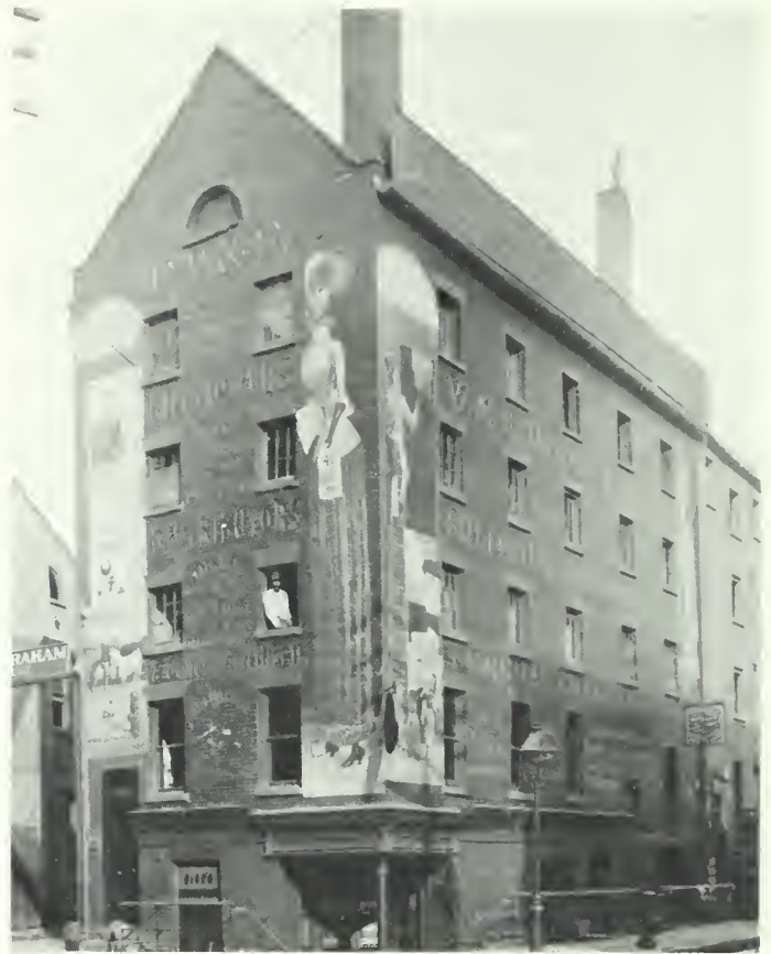
5. Painted figures and lines of text cover this building in New York City, about 1890. The woman is distributing handbills. The painted workman on the ladder is putting up a poster. Altogether the signs are striking examples of the signmaker's art in the late nineteenth century. Photo: Courtesy of the New-York Historical Society, New York City.
