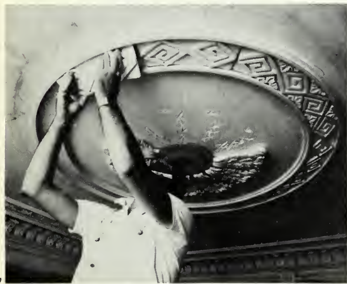
Fig. 7. Running and Enriching a Ceiling Medallion. The method of running and enriching a ceiling medallion remains the same today. (a) First, a plain-run surround is spun from a pivot point centered in the ceiling field. (b) Ornament layout is determined using plane geometric principles; segmented locations are deeply scratched to provide a rough surface for adequate bonding using plaster as an adhesive. Historically, cast enrichments could be bought from local suppliers and set individually, allowing architects to compose medallions to suit room dimensions and period motifs. Photos: Peter Sanders.
