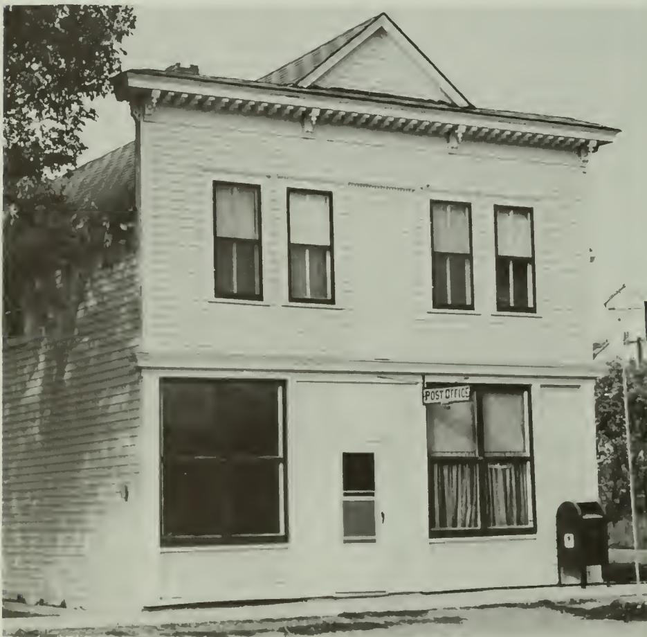
Post Office, Christine, North Dakota, c. 1895. This building is a good example of the vernacular "Boomtown" architecture typical of North Dakota's earliest years of white settlement. Originally constructed as a residence and commercial establishment, this became a post office in 1923 after Charles Hanson, a prominent local educator, became postmaster and lived with his family in the rear portion.
