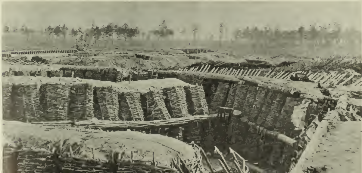
Trenches used by the Confederates in the defense of Petersburg. Note the use of rolls of wickerwork, or gabions, to line the sides of the trenches. Courtesy Signal Corps, U. S. Army.
