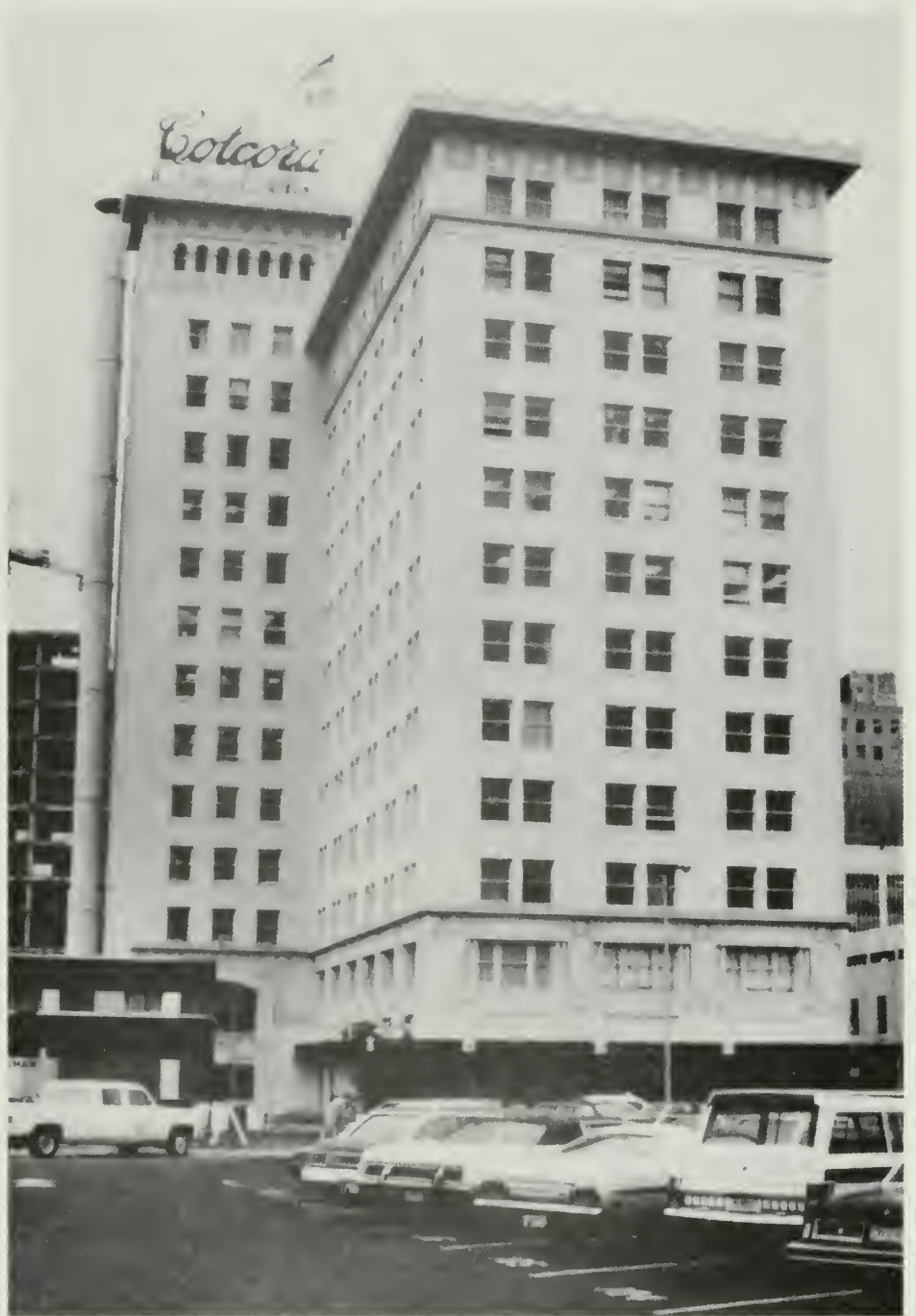
Figure 1. The Colcord Building, Oklahoma City, Oklahoma. This 12-story poured-in-place concrete building with terra-cotta ornamentation was built in 1910 and is individually listed on the National Register of Historic Places. (Photo: H. Ward Jandl)
