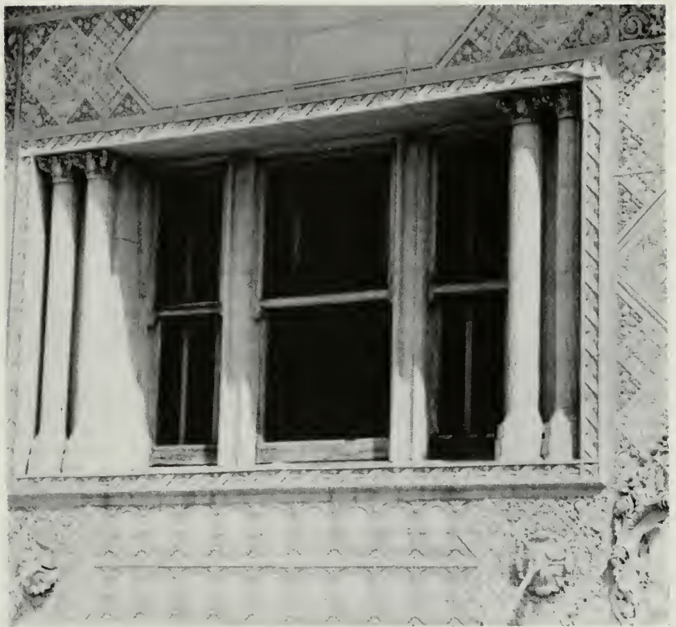
Figure 2. Original second-floor wooden windows of the Colcord Building. Note the high degree of ornamentation with the composition of the triple windows, the deep setbacks, the paired Corinthian columns, and the Sullivanesque terra-cotta panels surrounding the windows. The windows on the upper floors are of a simpler composition being paired one-over-one double-hung windows. (Photo: Jack Graves, AIA)
