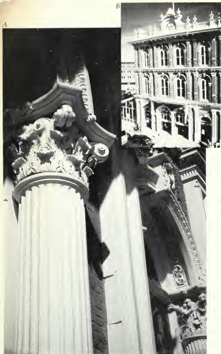
Fig. 19. (a) Fiberglass columns and aluminum capitals were installed to replicate the ornamental features on the east facade of the New Market Theater in Portland, Oregon, that had been destroyed by previous occupants. Like cast iron, crisp ornamental details can be achieved with cast aluminum. Although aluminum may be in contact with fiberglass, galvanic corrosion may result when aluminum is in direct contact with cast iron. Photo: William J. Hawkins, III. (b) The west facade of the theatre retains its original cast iron features. Photo: George McMath.
