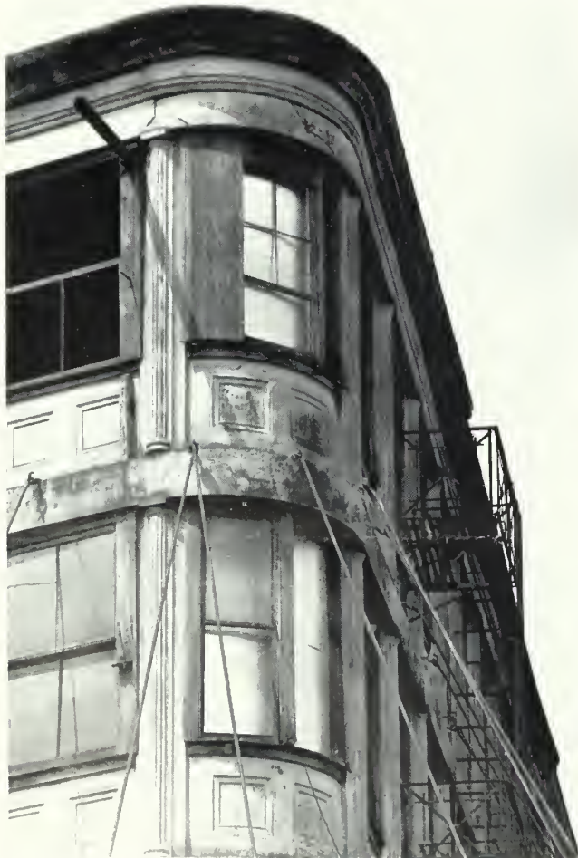
Fig. 2. The Edgar Laing Stores Block in New York City was designed by James Bogardus. It was the first building constructed with facades of self-supporting cast iron. This corner view shows the Doric-style engaged columns, panels, and spandrel beams; the loss of most of the original ornamental castings give it an austere look. As part of an urban renewal project, the facades were carefully disassembled in 1971 for later re-creation in another location—only to have its iron parts stolen for scrap. Photo: Jack E. Boucher, HABS Collection.
