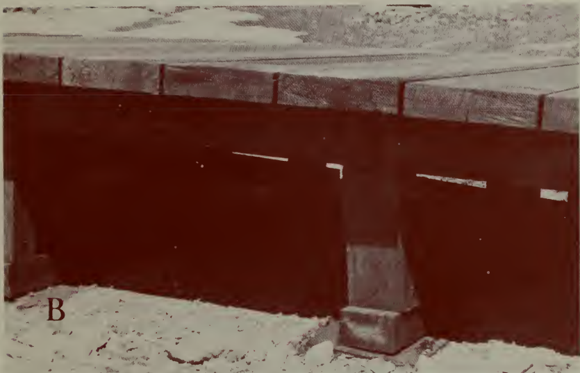
FIGURE 2. (A) Study area along wooden walkway, Logan Pass, Glacier National Park, showing: a. affected area south of walkway, b. affected area north of walkway, c. unaffected control area. (B) Construction details of wooden walkway showing dark colored, heavily treated lumber.
