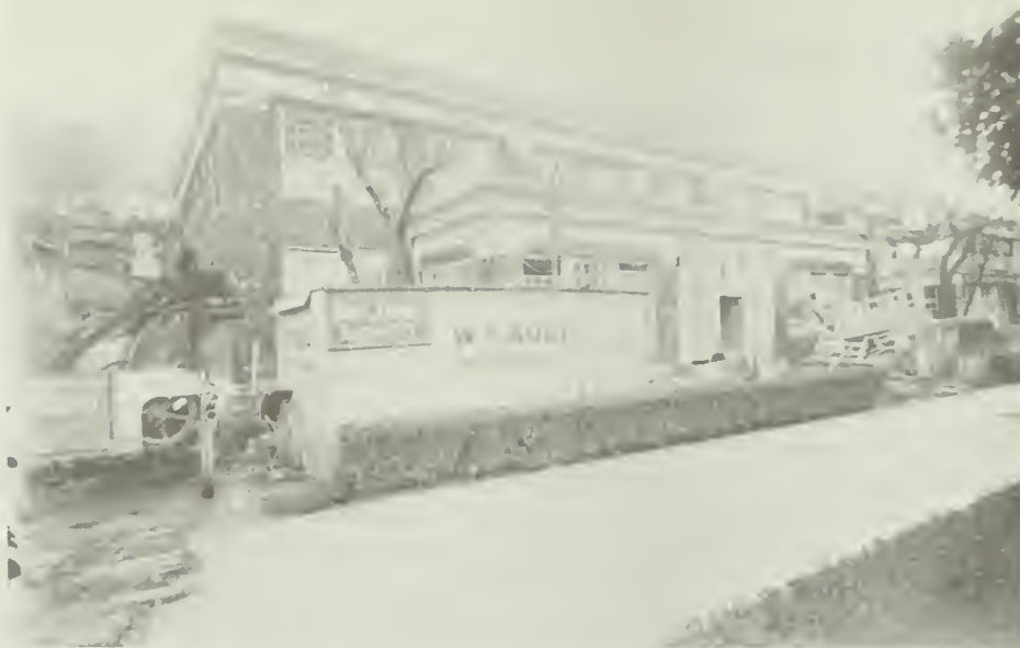
Figure 6: Superior Bathhouse under Construction, 1915-1916 (Source: Hot Springs National Park)
