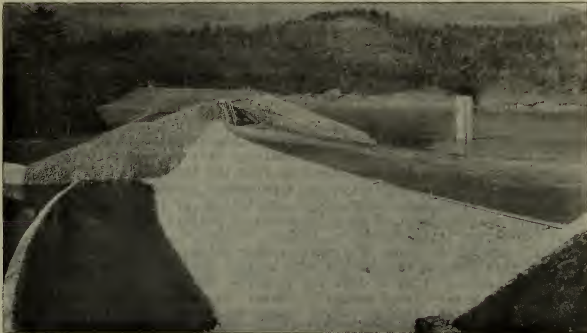
EARTH DAM AND SPILLWAY AT DOUTHAT STATE PARK, VIRGINIA Containing Nearly 200,000 Cubic Yards of Fill, This is the Largest Earth Dam Built by CCC Enrollees in Region One
