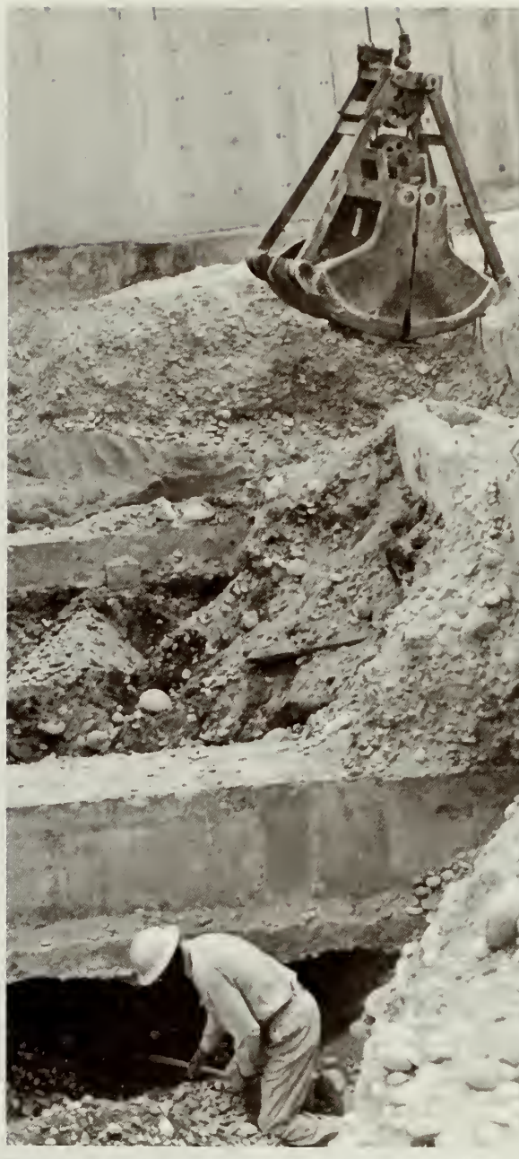
Clearing for a water line to cool reactor during deactivation.
