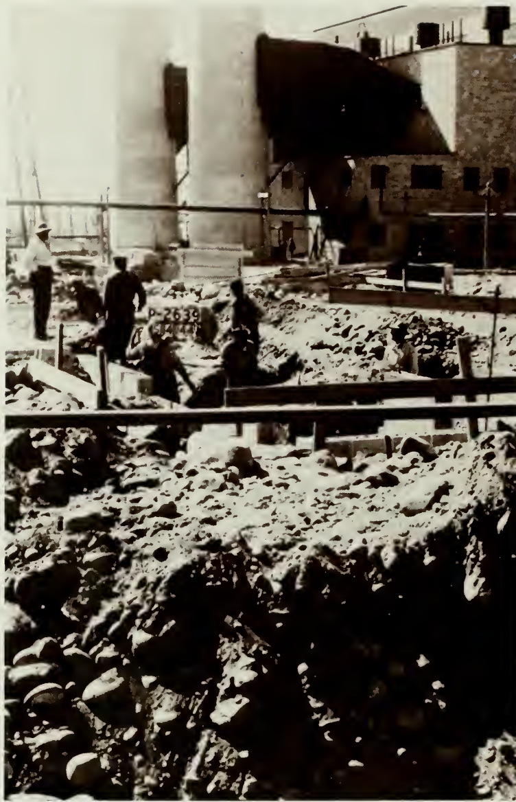
Powerhouse under construction, 1944.
