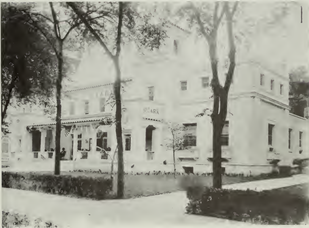
Figure 9: Ozark Bathhouse, 1922 (Source: National Archives, Natural Resources Division, RG 79)
