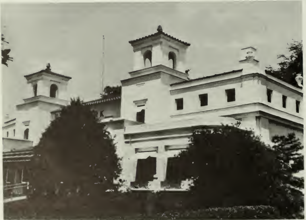
Figure 14: Ozark Bathhouse with Metal Awnings, after 1951 (Source: Hot Springs National Park)
