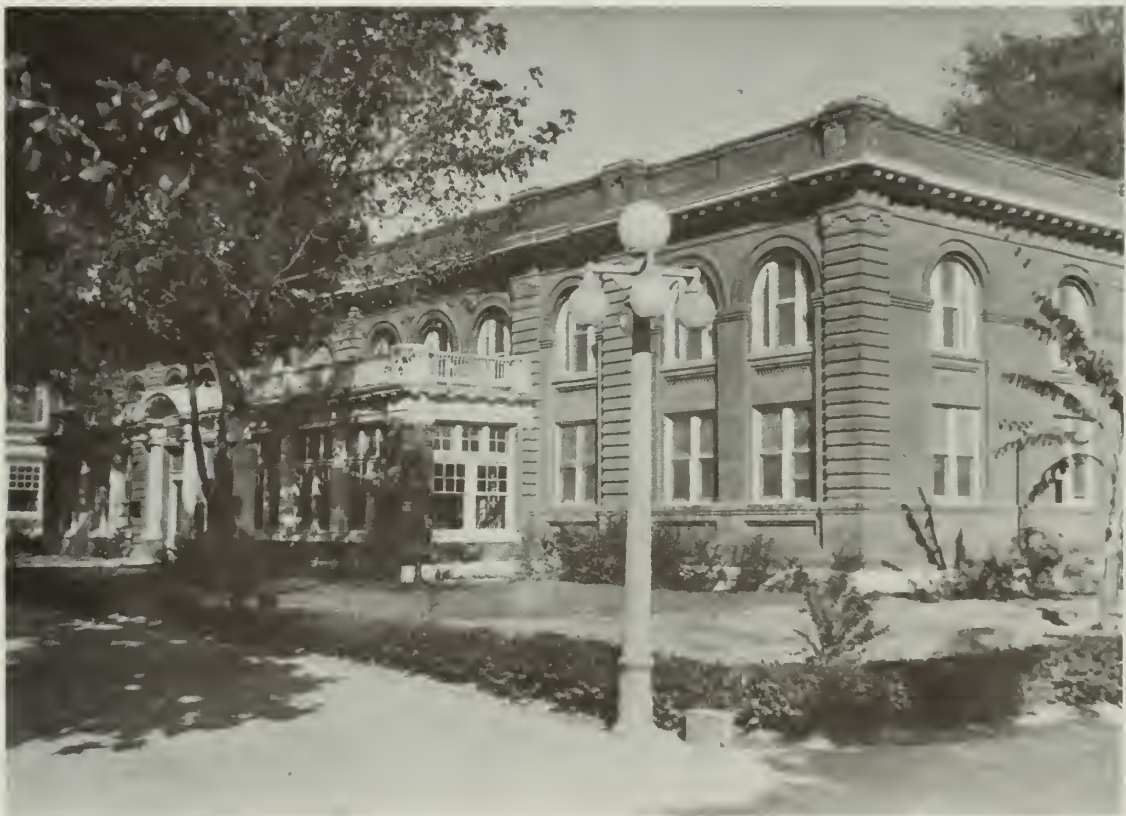
Figure 15: Hale Bathhouse, between 1915 and 1937 (Source: Hot Springs National Park)
