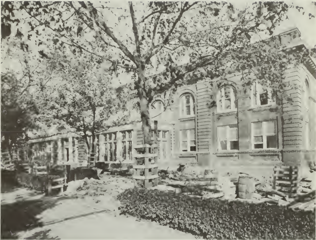
Figure 11: The Exterior of the Hale during Remodeling, 1914 (Source: National Archives, Natural Resources Division, R.G. 79)
