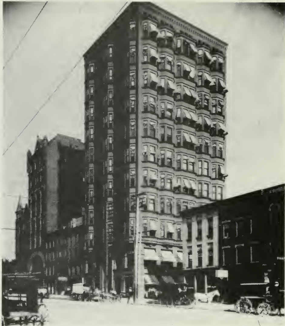
Fig. 10. The Wyandotte Building about the turn of the century. It was the first steel skelton-frame structure built in Columbus. Note the awnings, an early energy saving device. (Courtesy of the Ohio Historical Society)
