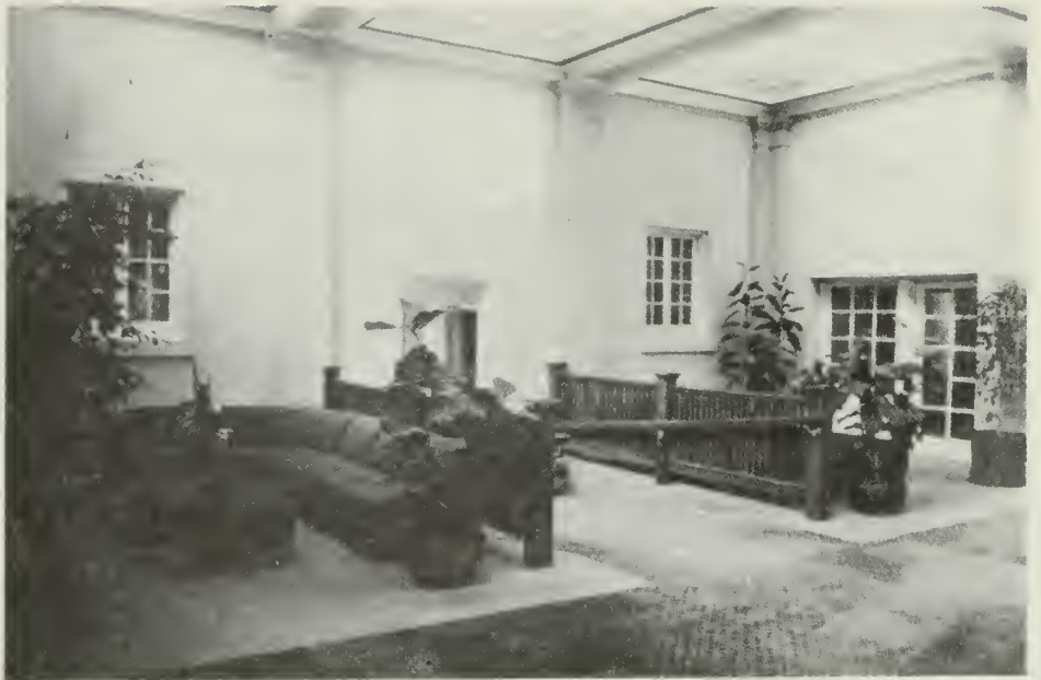
Fig. 8. The courtyard after rehabilitation. The original pilasters and skylight have been revealed after removal of the suspended acoustical ceiling. The wheelchair access ramp was installed as part of the rehabilitation. (Courtesy of John Powell, The Klein Group)
