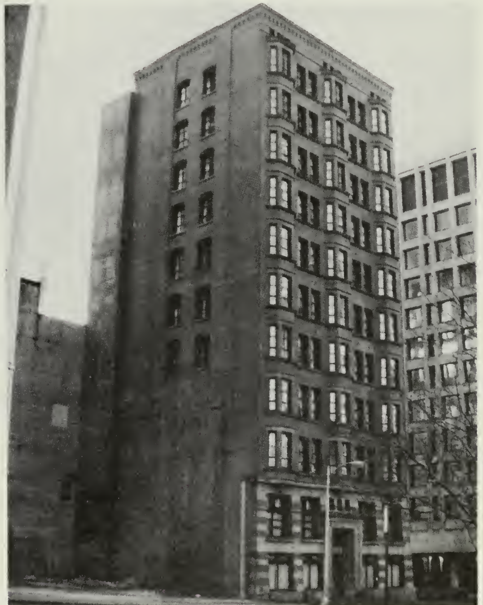
Fig. 12. The Wyandotte after rehabilitation. The new stair tower addition is at the left. (Courtesy of Judith Kitchen, Ohio Historic Preservation Office)
