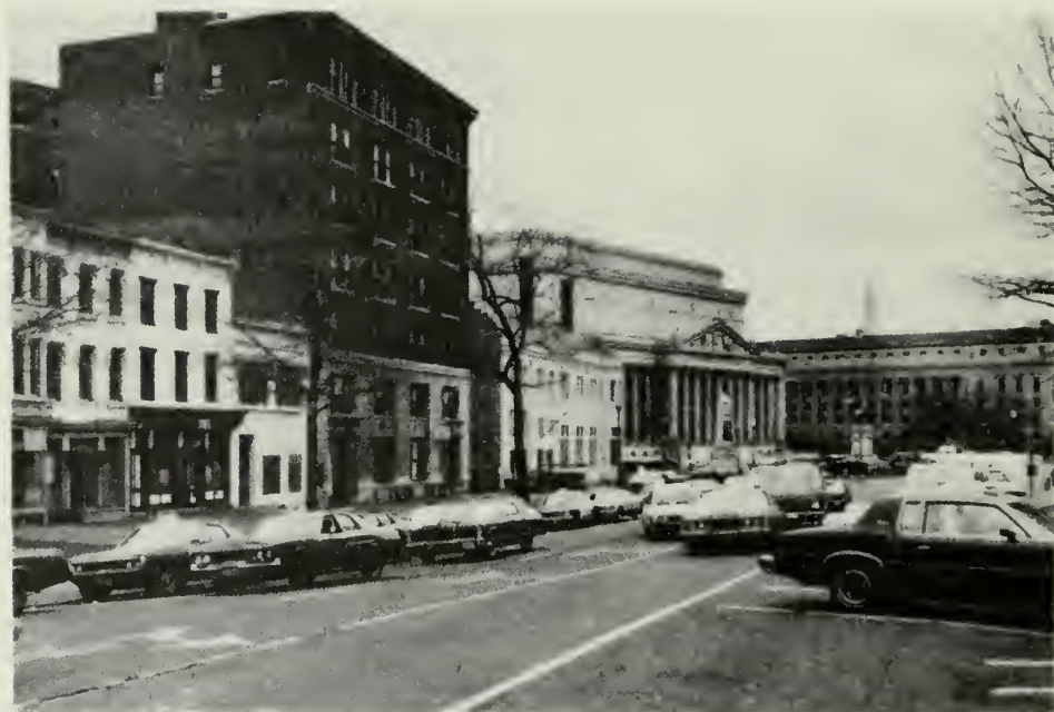
Fig. 1. This row of historic office buildings in Washington, D.C., is conveniently located near the Archives of the United States (right center) and other federal office buildings. (Courtesy of Bill MacRostie, Technical Preservation Services)
