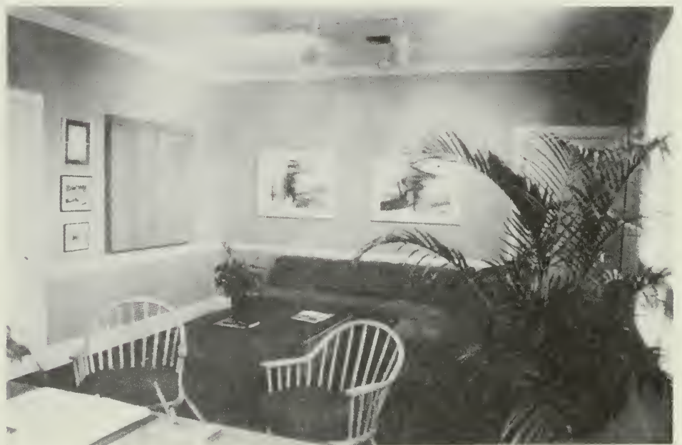
Fig. 9. Lowered ceilings in the perimeter offices were removed in the rehabilitation, restoring the ceilings to their original height. (Courtesy of John Powell, The Klein Group)
