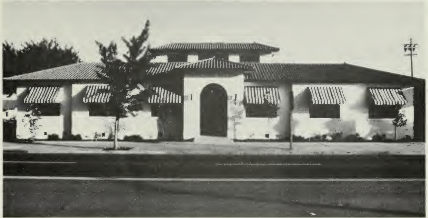
Fig. 6. The Physicians Building after rehabilitation with new awnings in place replicating the originals. (Courtesy of John Powell, The Klein Group)
