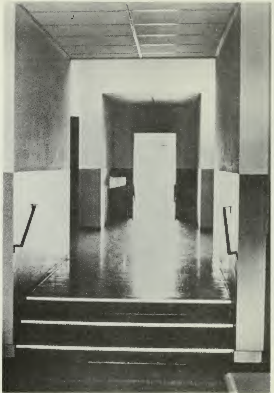
Fig. 5. The courtyard space with 1968 partitions and lowered ceilings. These non-original features were removed in the rehabilitation. (Courtesy of The Klein Group)
