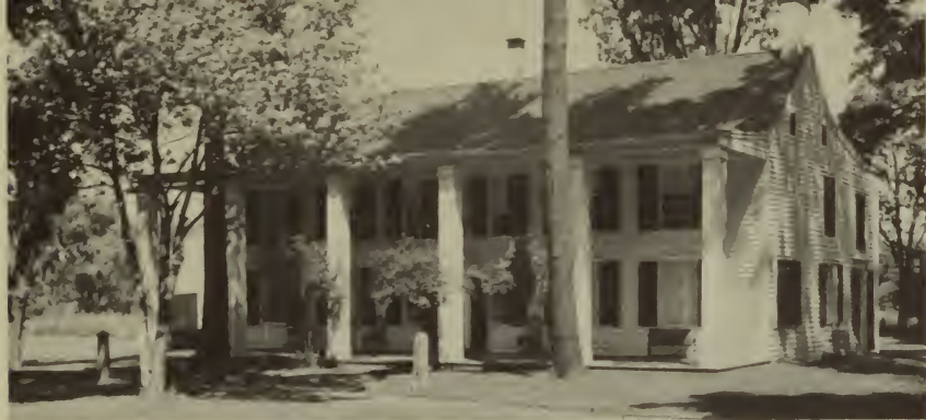
The Schuyler House. The main part of this building was erected by Gen. Philip Schuyler to replace an earlier house, which was burned by Burgoyne's troops on October 10, 1777. The house, situated in Schuylerville (Old Saratoga), is being restored to the period of Schuyler family occupancy.
