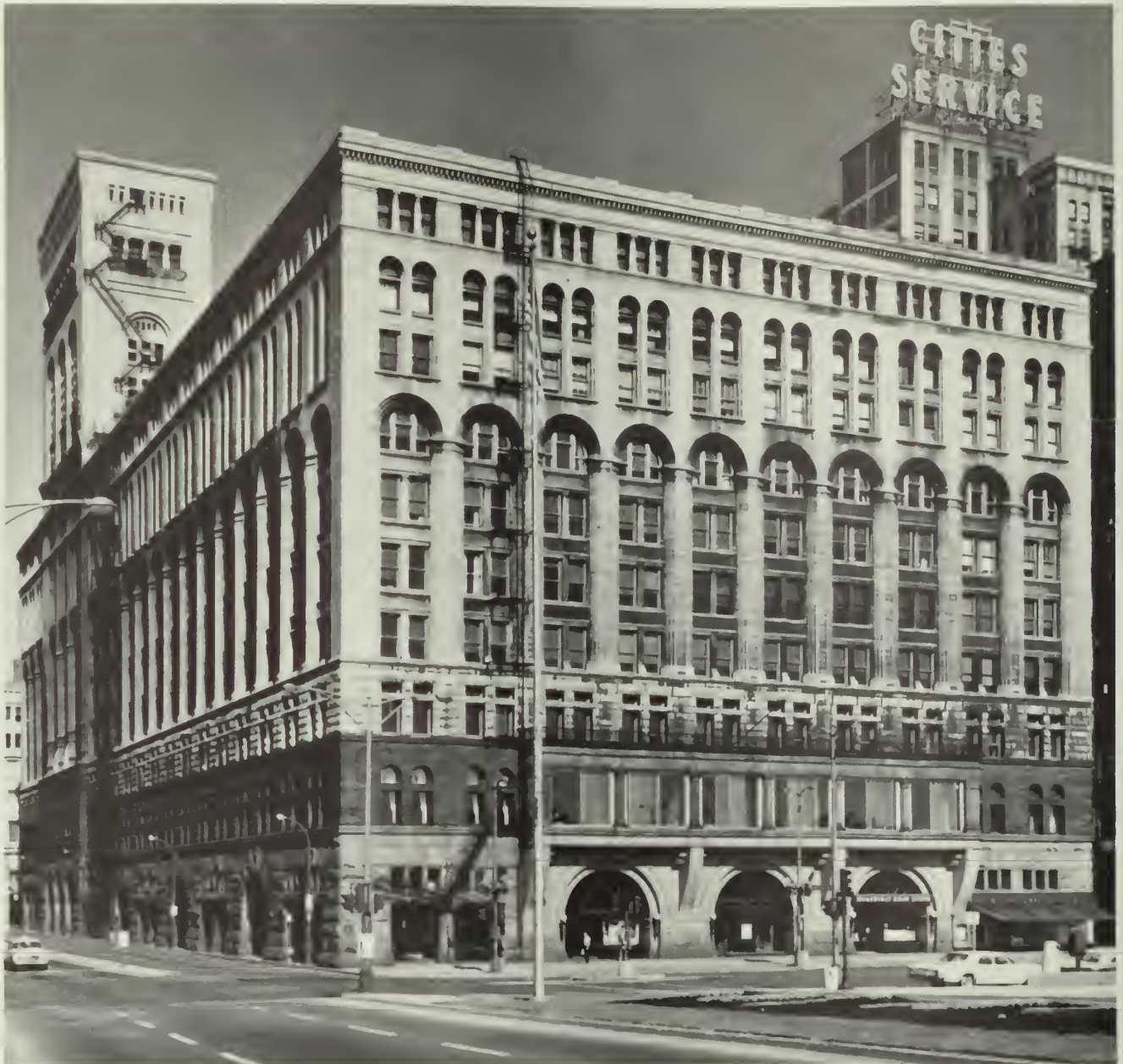
AUDITORIUM BUILDING, 1887-89. ADLER AND SULLIVAN, architects. Photograph by Cervin Robinson for Historic American Buildings Survey.
