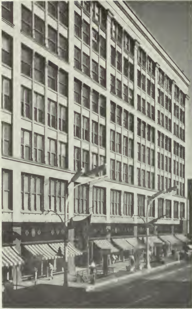
LEITER II BUILDING, 1889-91. WILLIAM LE BARON JENNEY, architect. Photograph by Cervin Robinson for Historic American Buildings Survey.
