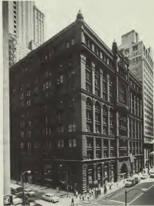
THE ROOKERY, 1885-86. BURNHAM AND ROOT, architects. Photograph by Hedrich-Blessing.
