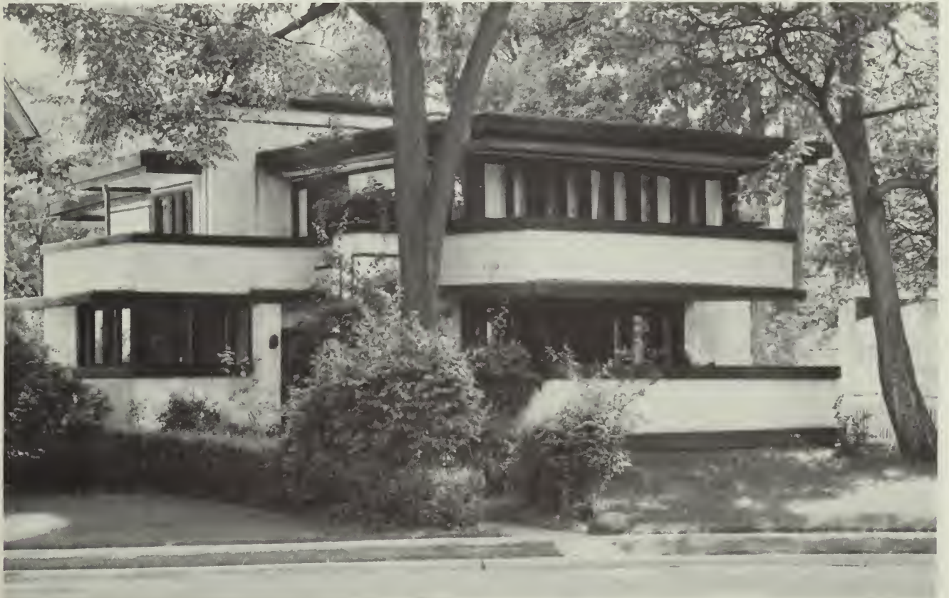
MRS. GALE HOUSE, 1909. FRANK LLOYD WRIGHT, architect. Photograph by Richard A. Miller for Landmarks Preservation Council, Chicago.
