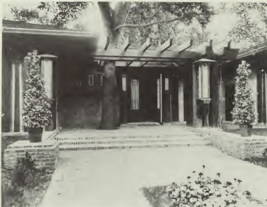
KENILWORTH CLUB, 1906. GEORGE W. MAHER, architect. Photograph for Historic American Buildings Survey.
