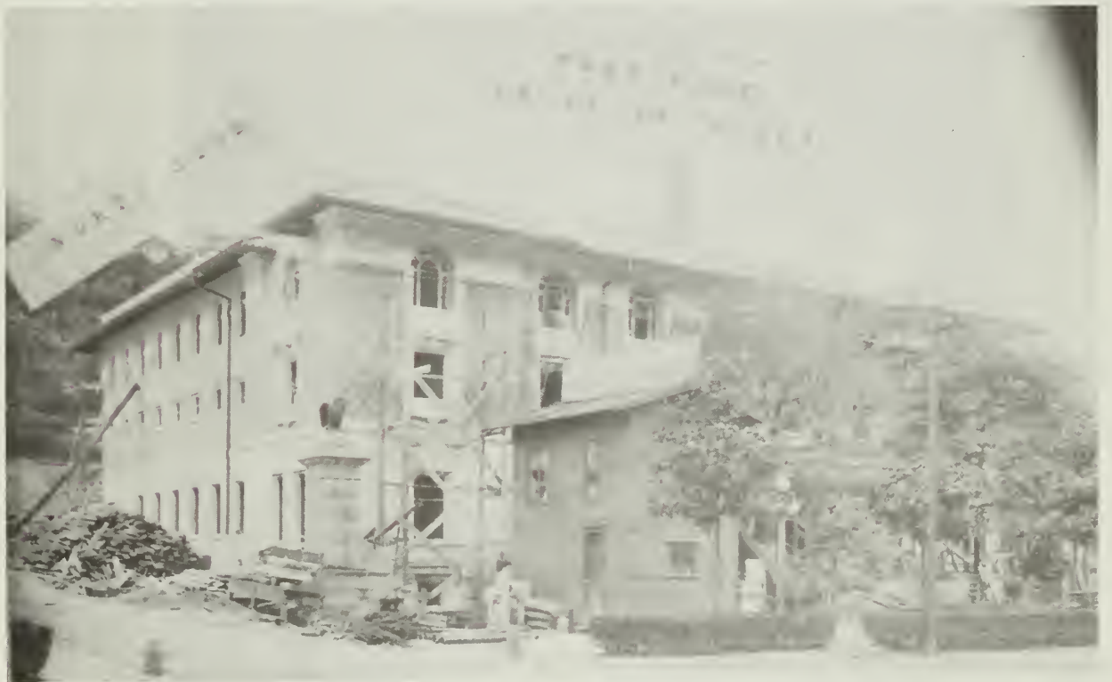
Figure 14. The Fordyce under Construction, 1914-1915 (Source: National Archives, Natural Resources Division, RG 79)
