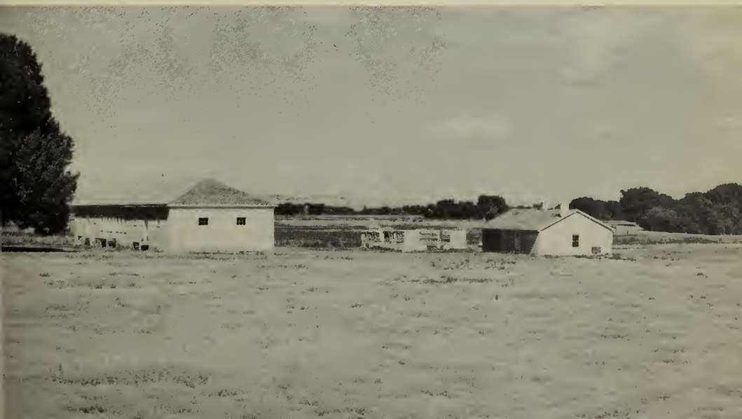
The restored commissary-storehouse, the old bakery, and ruined new bakery, 1954.
