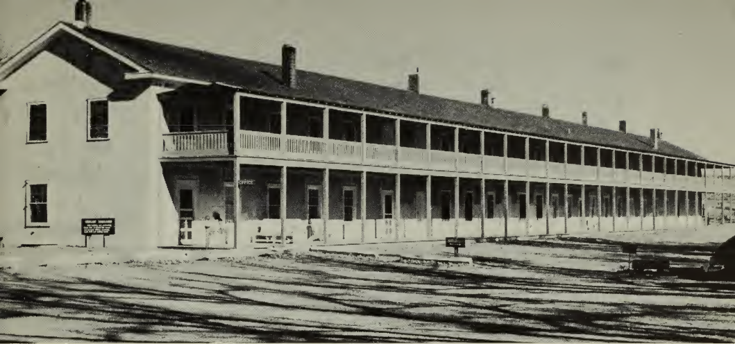
The cavalry barracks, 1954, partially restored.
