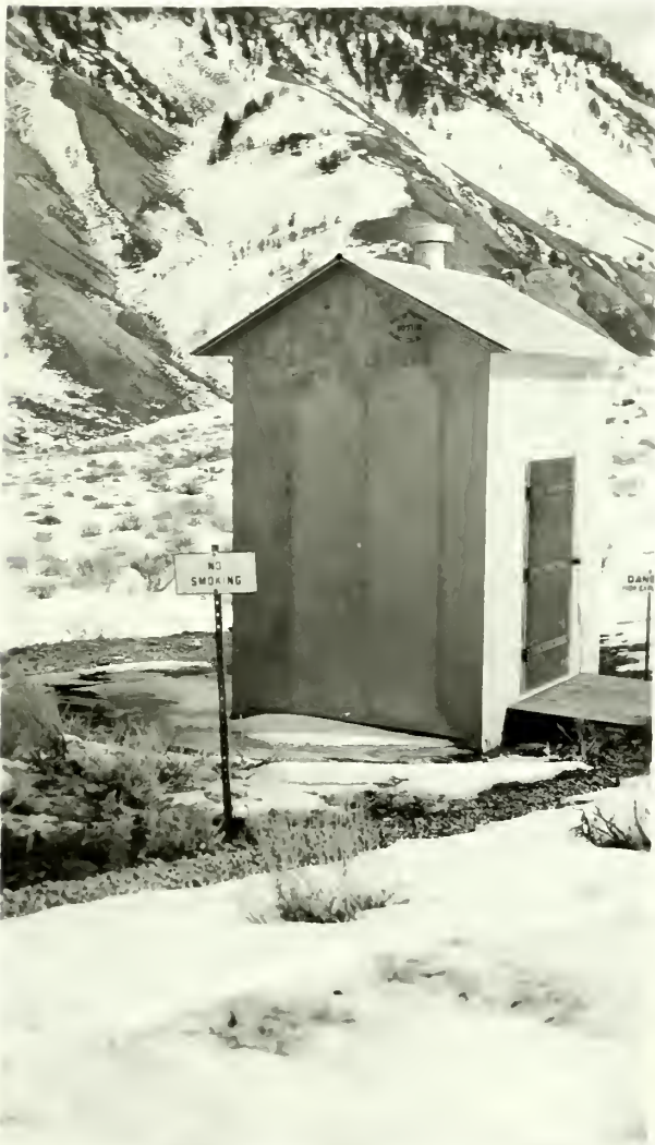
Storage Building for dynamite caps, CCC Job No. 243 at start and completion of work. Tenth Period.
