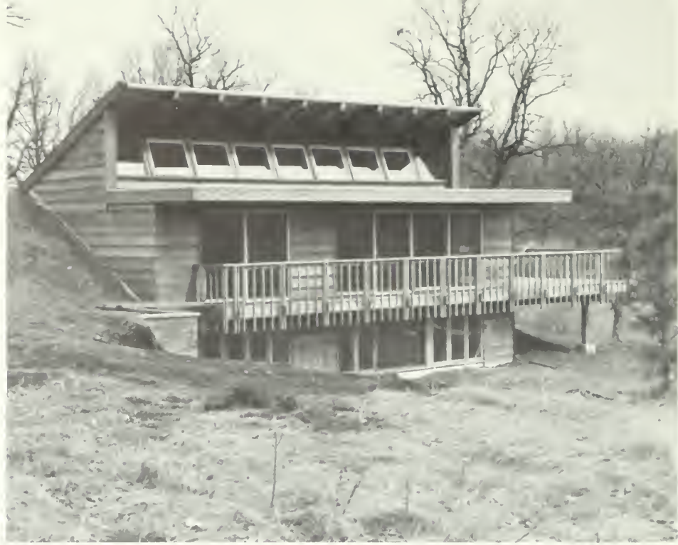
Passive solar and earth shelter design of this employee house at St. Croix Wild River State Park has brought considerable energy savings, while serving as a model for new energy conserving building technology. Photo: Minnesota Department of Natural Resources
